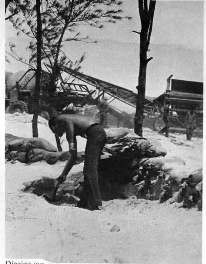
Digging out from bunkers at NSAD Dong Ha Cua Viet
