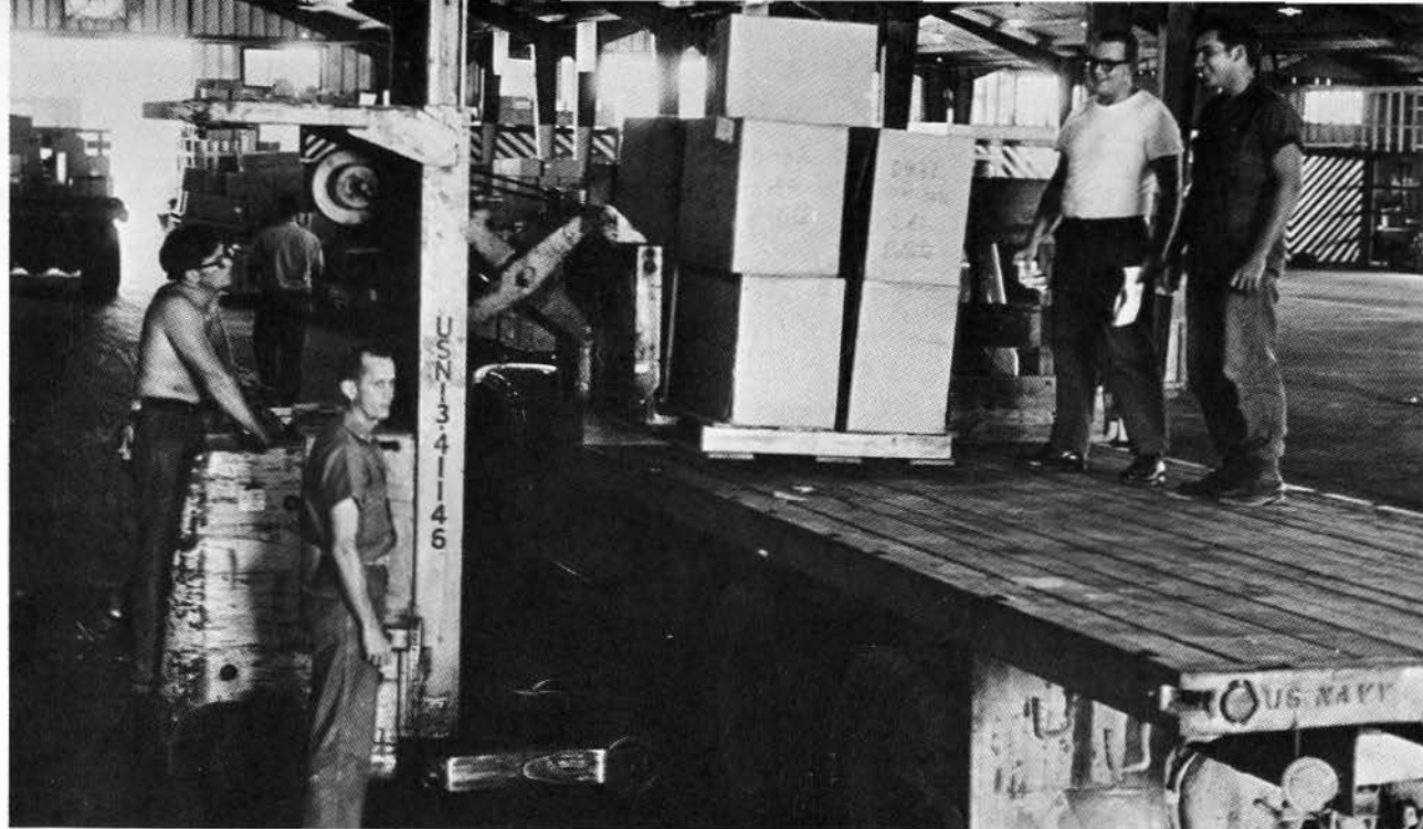
▲ Heavy equipment like this makes the job easier
