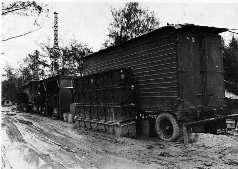
Communications and Power Center
