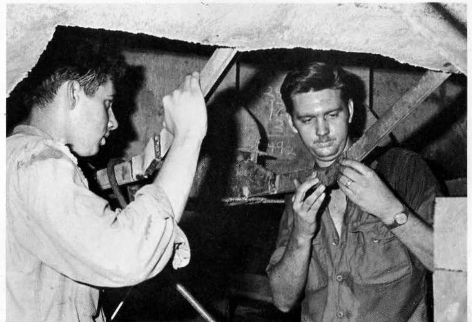
M.L. Sullivan, SFM3, and L.L. Holter, SFM3, weld in bracing for LCU hull.
