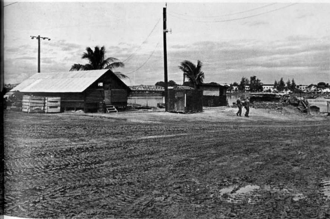
Office at Hue Ramp
