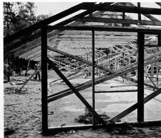
New galley under construction
