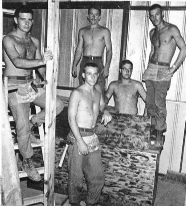
Working on new officer's mess at Chu Lai
