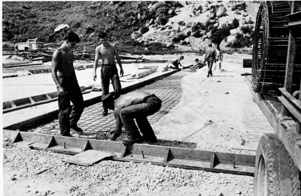
▼ Laying concrete is hot, exhausting work
