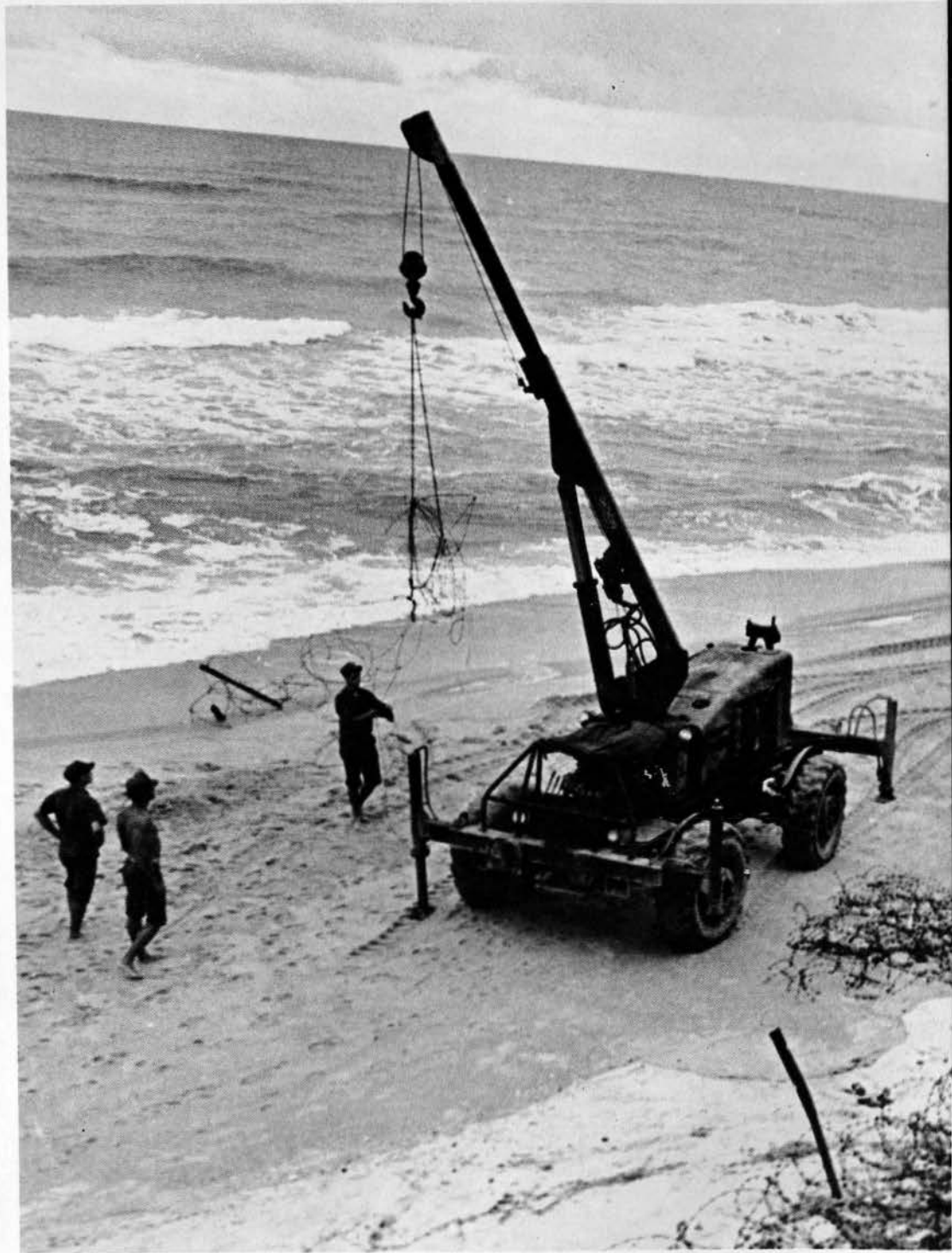
Men working on perimeter
