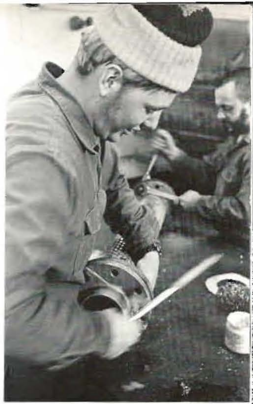
LOOSENING A FLANGE, Constructionman Jim Sellers removes one end, and Utilitiesman second class Dennis Larochelle the other, while (BELOW) Utilitiesman first class Jackie Williams cuts pipe.
