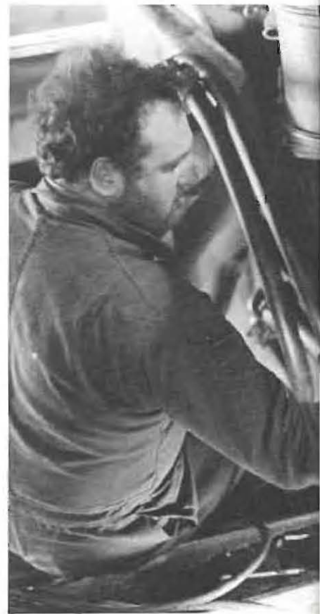
REINSTALLING A D-8 STARTER after repair, New Zealander Alastair Brass (BELOW) tightens bolts to secure it to the engine.
