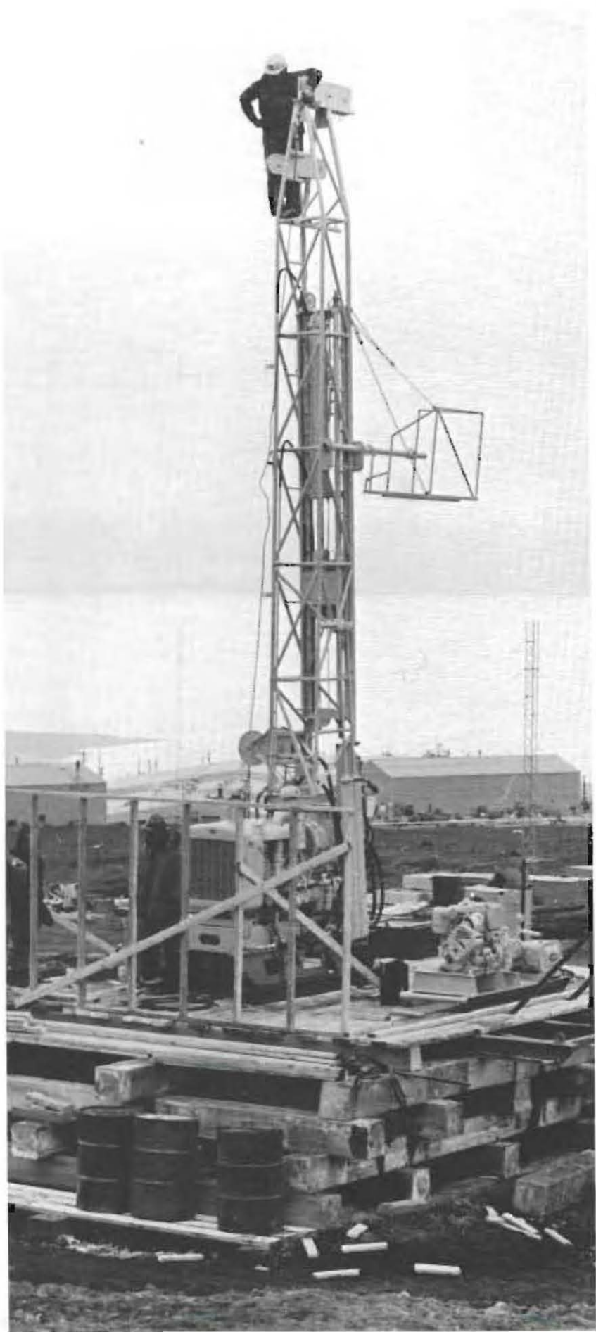
TOWERING ABOVE MCMURDO, the drill rig (RIGHT) is being used to extract cores from beneath the surface of Ross Island.
