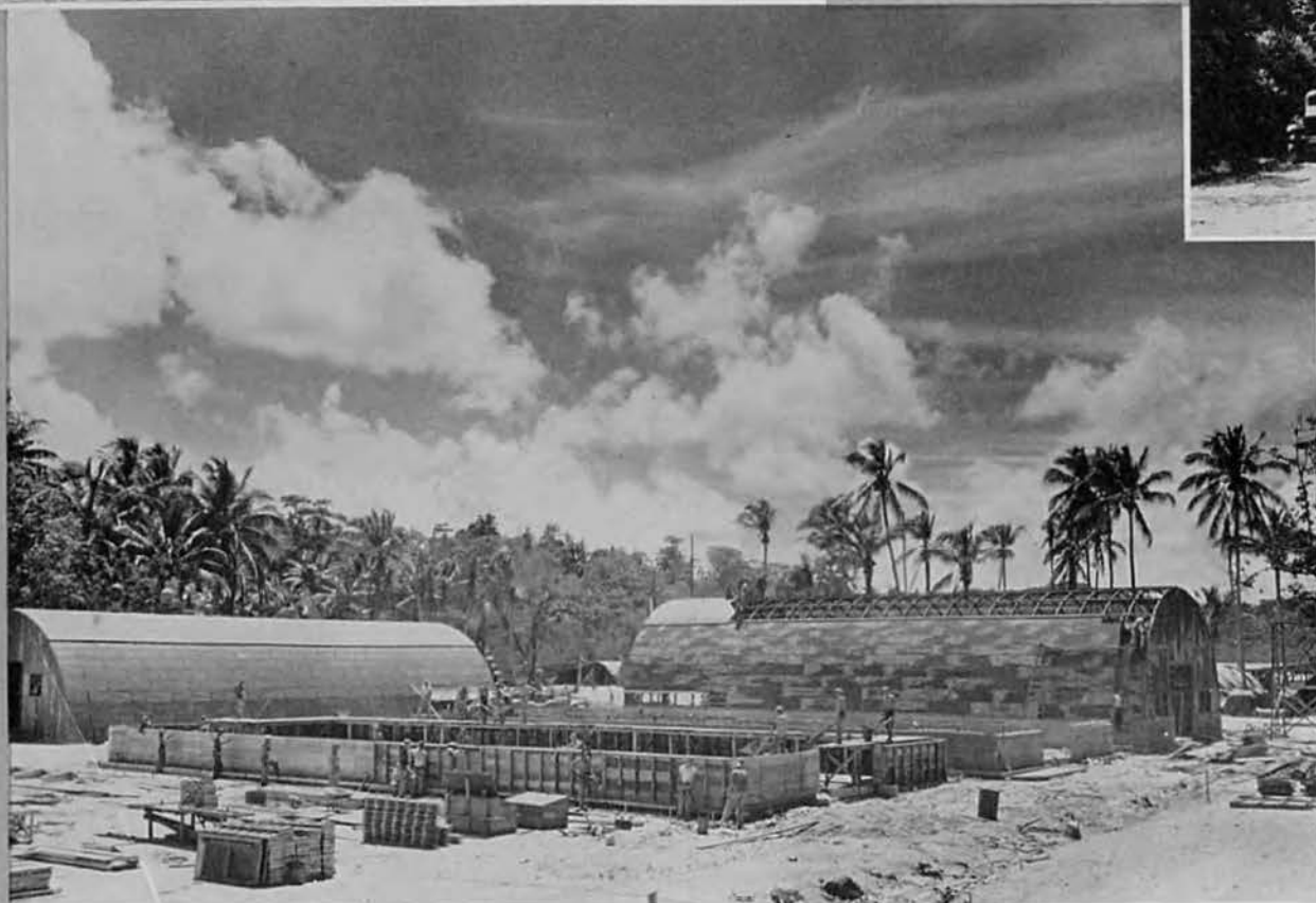
Upper left: 1008 Maintenance Camp at Carter City, to house rear echelon. Upper right: Original Maintenance Shop at Carter City. Lower pictures: 40x100 quonset warehouses, with 4' high concrete foundations under construction for radar and radio lab at Carter City.
