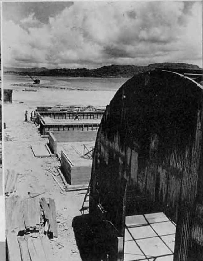
Upper left: 1008 Maintenance Camp at Carter City, to house rear echelon. Upper right: Original Maintenance Shop at Carter City. Lower pictures: 40x100 quonset warehouses, with 4' high concrete foundations under construction for radar and radio lab at Carter City.
