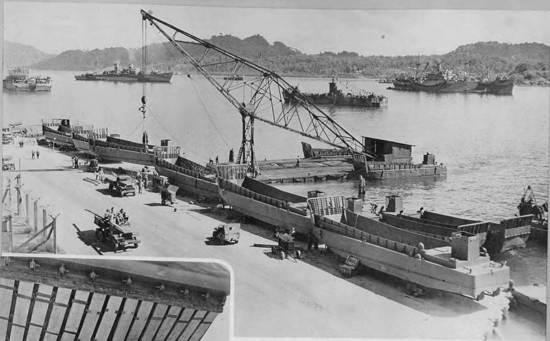
The 1008 shipyard where progressive in-line construction was carried on. The 75 ton crane in the upper picture is picking up a completed LCM preparing to put it back in the water. 65 bottoms were fabricated and attached to LCM's in thirteen days. Heretofore, coral reefs destroyed the bottoms of LCM's when making an invasion, but with wooden skids like these it was possible to hurtle the reefs without damage to the hull. This work was carried on during the staging period before the invasion of Okinawa. Stateside lumber was first used for this but it frequently cracked due to the bends required. It was found that native lumber cut the day prior to use would conform to the contours of the LCM best. The picture at lower left shows the completed product.
