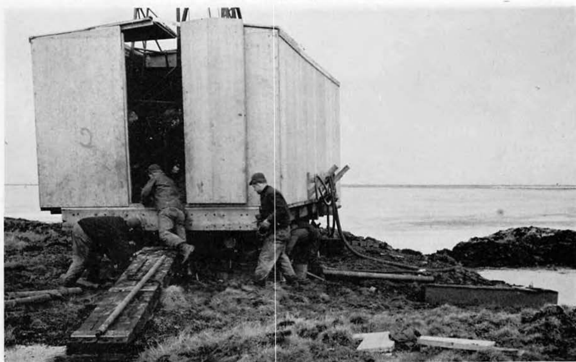
Core drilling at the Simpson Camp.
