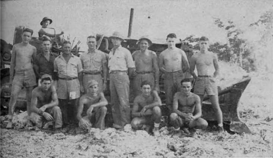
... GRADING AND CLEARING
