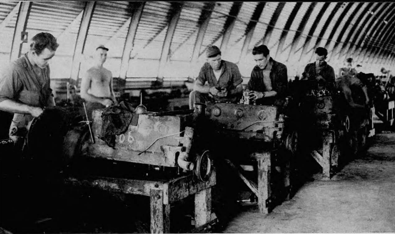
Assembly Line Repairs!
