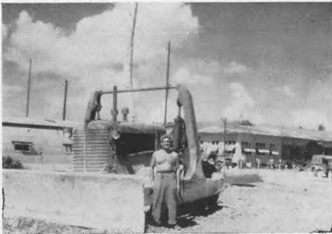
Sinico and his bulldozer.
