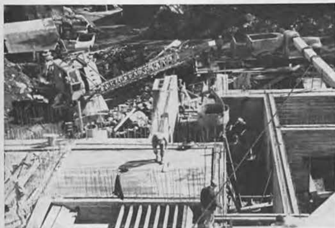
Top: Makhnati construction. Bottom: Bay City at work.
