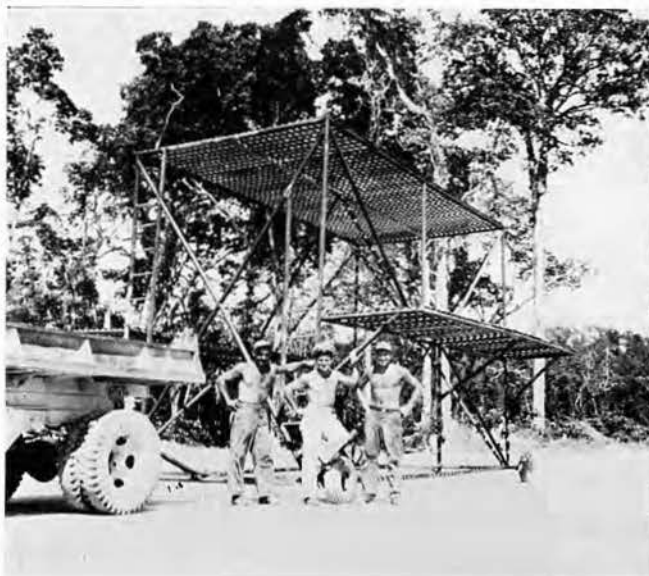
Portable Scaffold for Dismantling Quonsets; Wait's Patent.
