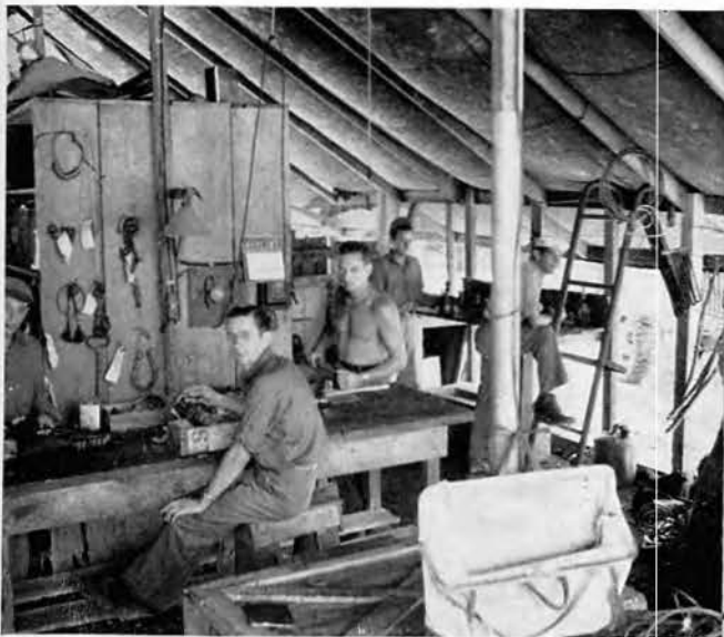
The electric and refrigeration repair shop on Munda . . . maintaining New Georgia's extensive electrical system was their job . . .
