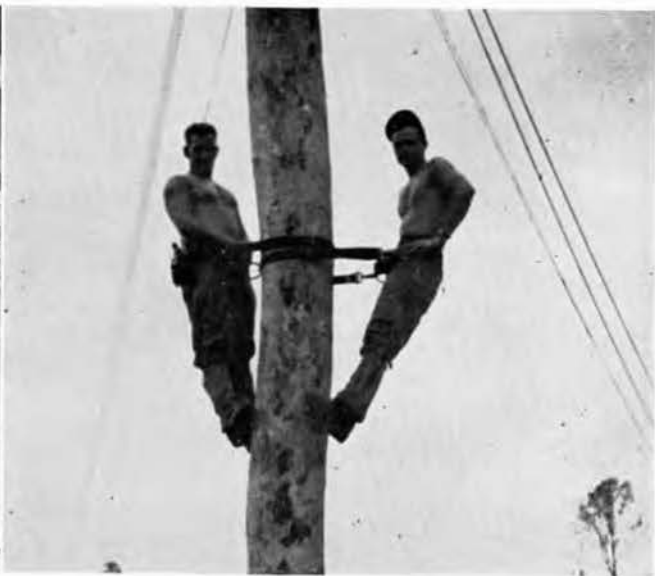
. . . and the communications electricians kept up the island's telephone system . . .
