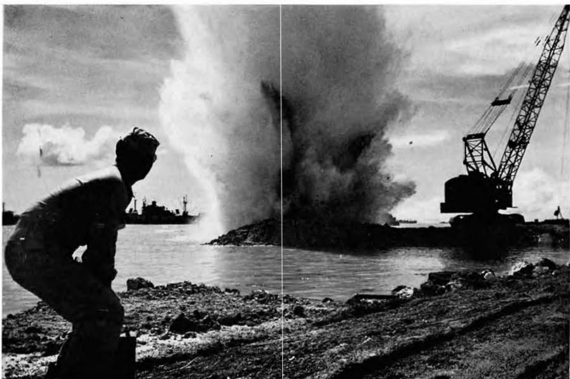
Keeping Seadler Harbor's dock approaches deepened was our continuous job.
