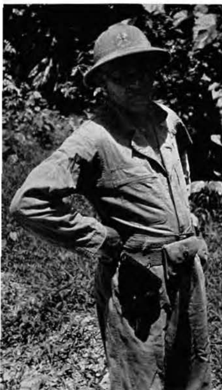
Warrant Officer Dod ruled the construction end with an iron hand . . .
