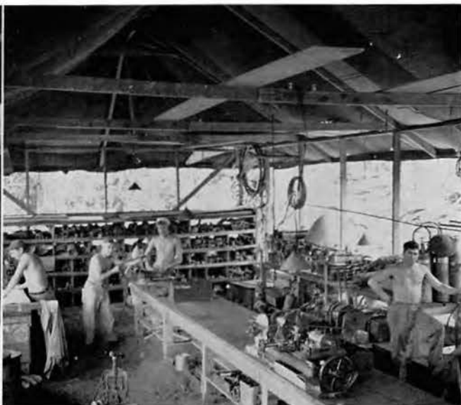
Plumbing and sheetmetal shop at Munda.
