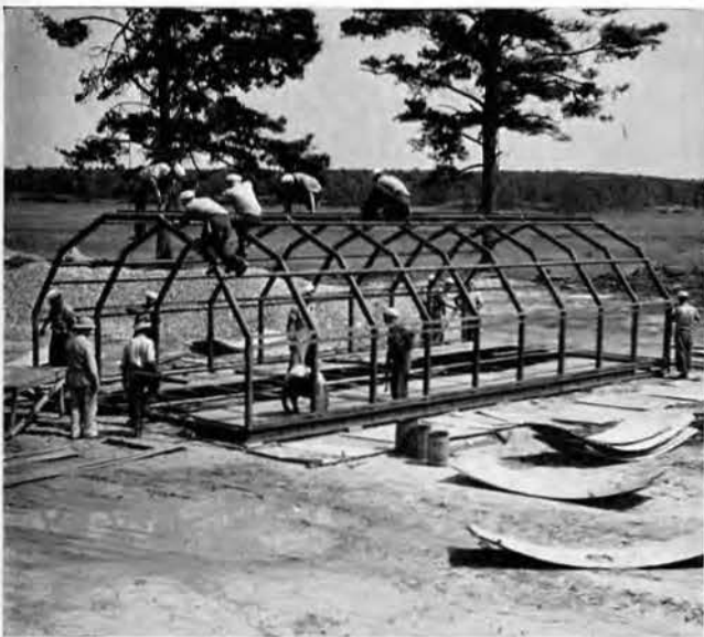
Learning to assemble a 20' x 48' Quonset Hut in 120 man hours so bases could spring up quickly in the Pacific.
