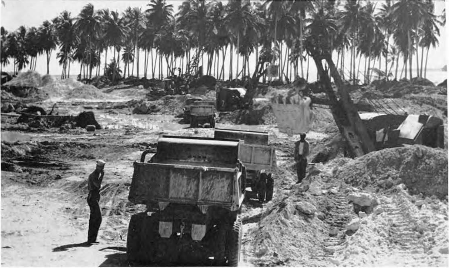
This is the Bougainville airstrip, in preparation.
