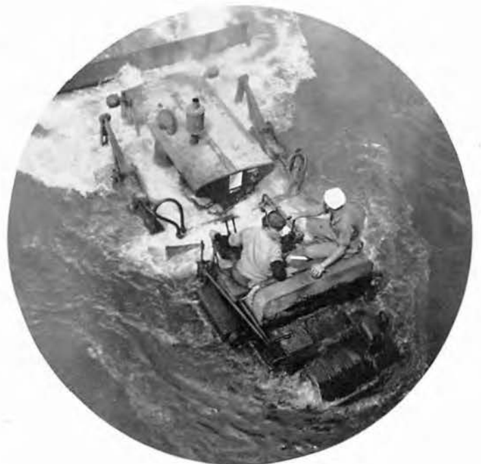
A Seabee tractor backs from shore to ramp over a submerged steel mat. The shot was taken at Port Hueneme, California.
