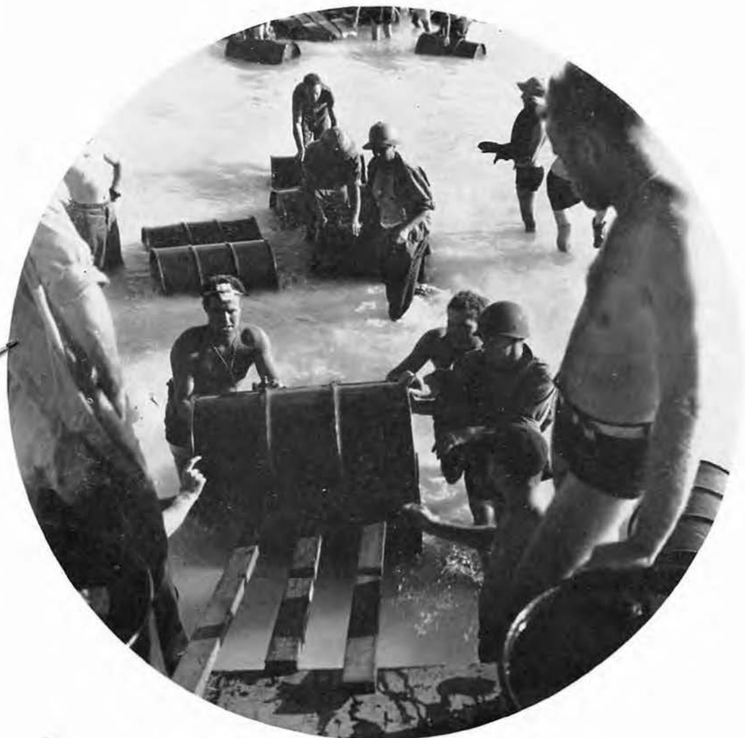
Seabees roll in the barrels. The drums are filled with aviation gasoline.
