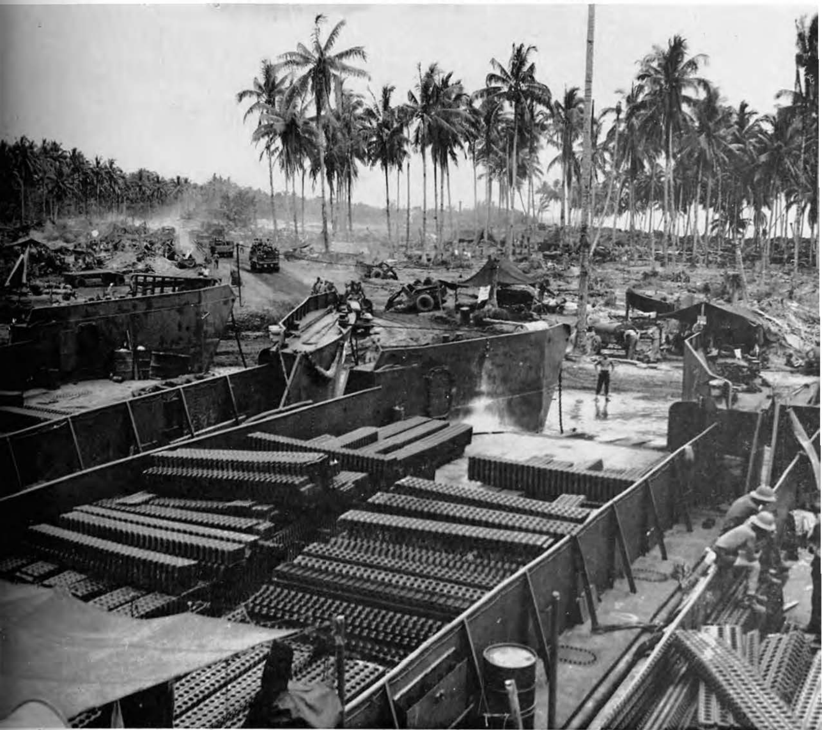
Seabees unload their supplies and equipment, to clear the jungles, roll the airport and put the metal strips together to form an airfield. The scene is in the Bougainville jungles.
