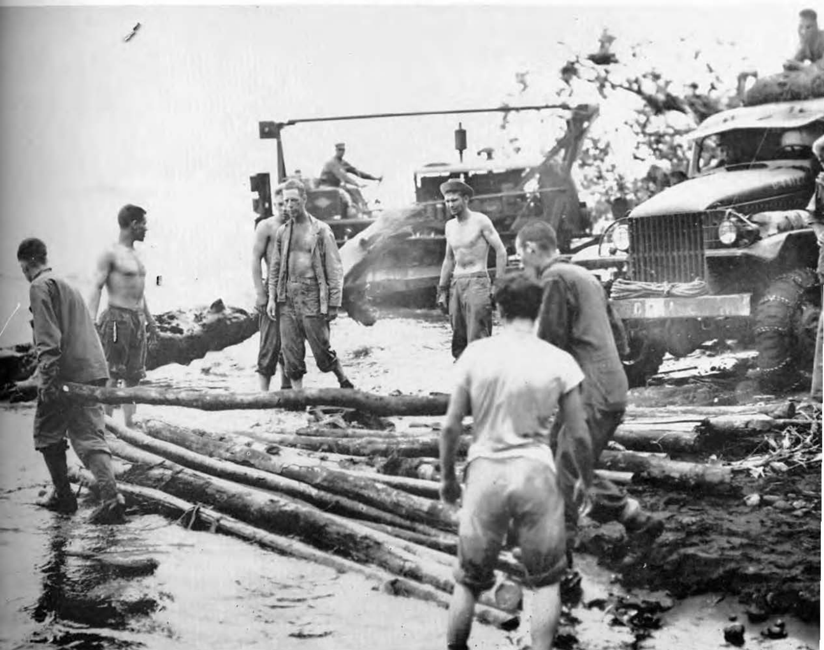
Trees and logs are put in place by Marines and Seabees for a bridge across a jungle stream on New Britain Island.
