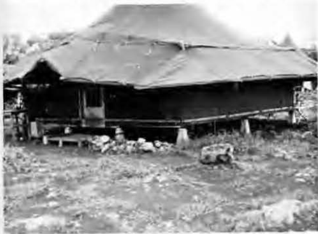
38th Battalion prefabricated 16 x16 foot squad tent. Photo, Merle C. Duncan.
