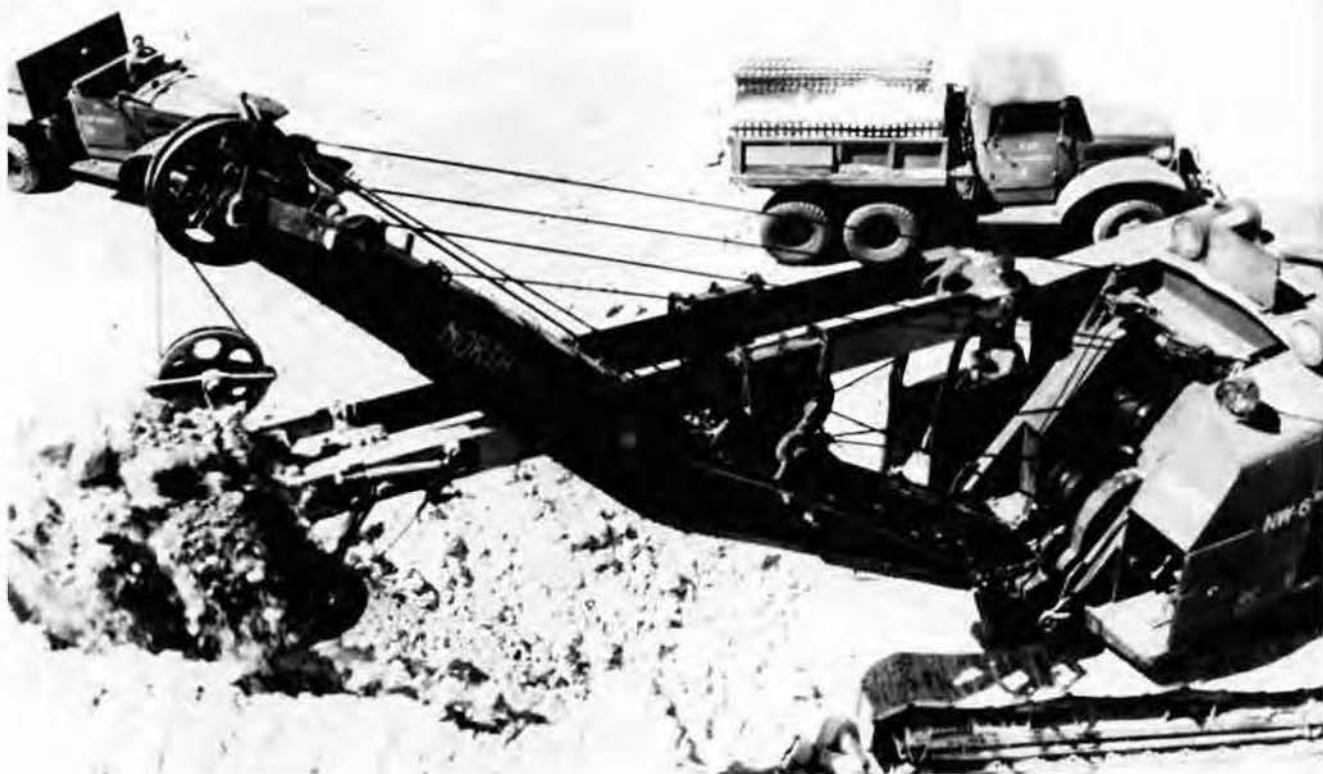
Power shovel loads dump truck. Photo, W. S. Eoff.
