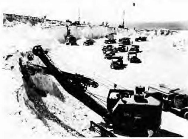
Power shovel scoops coral for loading into waiting dump trucks. The trucks shuttled to and from the construction sites, providing the needed fill material.
