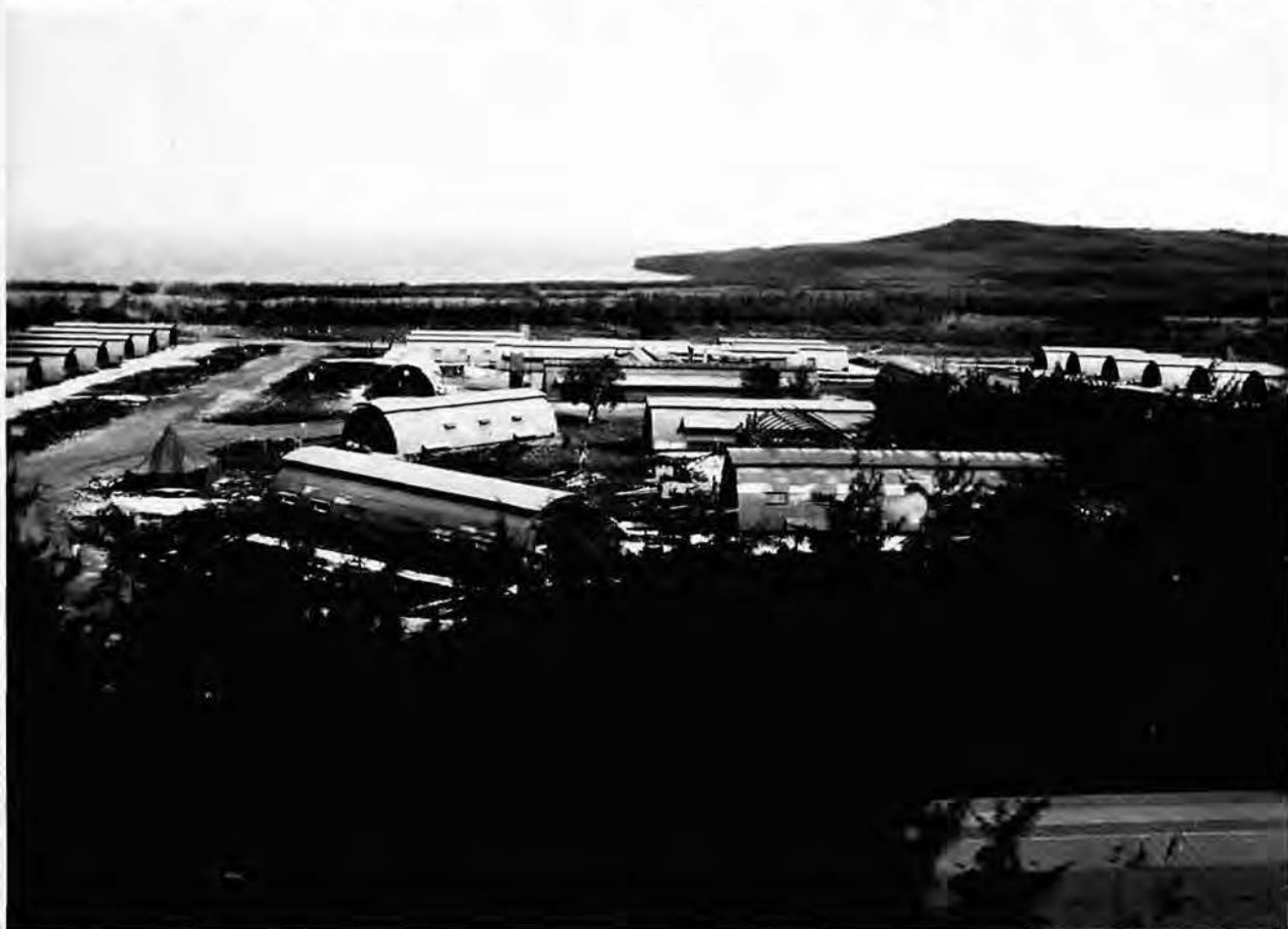
135th quonset hut camp. Photo, George W. Larson.
