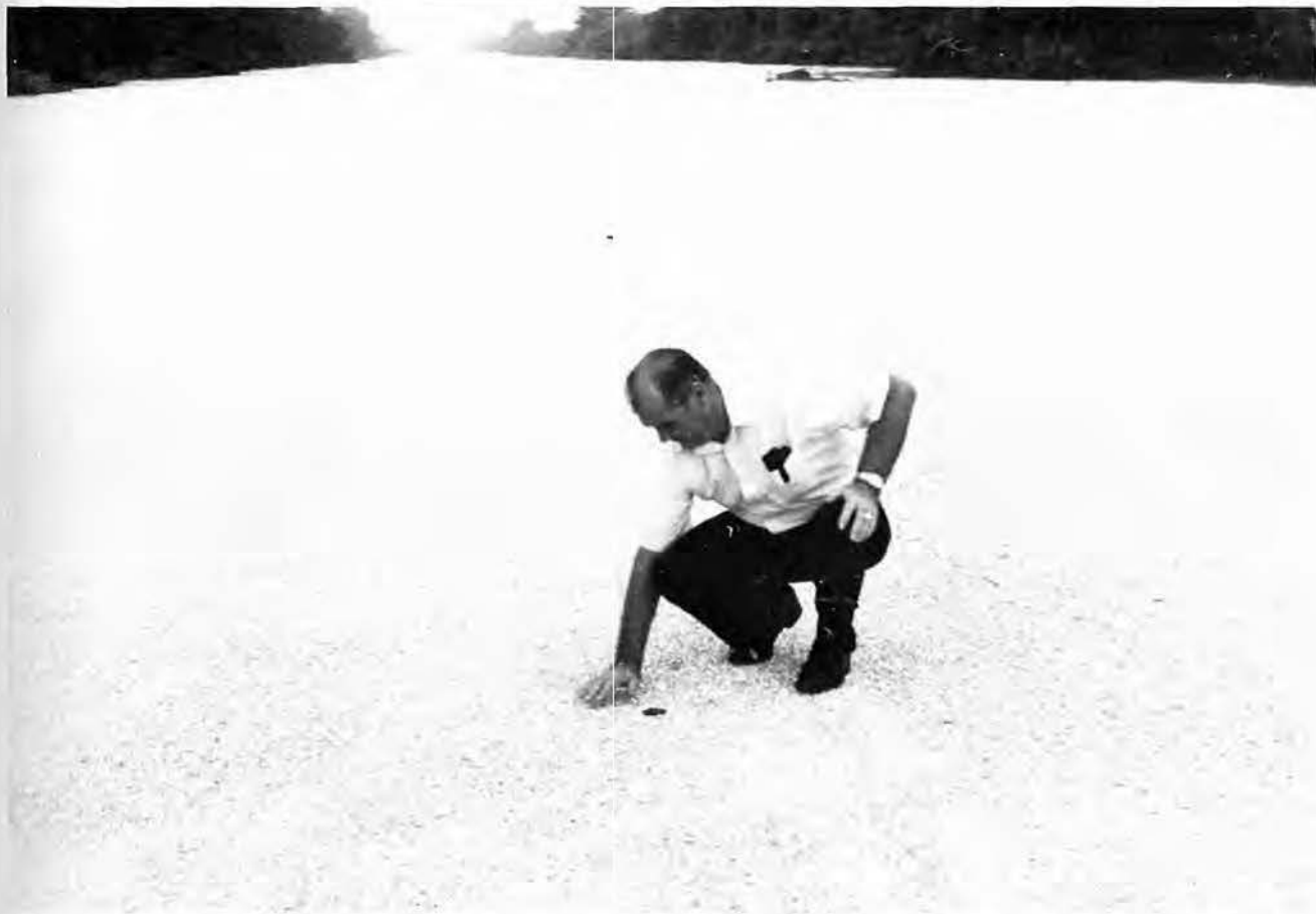
The coral surface on North Field, still exhibits a tight surface that can be used by the most modern aircraft in the U. S. inventory. Photo, George A. Larson.
