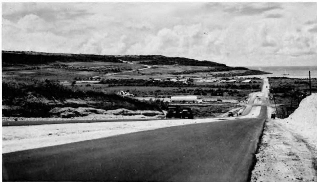
Main haul road. Photo John H. Vandervort.
