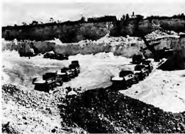
Power shovel scoops coral for loading into waiting dump trucks. The trucks shuttled to and from the construction sites, providing the needed fill material.
