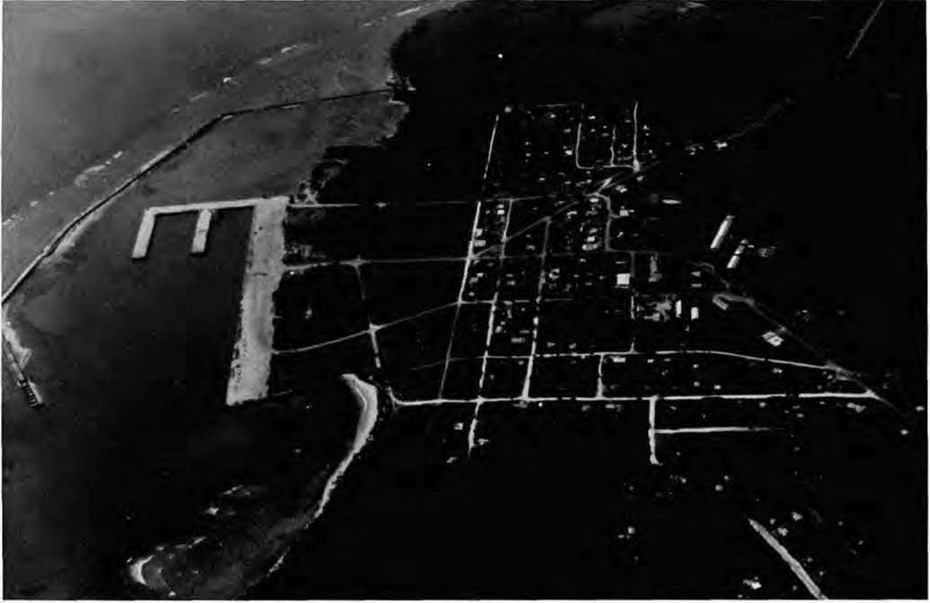
Artificial breakwater surrounds the U-shaped pier complex, built at south end of Tinian. Up to eight Liberty ships could unload at the same time. Photo taken in 1981, shows durability of Seabee construction. Photo, George A. Larson.
