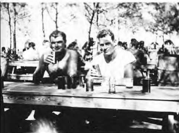
As construction work continued, tables were added outside the messtent for meals and breaks. Photo, George W. Larson.
