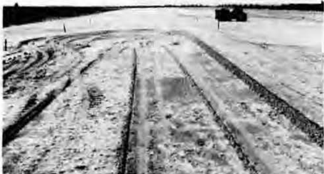
Coral dumped on the runways, bulldozed, graded, rolled with a sheep's foot's spiked rollers. Then as salt water was added to the surface, roller compacted it, providing a hard surface. Photo, W. S. Eoff.
