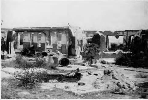
U.S. naval shelling destroyed many island homes. Concrete buildings on the island absorbed heavy gunfire and remained standing. Photo, Elmer F. Goodwin.
