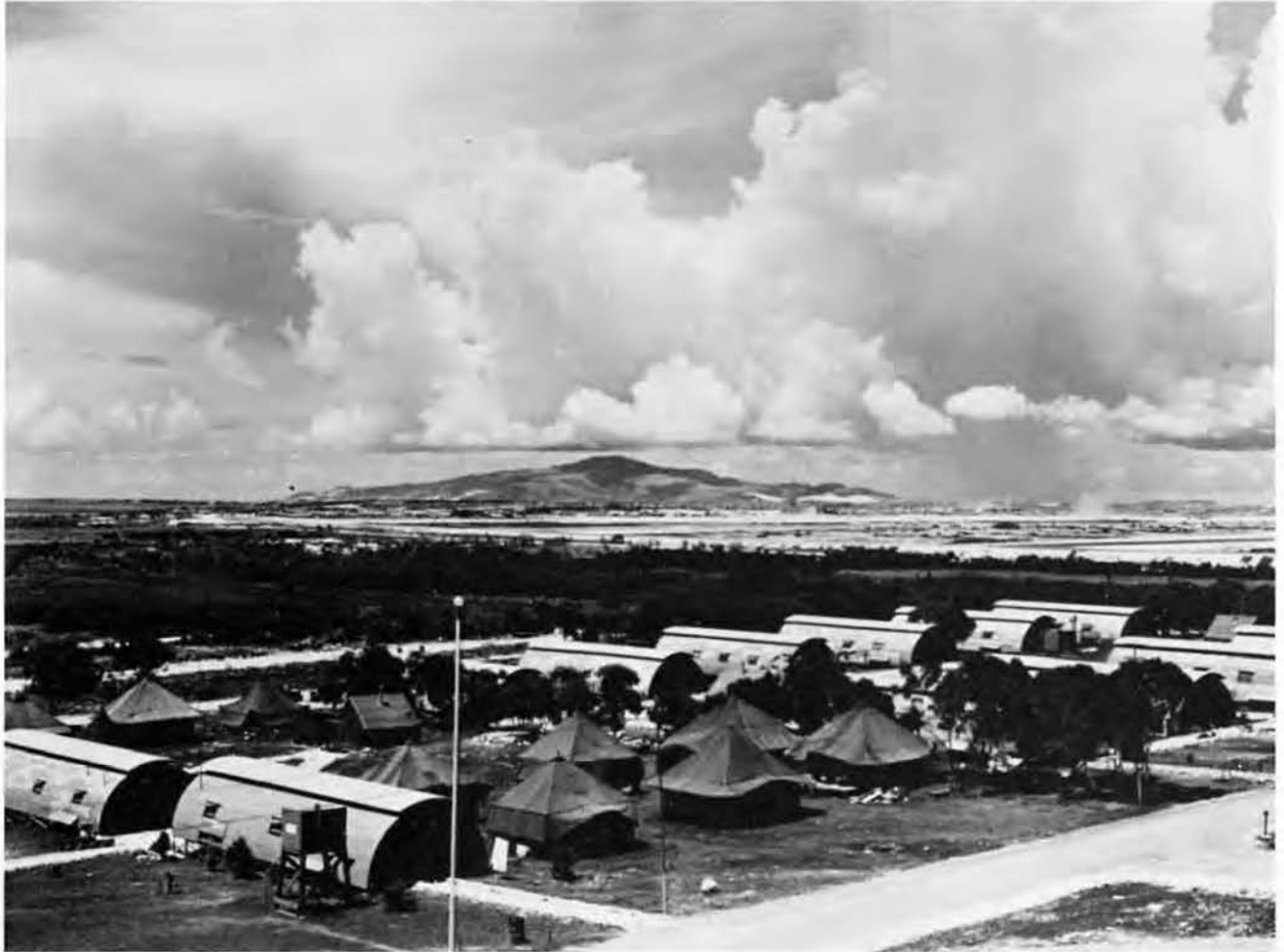
The 509th Composite Group initially lived in tents between quonset huts when first on Tinian. Two weeks later they moved into permanent buildings. Photo, John Vandervort.
