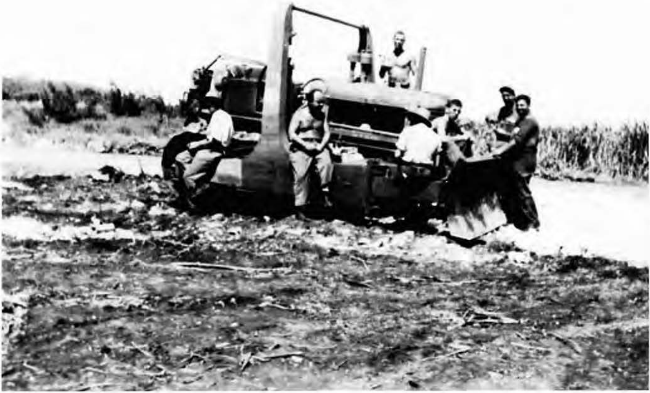
Bulldozer crew starts to clear cane field for camp on Tinian. Photo, Lloyd Ringrose
