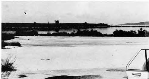
Coral filled, steel plank constructed pier. Photo, George A. Larson.
