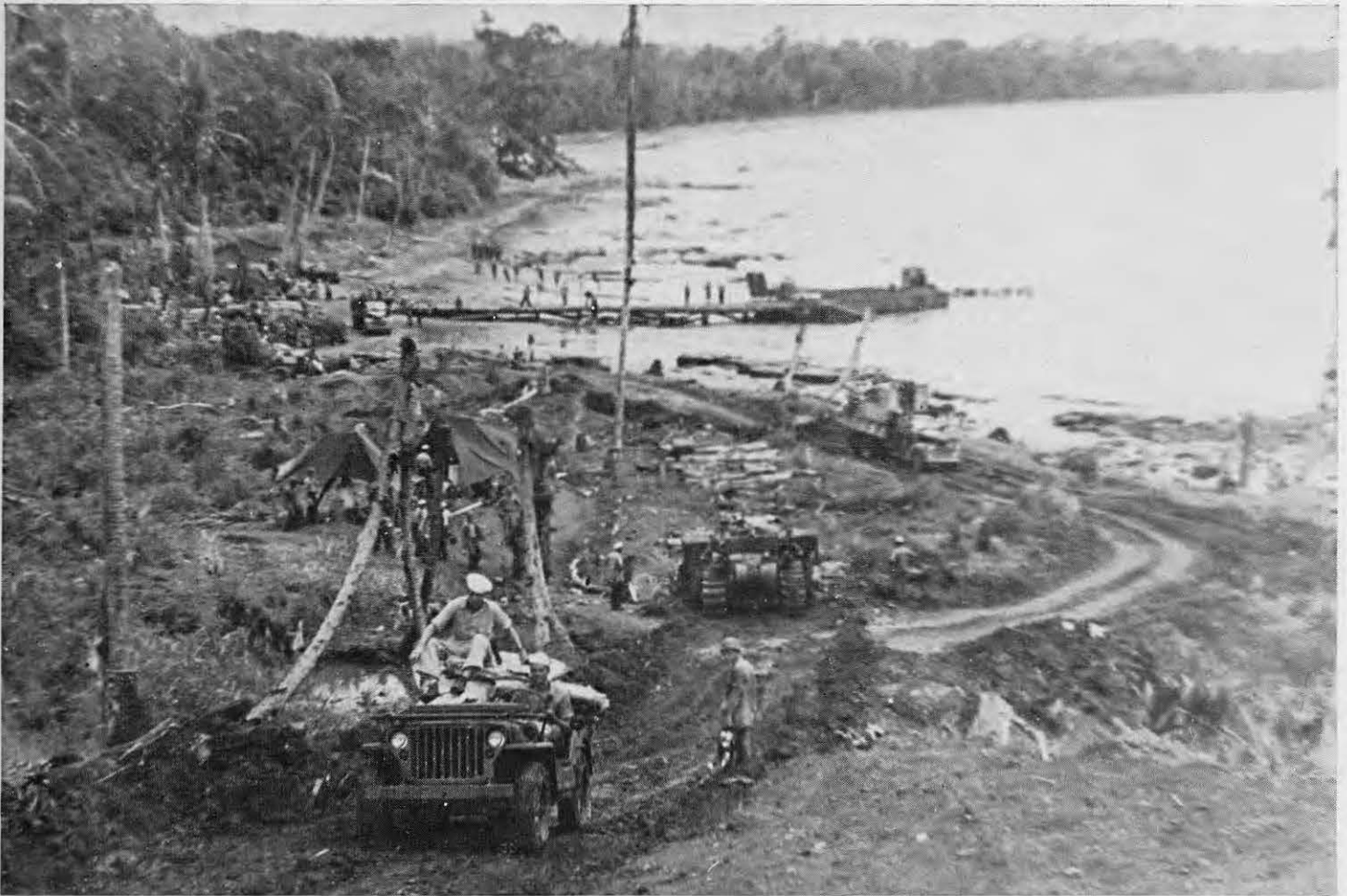
ROAD FROM LANDING—PLUS MUD
