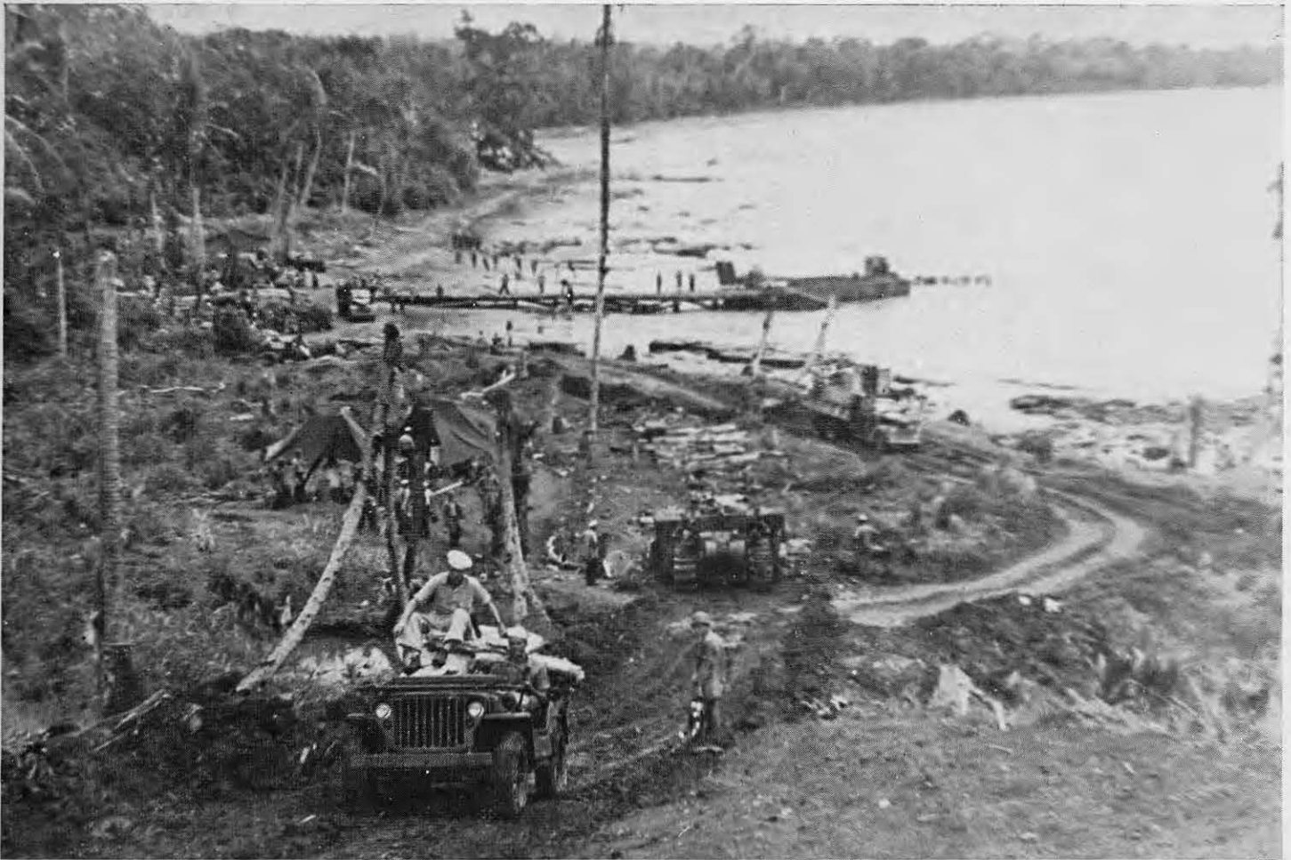
ROAD FROM LANDING—PLUS MUD
