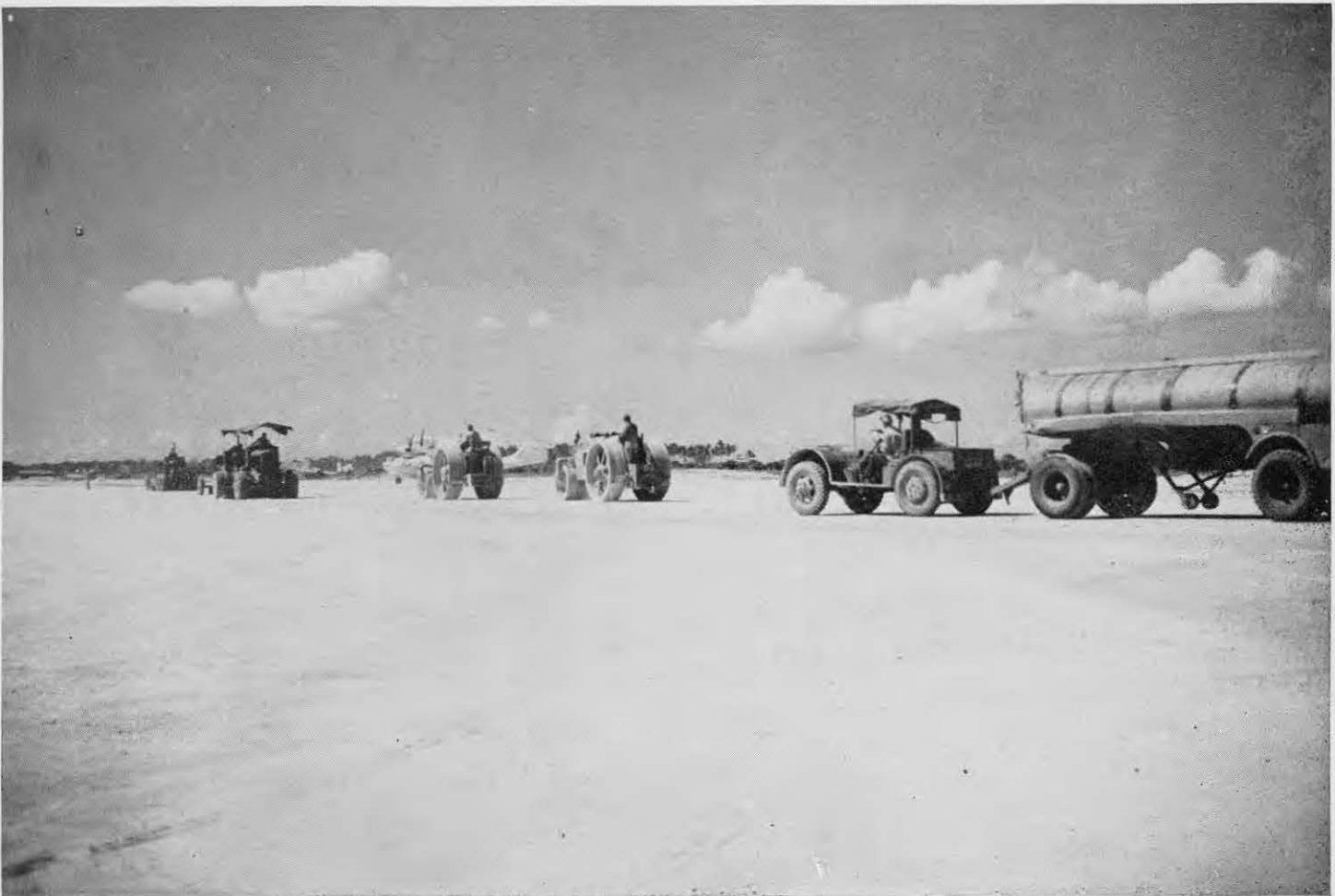
SCRAPING, ROLLING, AND SETTLING THE DUST
