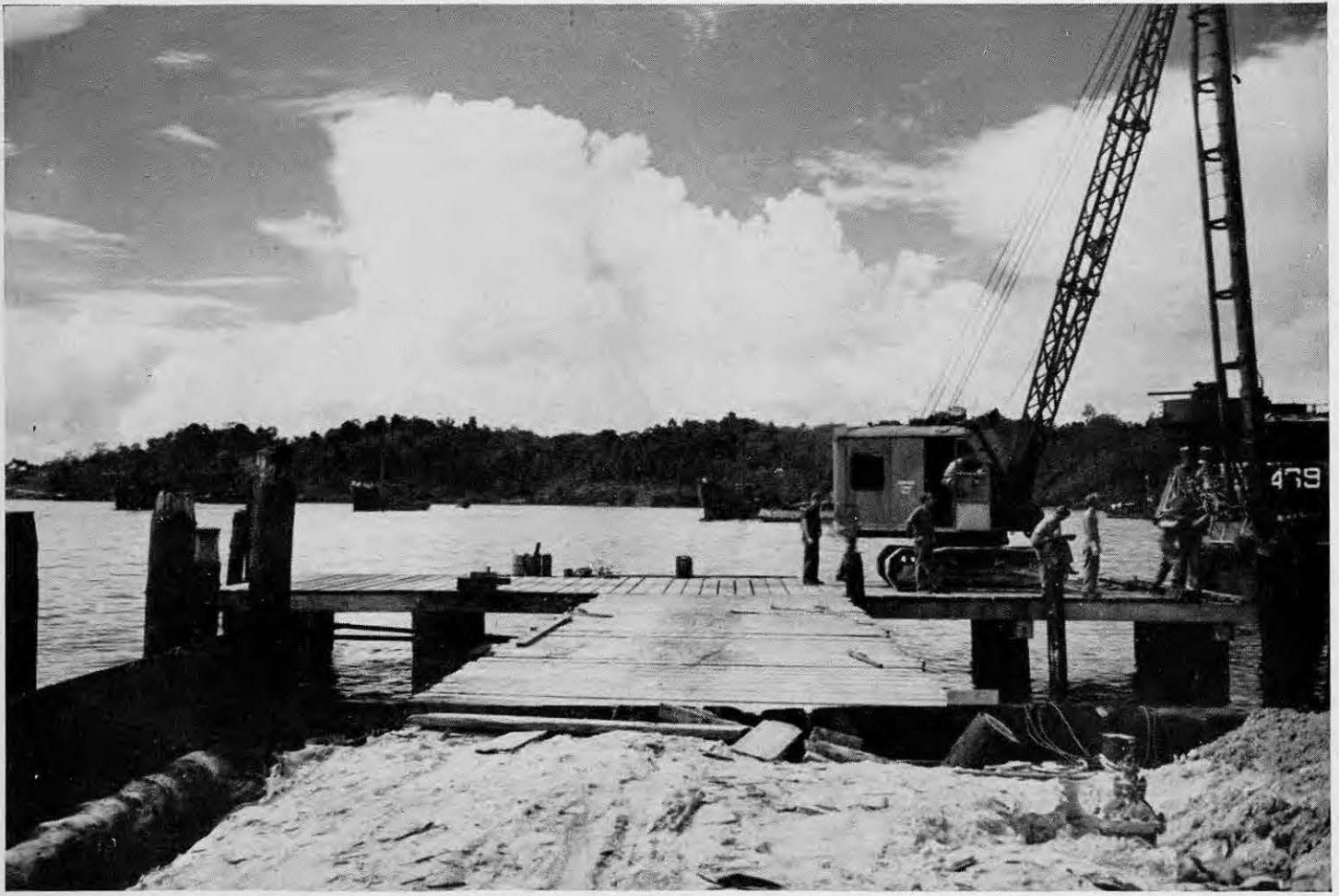
DRIVING PILES FOR SMALL BOAT LANDING
