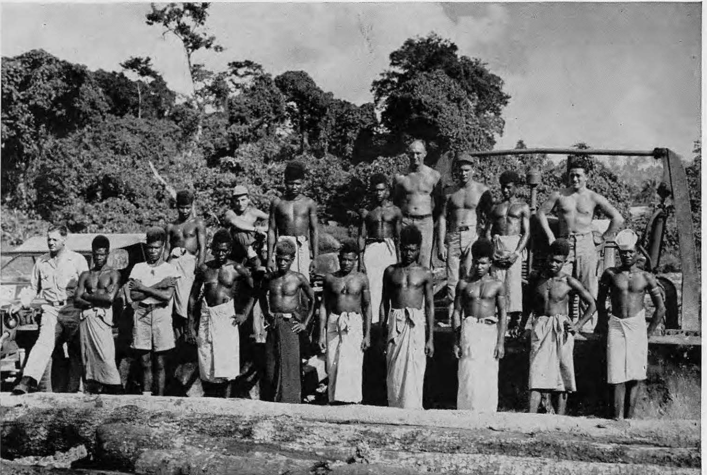
POLE CREW AND AUXILIARY
