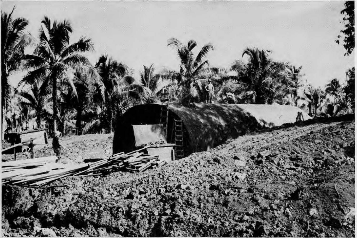
PARTIALLY COMPLETED AMMO DUMPS
