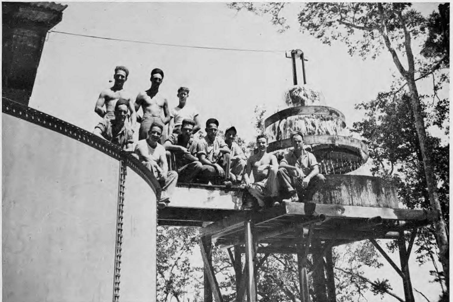
WATER PLANT CREW
