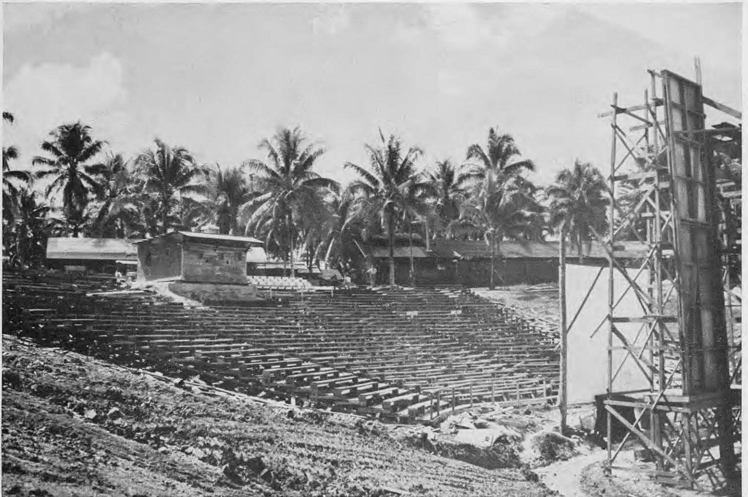
THEATER UNDER CONSTRUCTION
