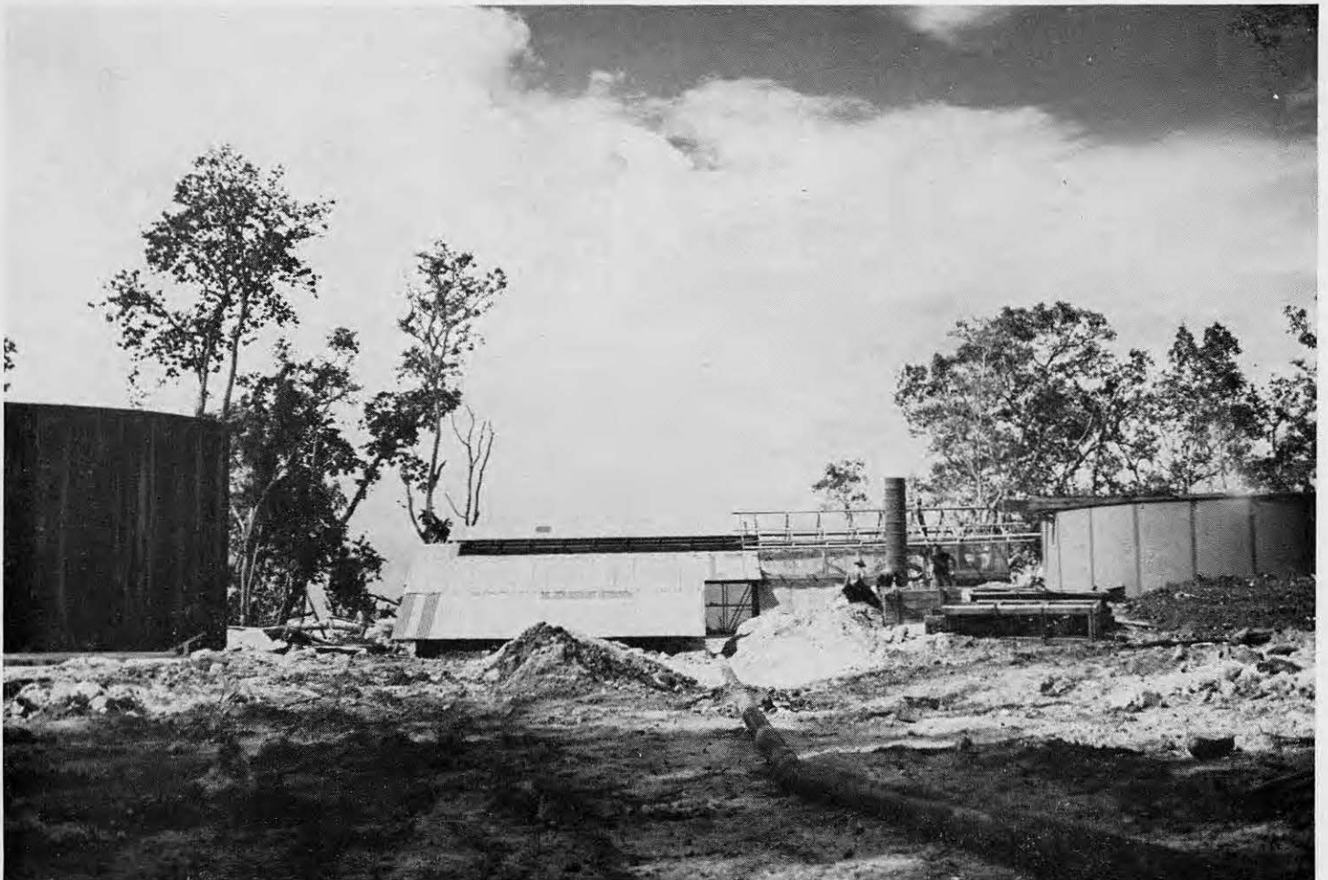
BASE WATER PLANT
