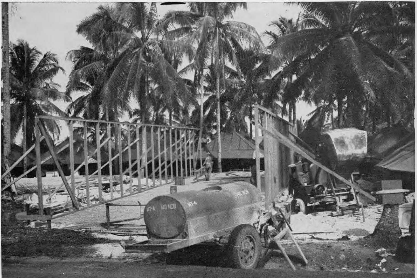
WAREHOUSE UNDER CONSTRUCTION
