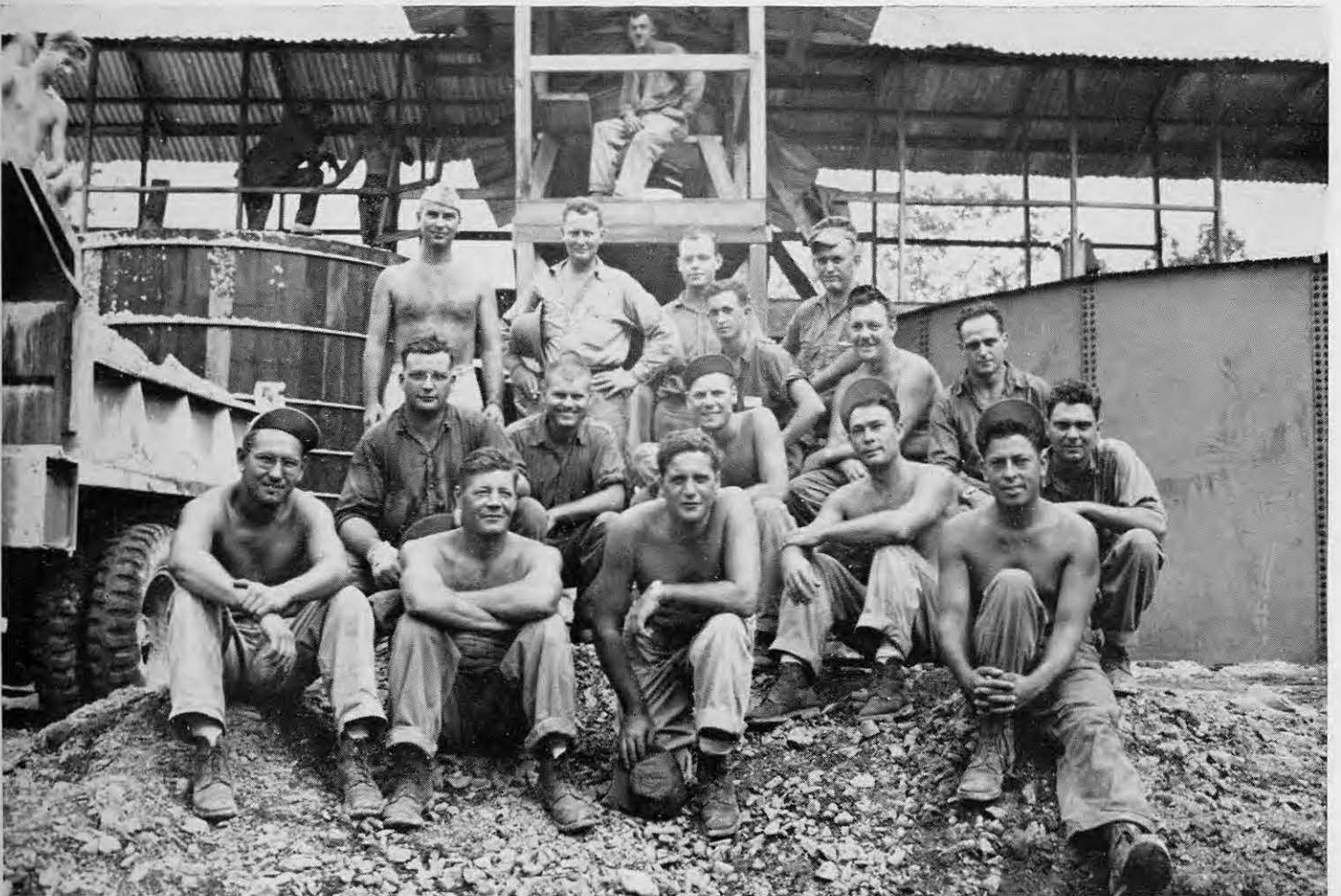
WATER PLANT CONSTRUCTION CREW
