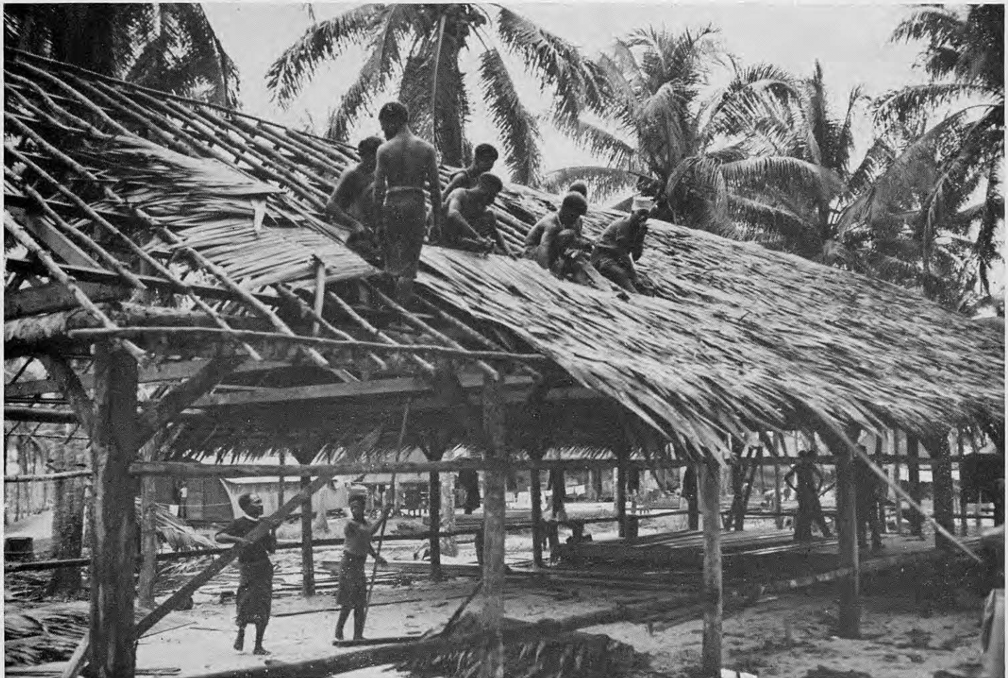
CHAPEL UNDER CONSTRUCTION
