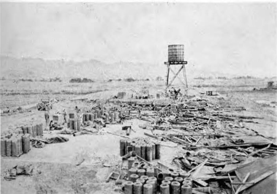
A few pipes and the water tower were all that was left of the 145th's concrete pipe plant after the typhoon.
