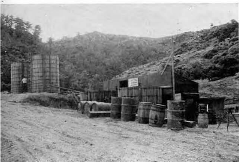
Top photo shows the reservoir to the 145th's new camp on Okinawa. Tanks and treating plant are at the right, and part of the camp can be seen below the hill. The reservoir was created by an earth dam on a small creek that flowed thru camp. Lower pictures show tanks and plant for the water system. Water was pumped from the beach by pipeline, treated and stored, and flowed over the camp thru a gravity system.
