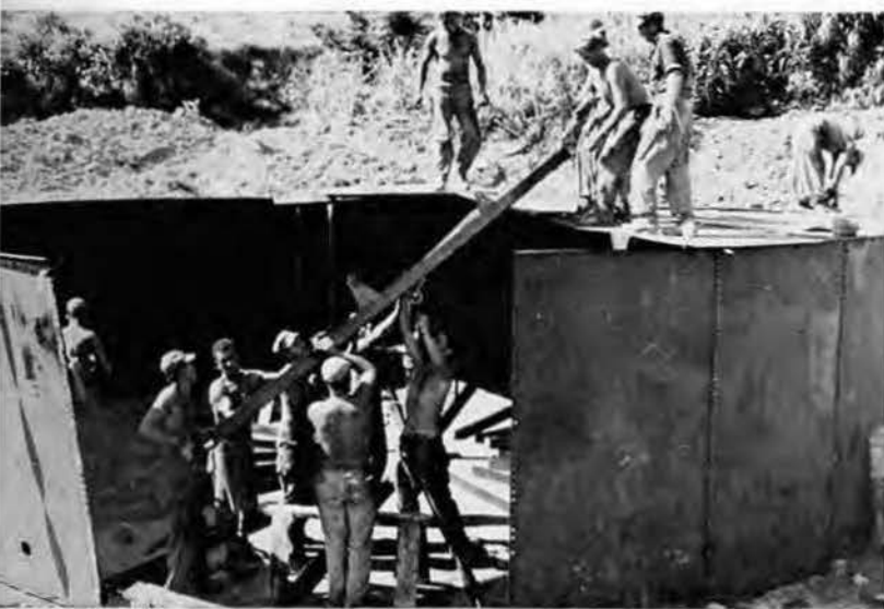
Here are three views of men of the 145th constructing a huge aviation gas tank farm near Yonabaru airfield. The twelve one-thousand barrel steel tanks were located about a mile north of the field and west of Route 13. Besides construction of the tanks, the job included the laying of two miles of four and six inch pipeline. The job was under supervision of Lt. Bentz, Lt. (jg) Redd, and Lt. (jg) Hewett.
