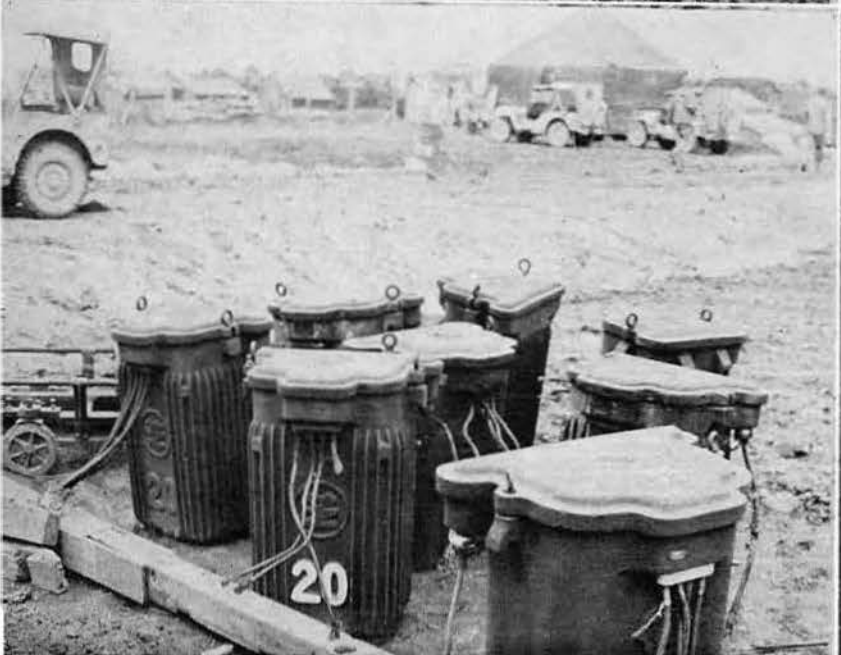
Upper left, Navy Privateers on Yontan airfield; right, C-54's on Kadena airfield; center left, 145th rock crusher, like some pre-historic monster; right, remains of a Jap Saki plant; lower left, Jap transformers salvaged and reconditioned by 145th electrical shop; right, burning Jap plane, shot down at edge of 145th camp.
