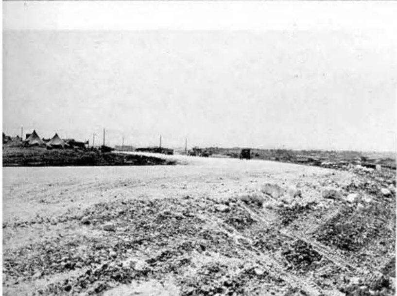
Shown here are three views of Route No. 6 constructed by the 145th from Hiza up the west side of the island along the beaches for about five miles. One of the island's heaviest traveled roads during the Okinawa campaign, this artery was built extra wide and heavily coraled.
