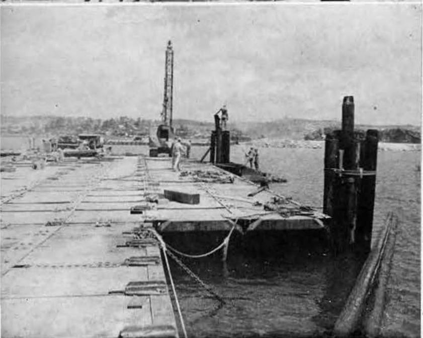
A giant causeway was built on the China Sea near Machinato in July by men of the 145th. It consisted of two earth piers, one 1100 feet long and the other 1400 feet, and both bearing 40-foot roadways. The piers were connected by a pontoon causeway 800 feet long and six pontoons wide. At the end of one pier an LST unloading ramp 60 by 200 feet was constructed. During the project a temporary camp for 400 men was located at the site. The three photos on the left show the pontoon section; upper right and center right show the building of the earth sections; and lower right photo shows the completed dock in operation.
