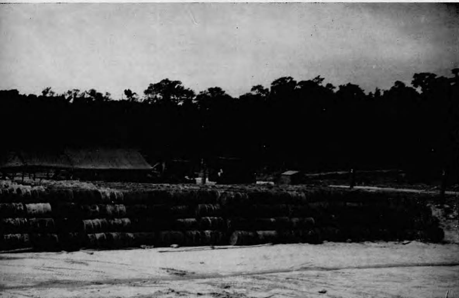
How we finished—the cement stowed and ready for shipment.
