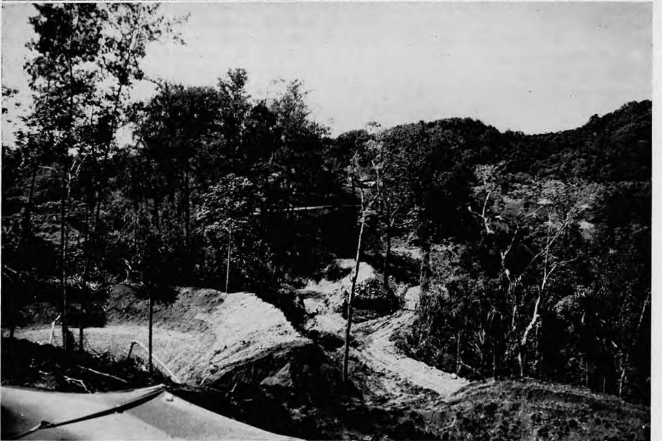
Level ground for tank sites was scarce and sites such as that shown above were often used. Lower, a completed tank site is shown.
