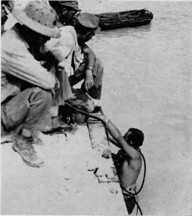
The diver goes down to check progress.
