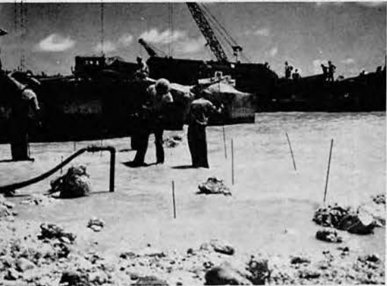
Cleaning holes we have drilled preparatory to setting dynamite charges.
