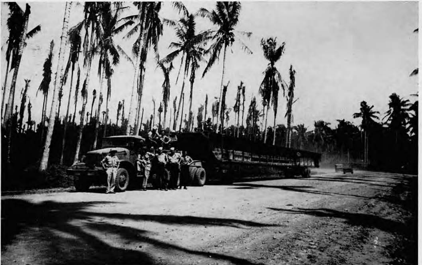
The strings of "Big Joe" move to the job.
