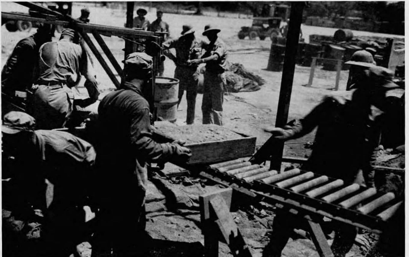
The conveyor lines to the hopper.
