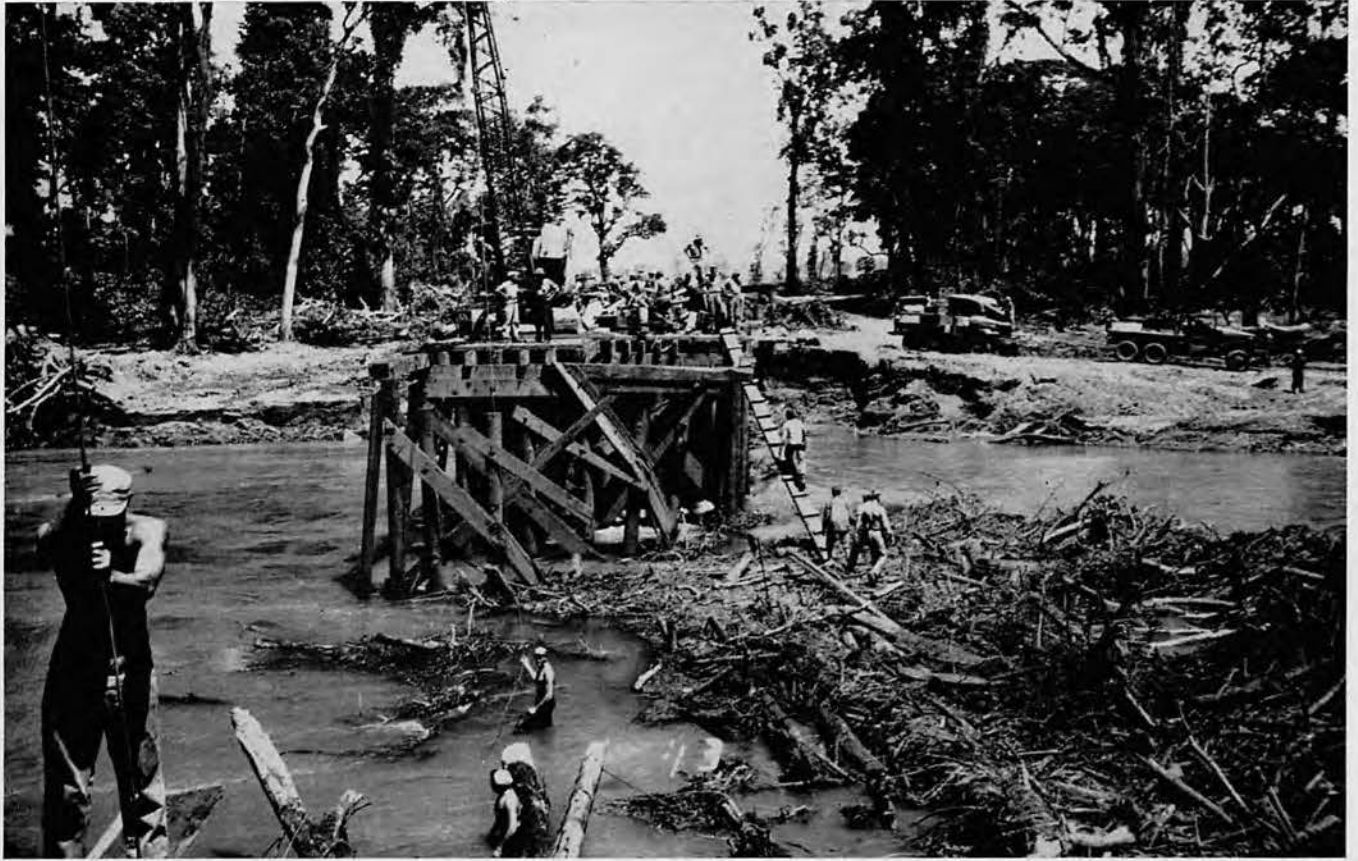
Removing the last of the wreckage.
