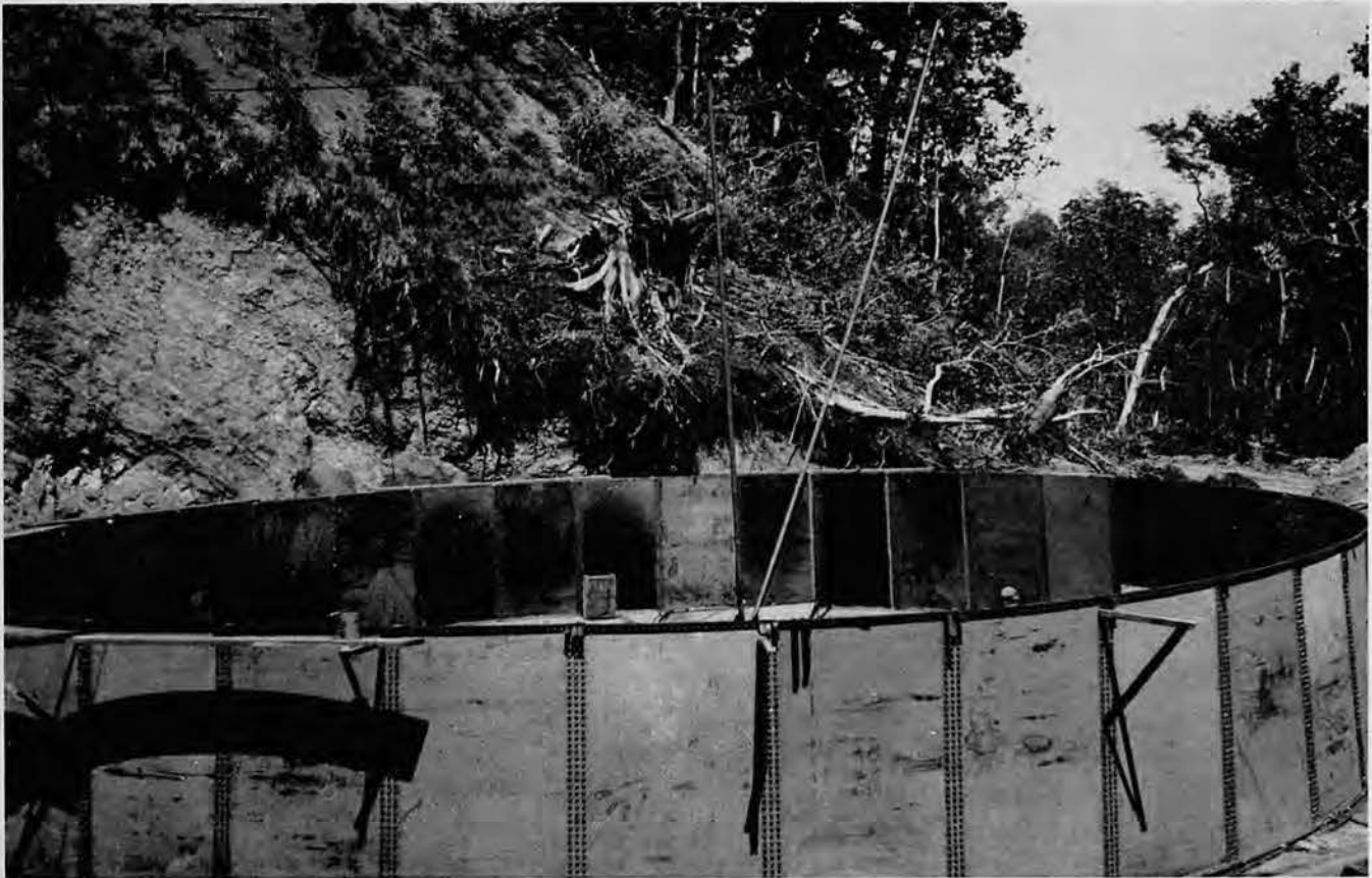
The walls rise.
