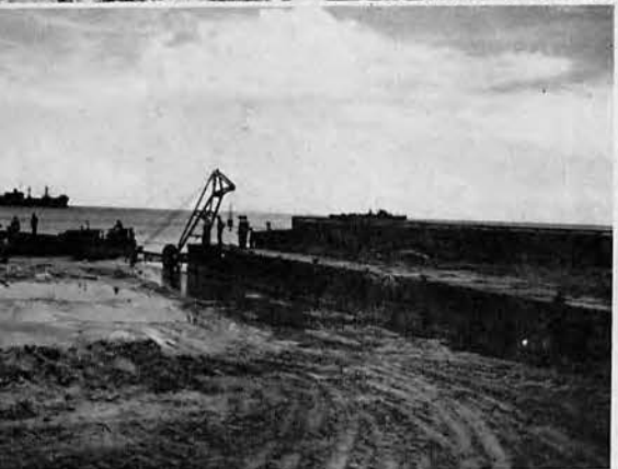
Setting strings which will form edges of the slips.
