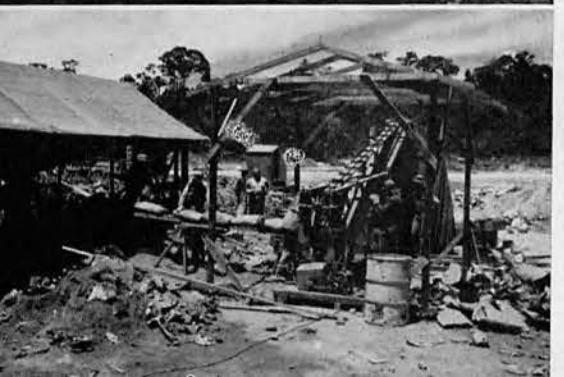
The "contraption" starts to work on reclamation of 31,000 bags of partially spoiled cement.
