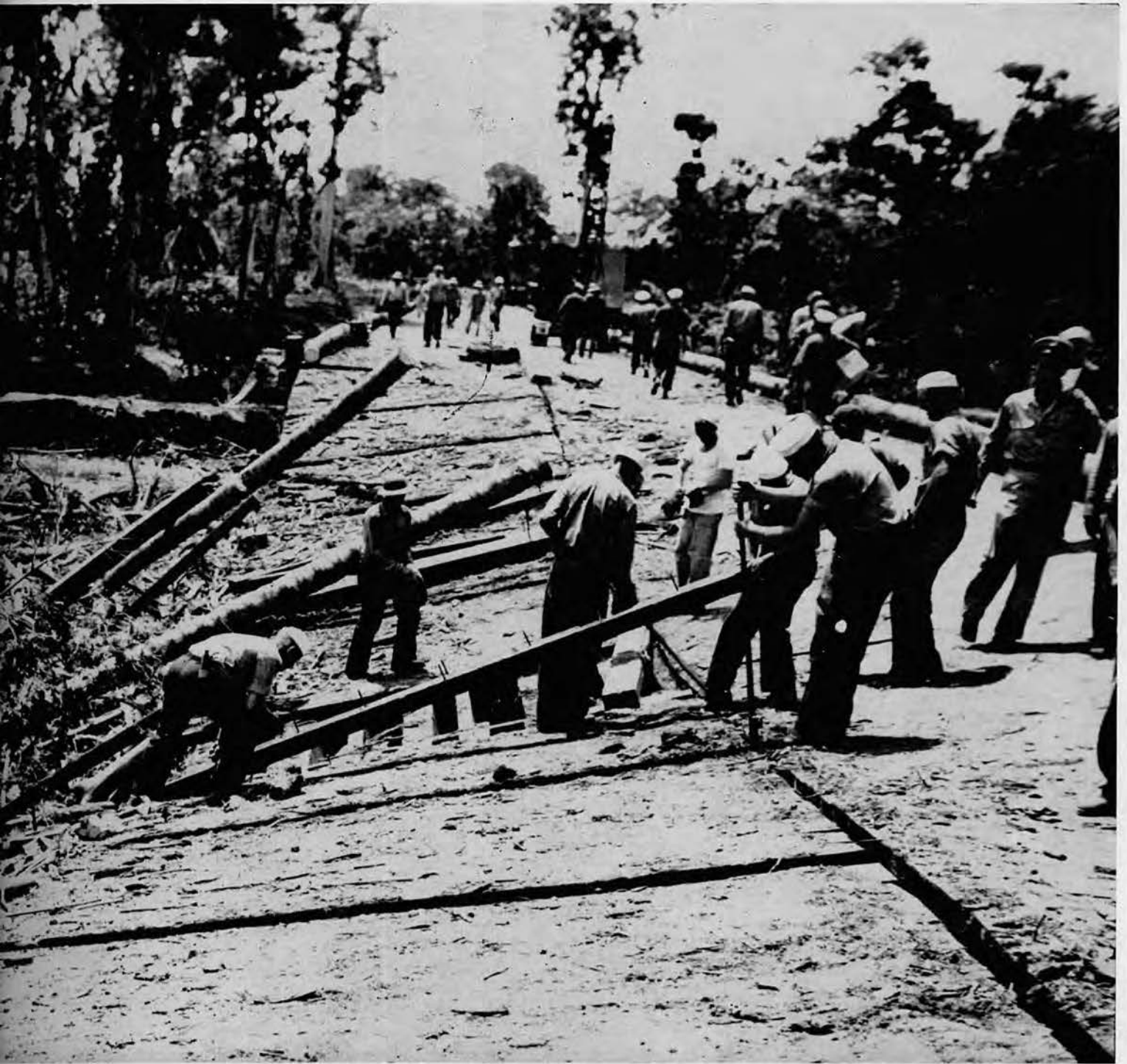
Clearing the debris.
