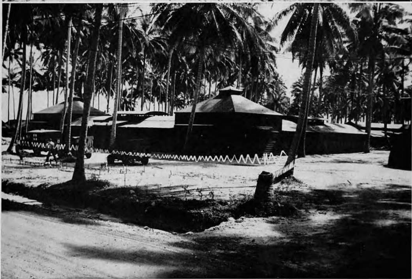
One of our crews erects a warehouse at the Naval Base (upper photo). The Naval Base Sick Bay is shown lower.
