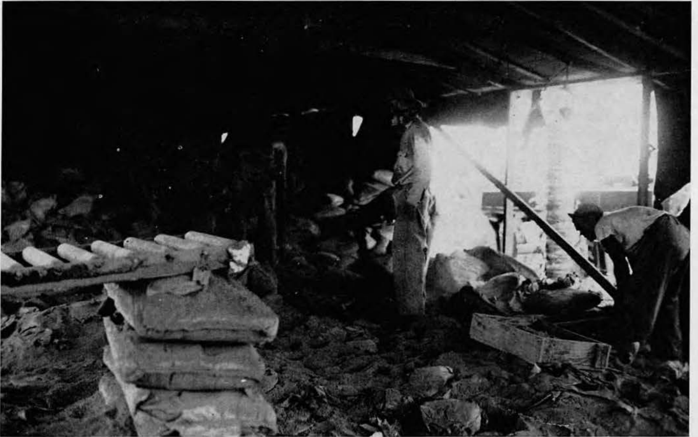
What we started with—the broken sacks inside the warehouse.
