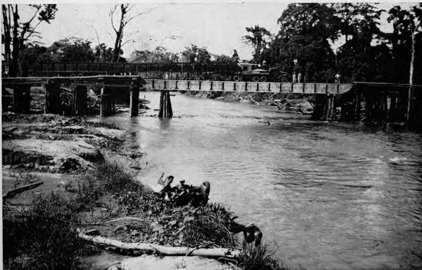
Testing the completed bridge.
