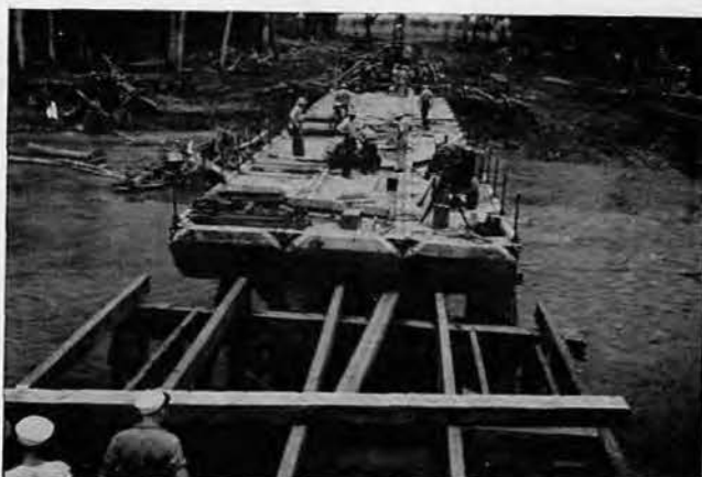
The Strings Set. All that remains is to frame the approaches.
