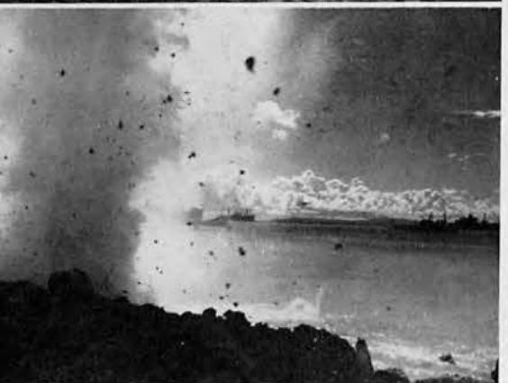
Blasting the coral end of the slip.
