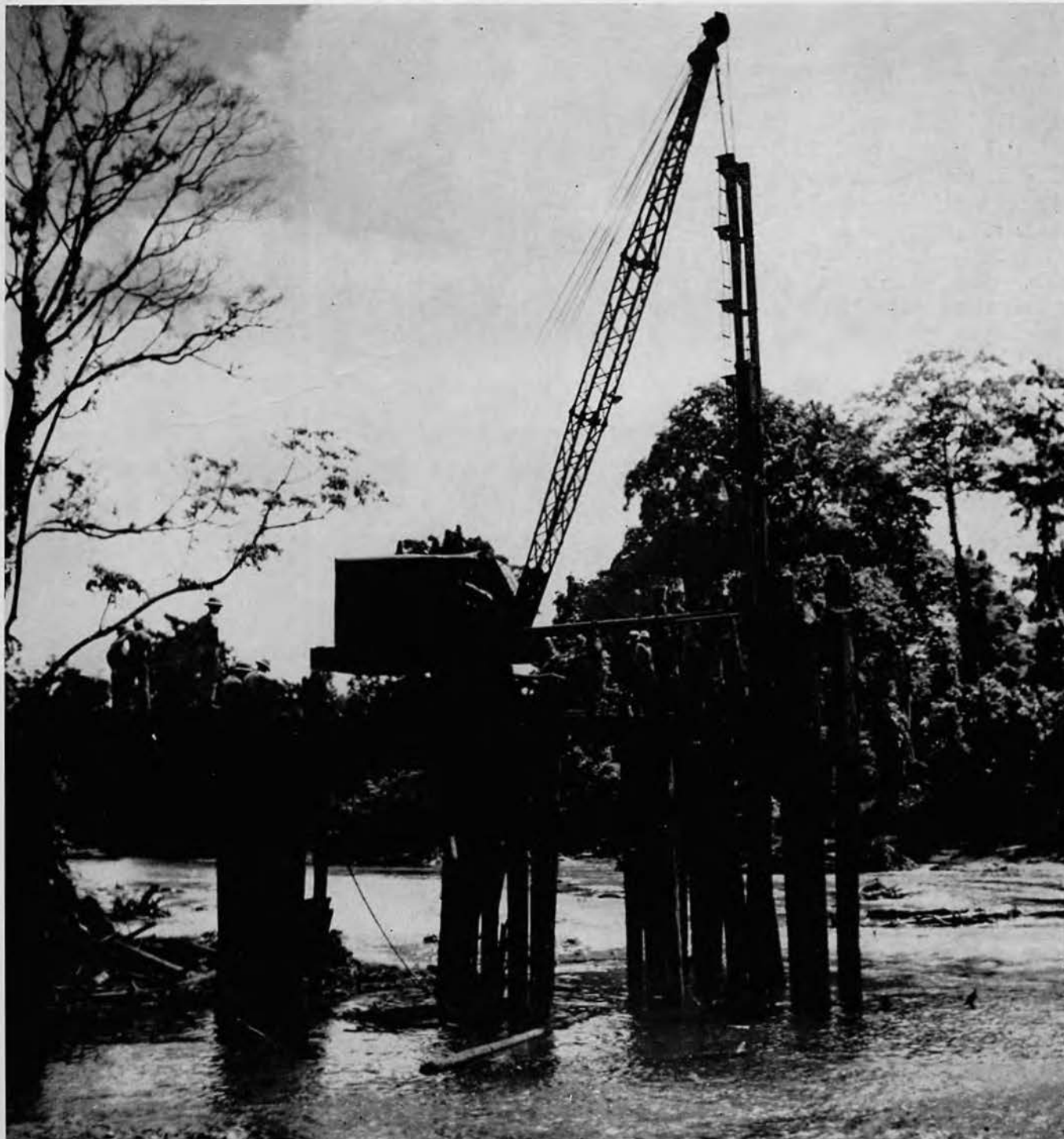
Driving the new bents.
