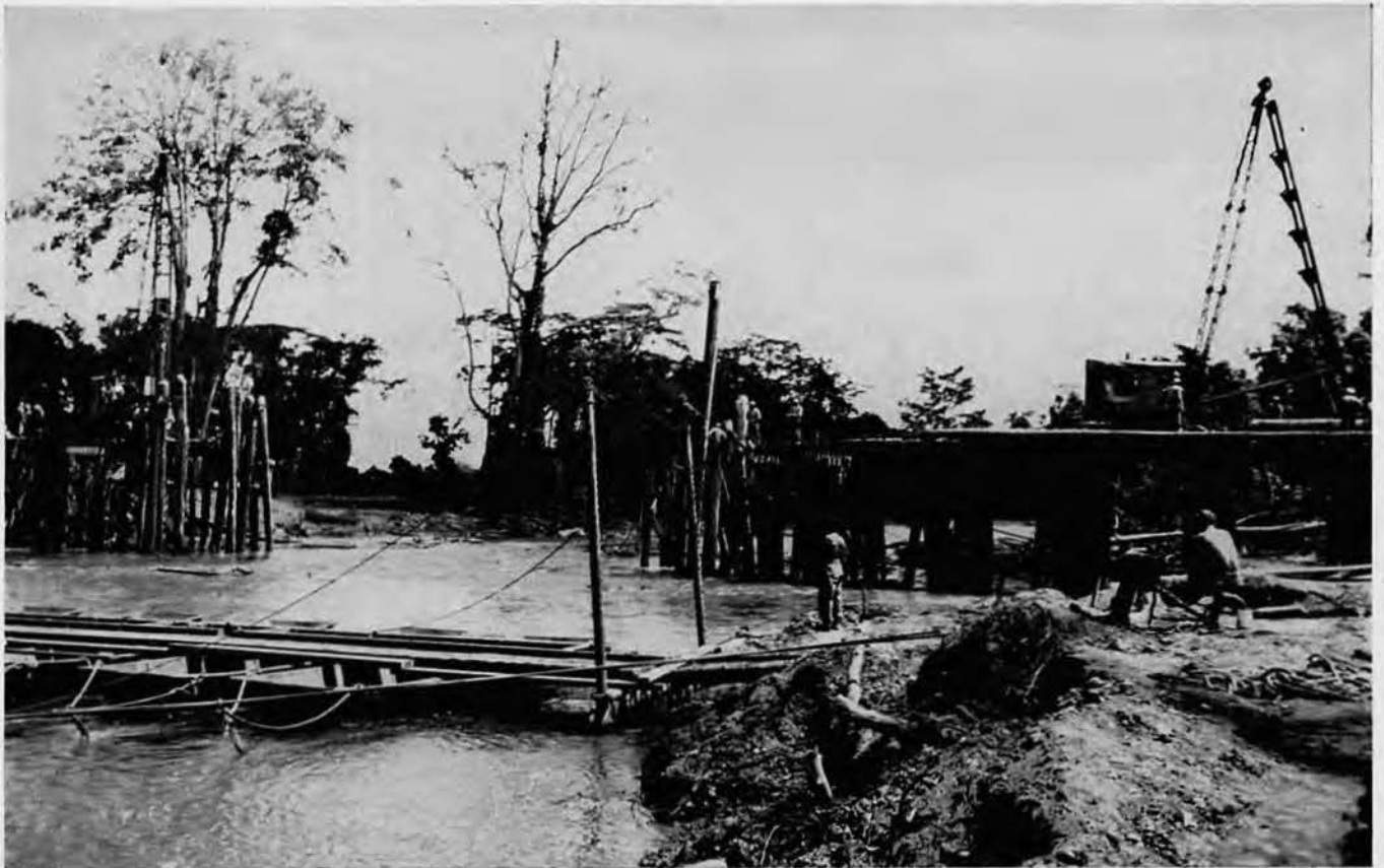
The pile driving is completed.
