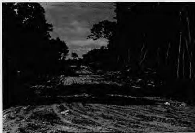
A roadway cleared and rough grading started on the roadbed.
