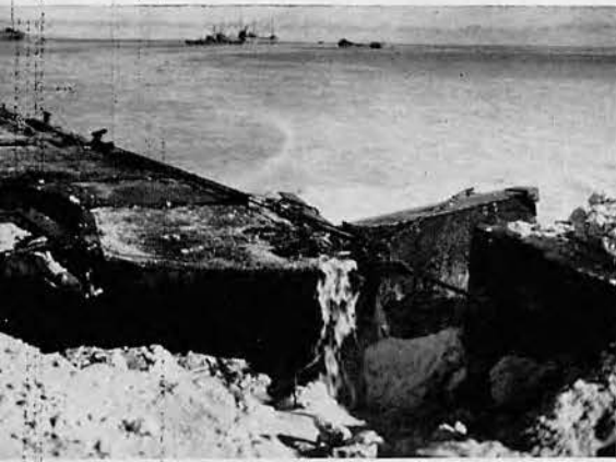
The wrecked in-board end of the piers.
