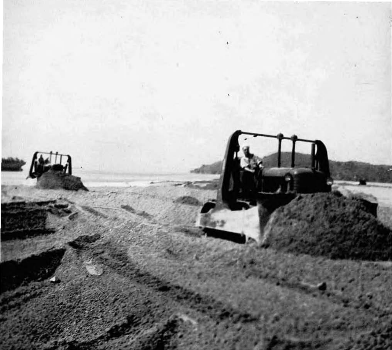
From dredge to dozer.
