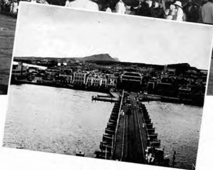
Pontoon bridge at Willemstad.
