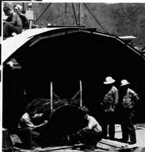
Net gate barge.
