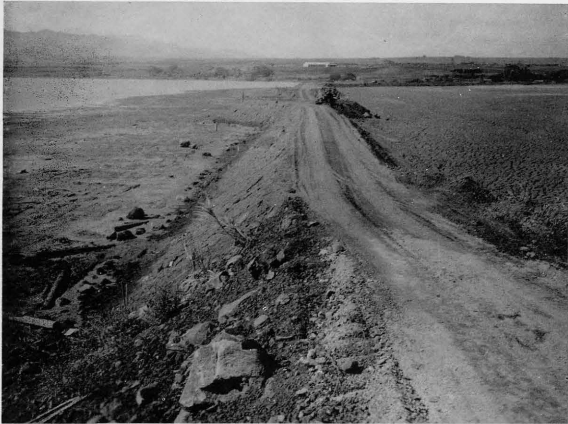
LOOKING ALONG DYKE
