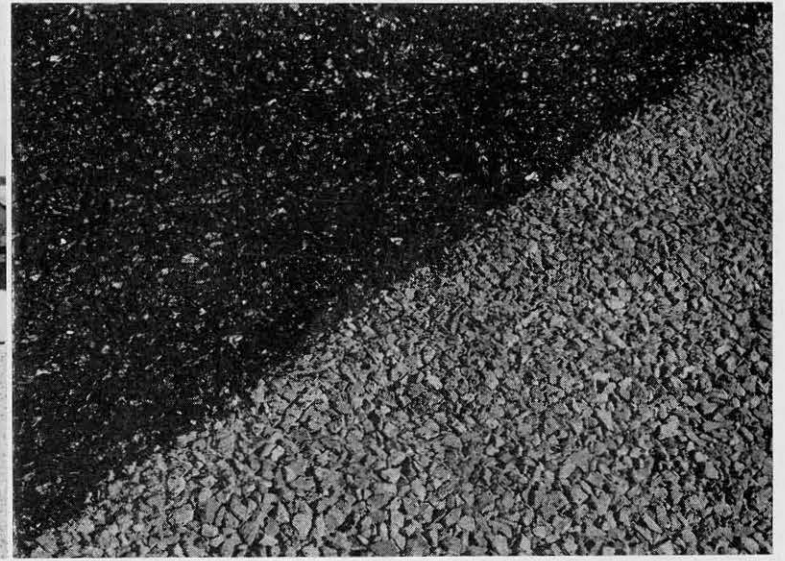
FINAL ROLLING APPLYING BITUMUS
