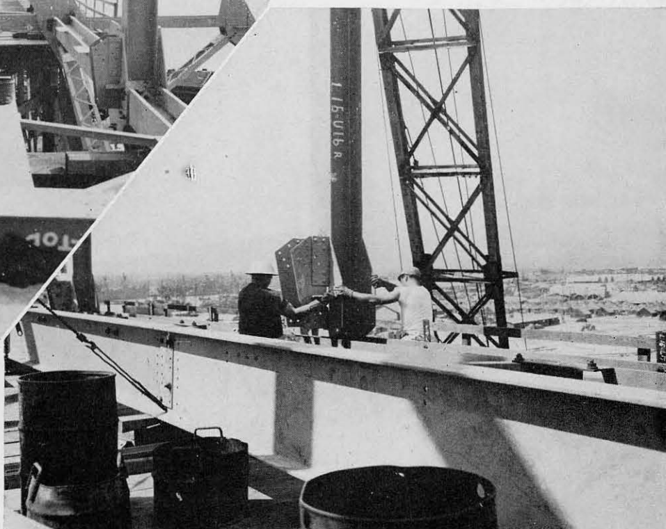
PLACING A GIRDER
