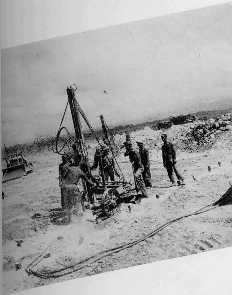
DRILLING HOLES TO SET CHARGES
