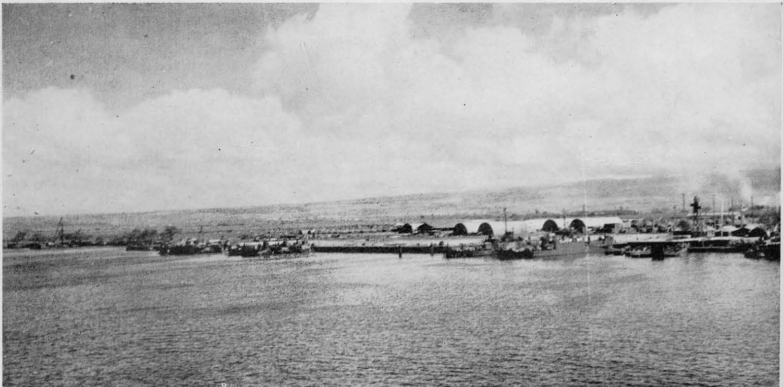
OVERALL VIEW OF WATERFRONT CONSTRUCTION SITE
