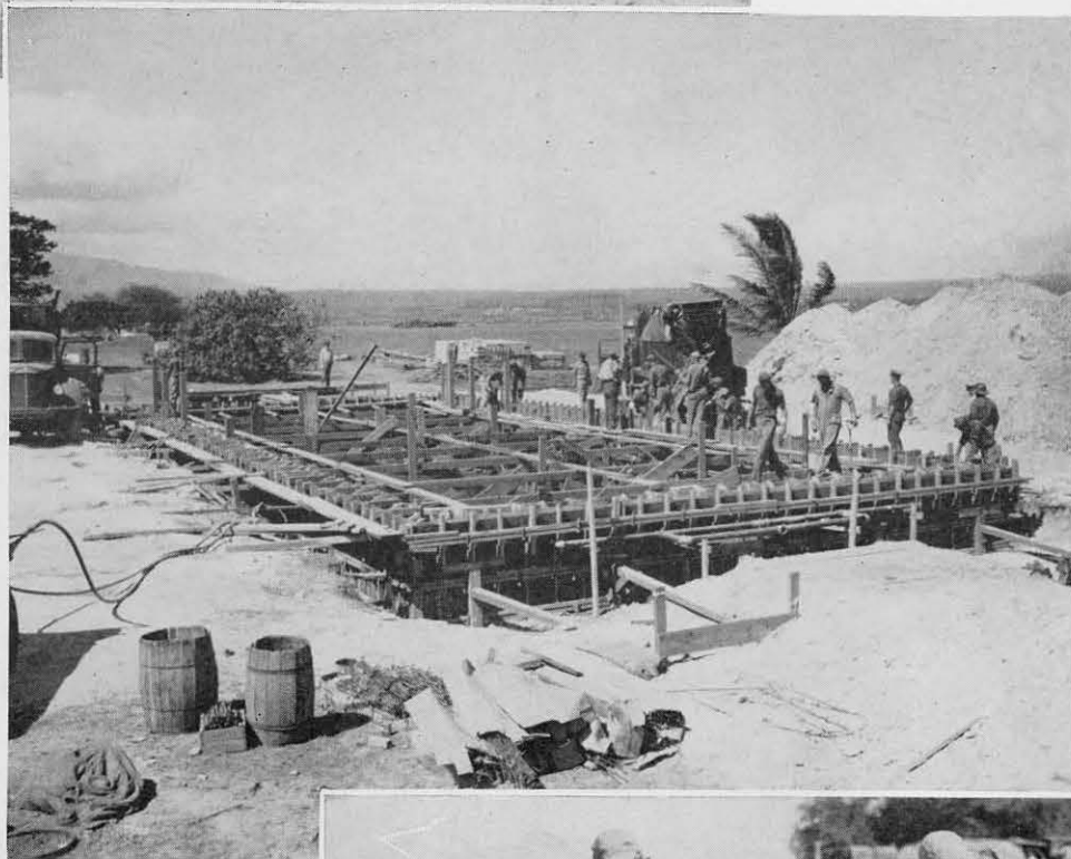
PLACING CEMENT FORMS
