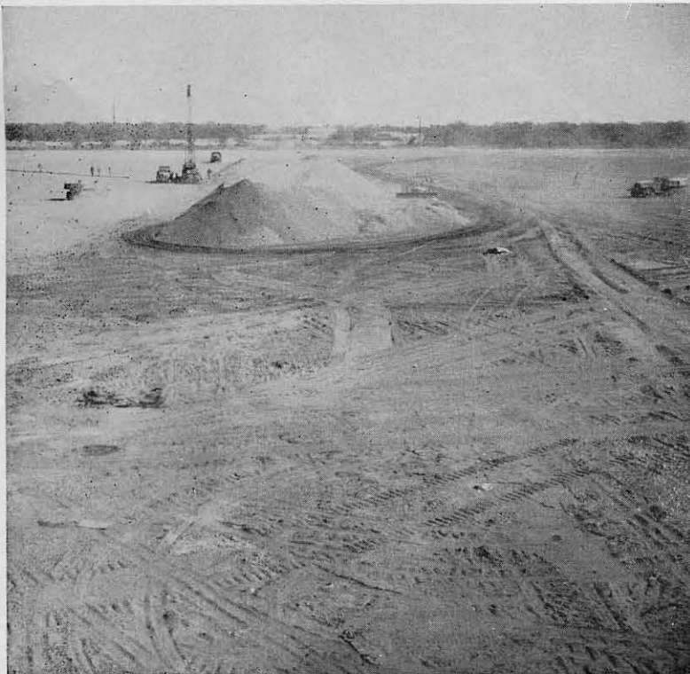
FINISHED SUB GRADE AND ROCK STOCK PILE
