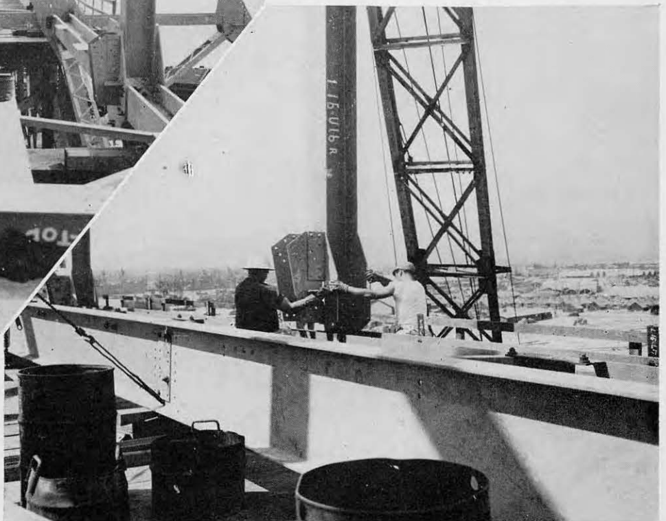
PLACING A GIRDER
