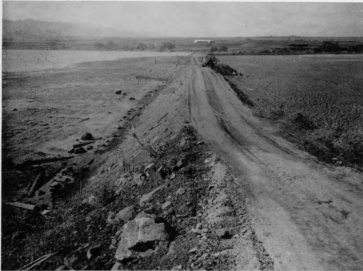
LOOKING ALONG DYKE
