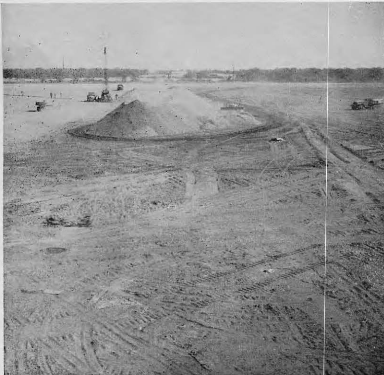
FINISHED SUB GRADE AND ROCK STOCK PILE
