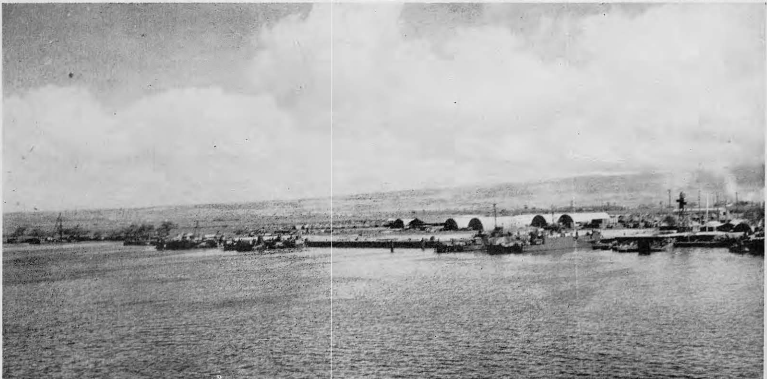
OVERALL VIEW OF WATERFRONT CONSTRUCTION SITE
