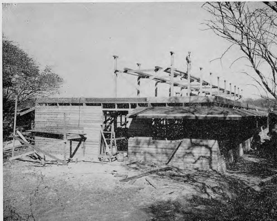
SHOWER ROOM NEAR COMPLETION
