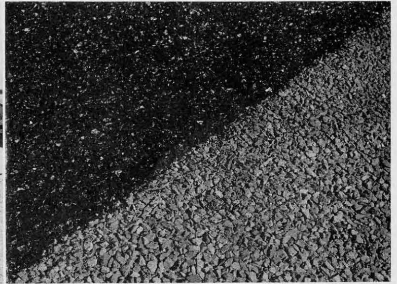
FINAL ROLLING APPLYING BITUMUS
