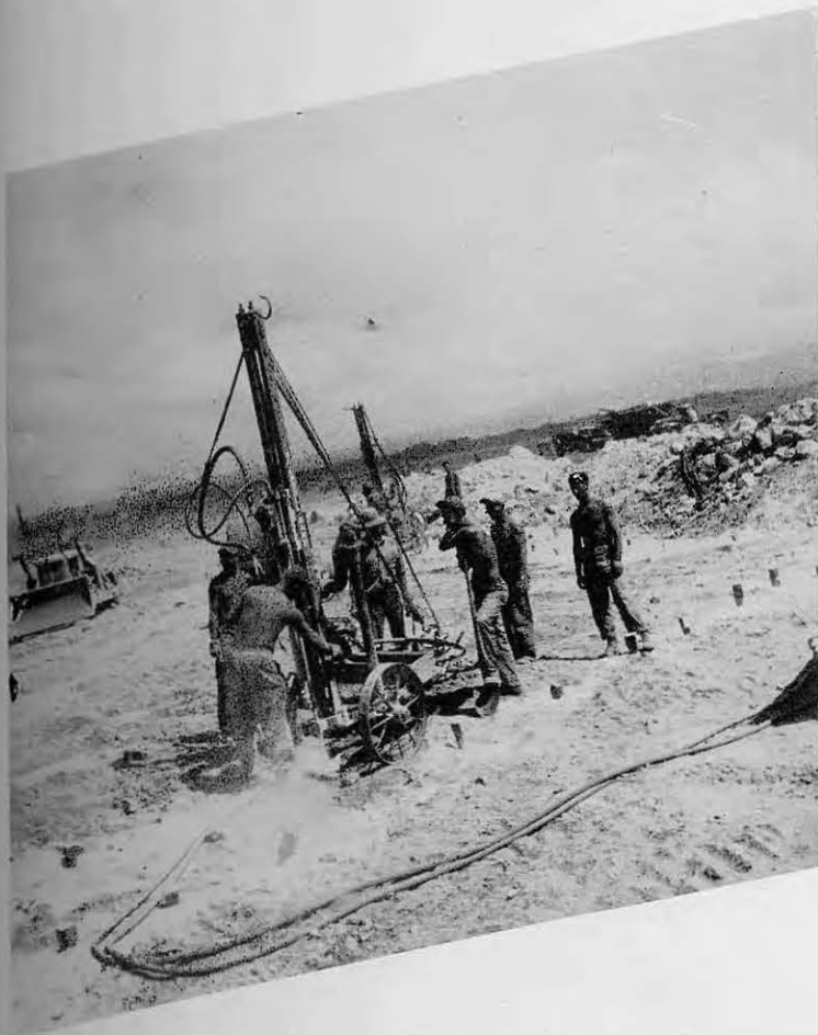
DRILLING HOLES TO SET CHARGES
