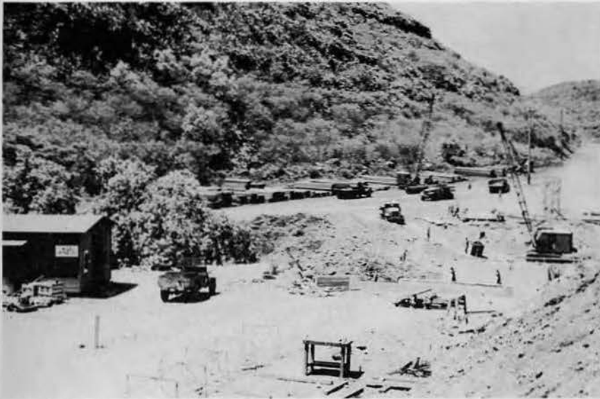
HEAVY EQUIPMENT LOADS BUILDING MATERIAL
