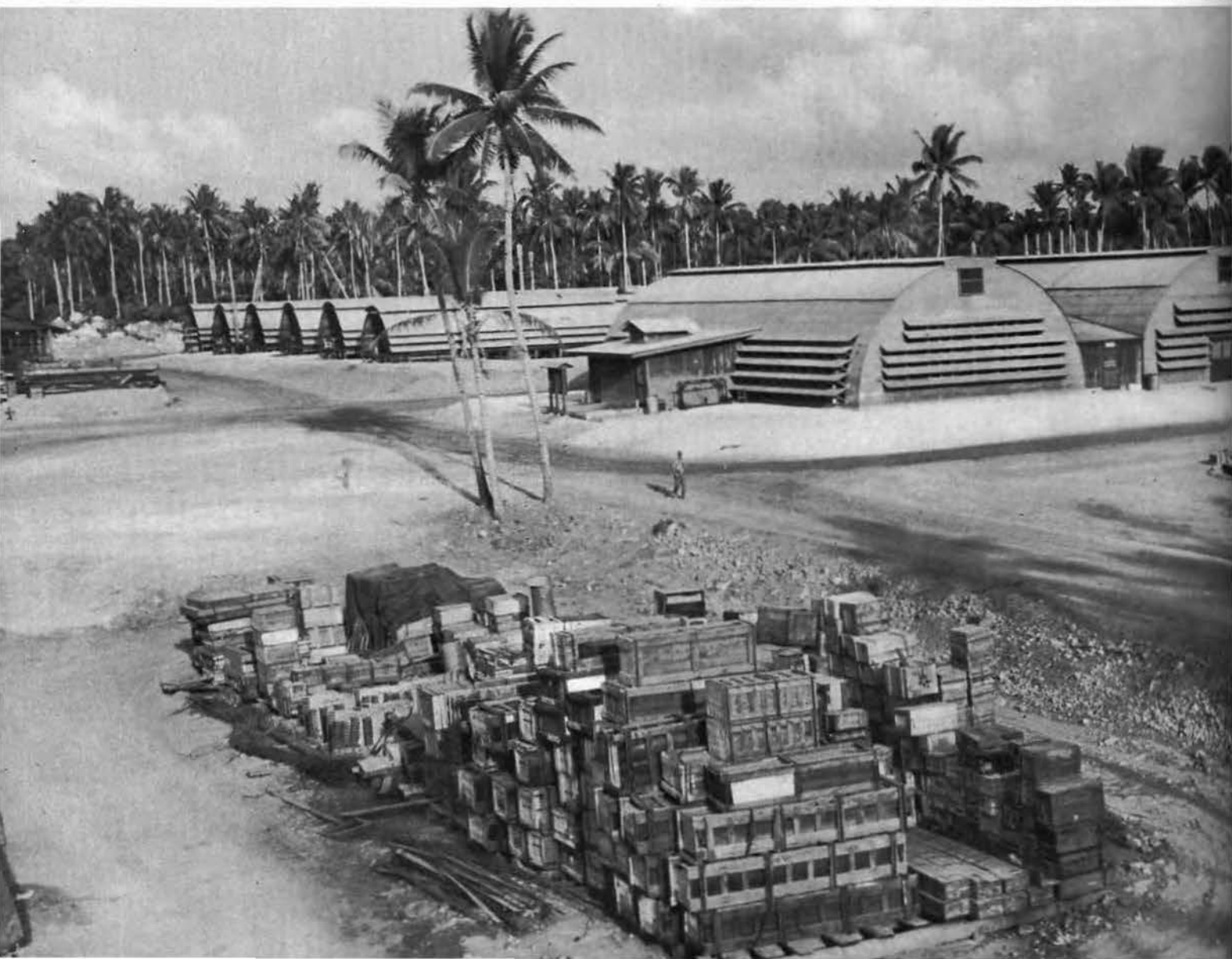
VIEW OF CHOW HALL IN FOREGROUND AND SECTION OF CAMP AREA
