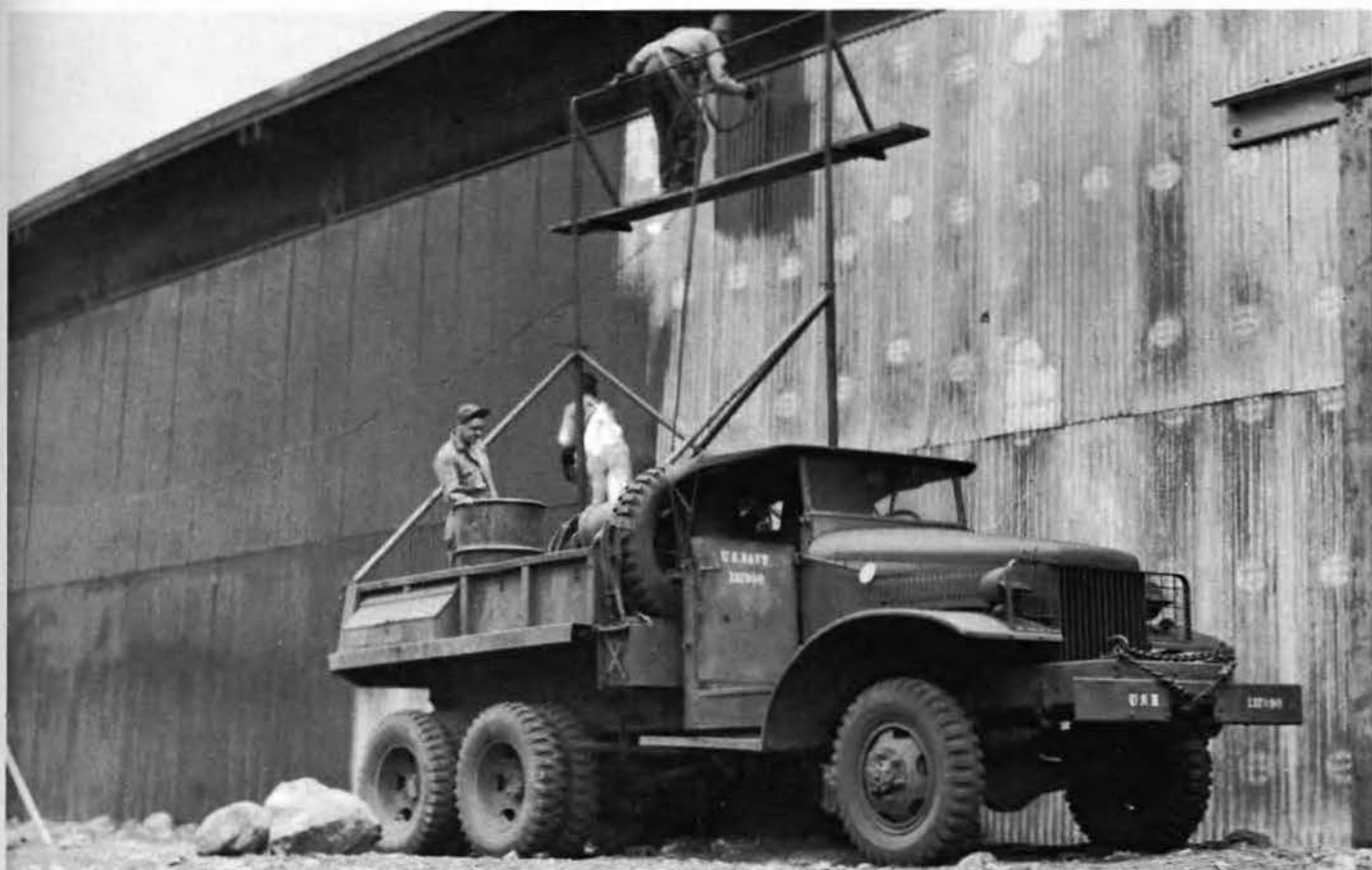
MOBILE PAINT UNITS ADDED THE FINISHING TOUCHES WITH DISPATCH AND THOROUGHNESS
