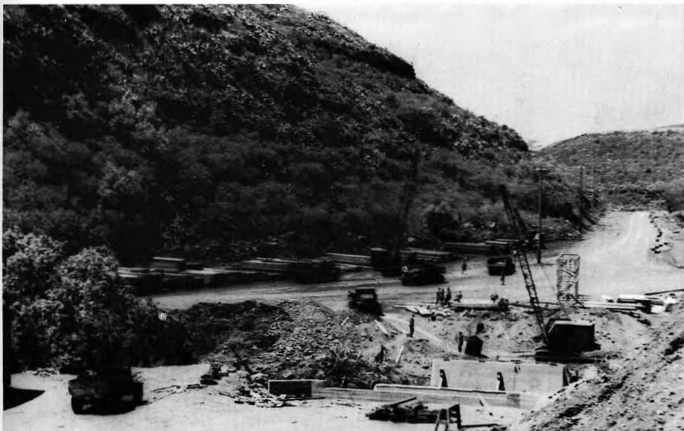
BRIDGING "GULCH CREEK" WAS A MAJOR JOB OF CONCRETE AND STEEL
