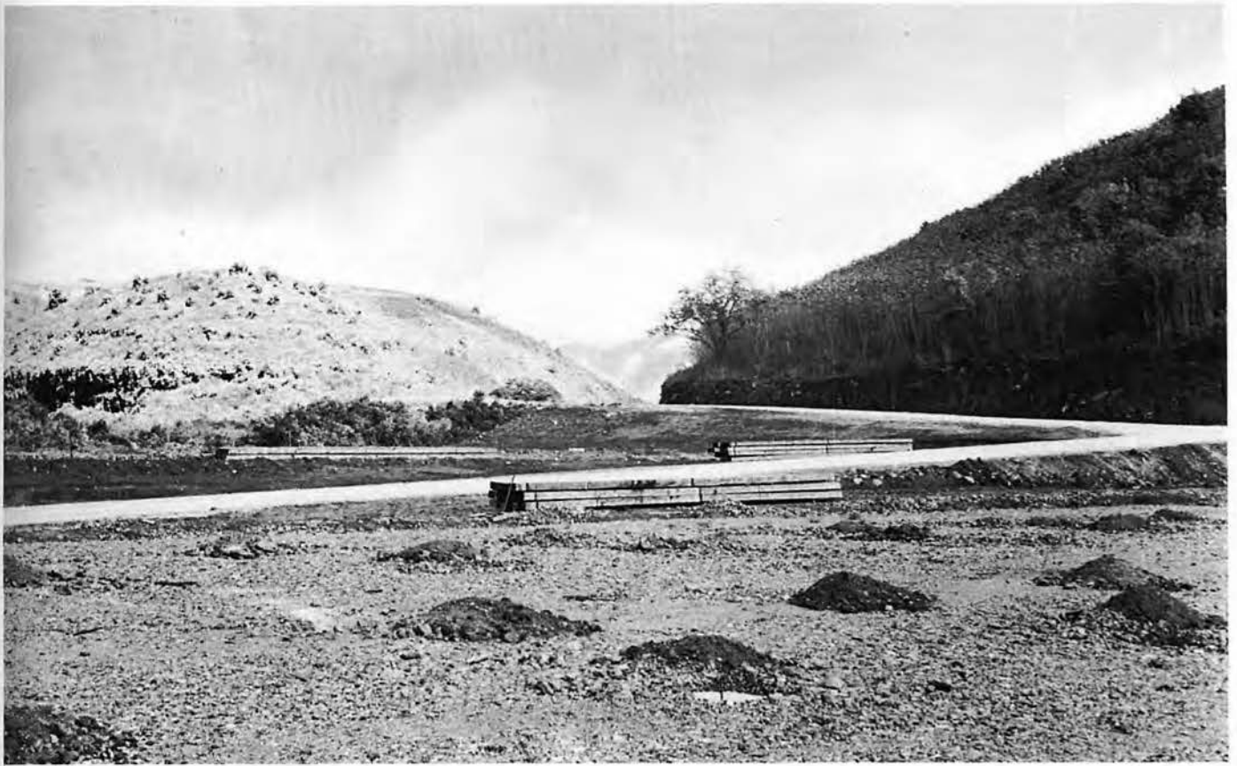
THE FIRST ROADWAY AND CONSTRUCTION SITES TAKE FORM
