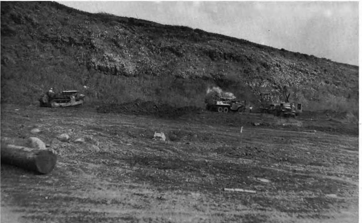
GROUND WAS BROKEN AS HILLSIDES WERE CUT AWAY AND VALLEYS FILLED
