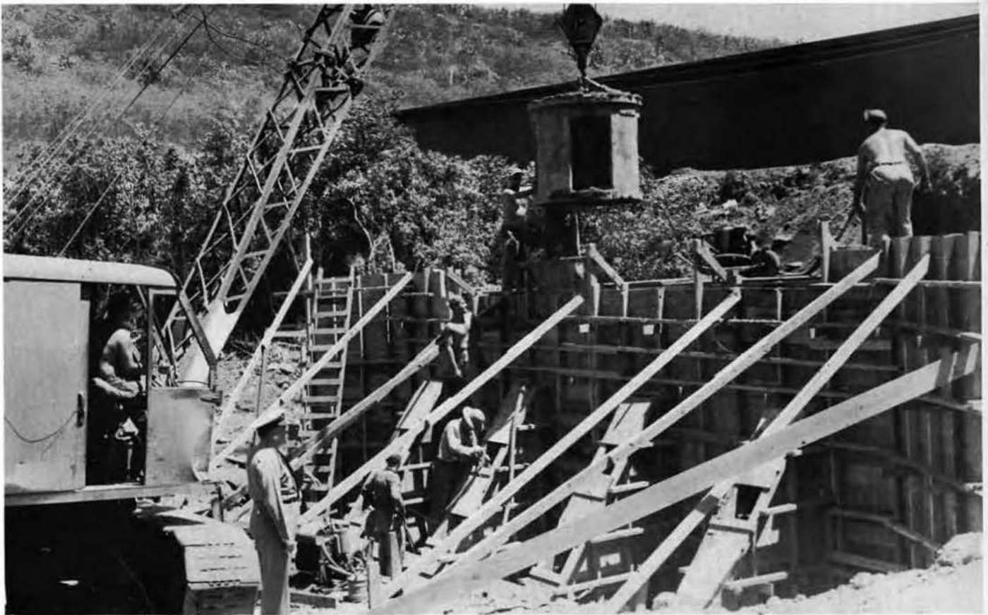
POURING CONCRETE FOOTINGS
