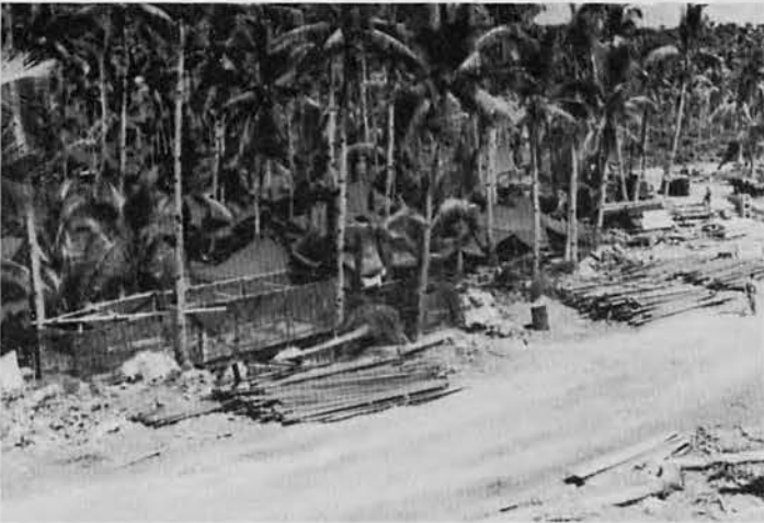
INITIAL PIPE DUMP
