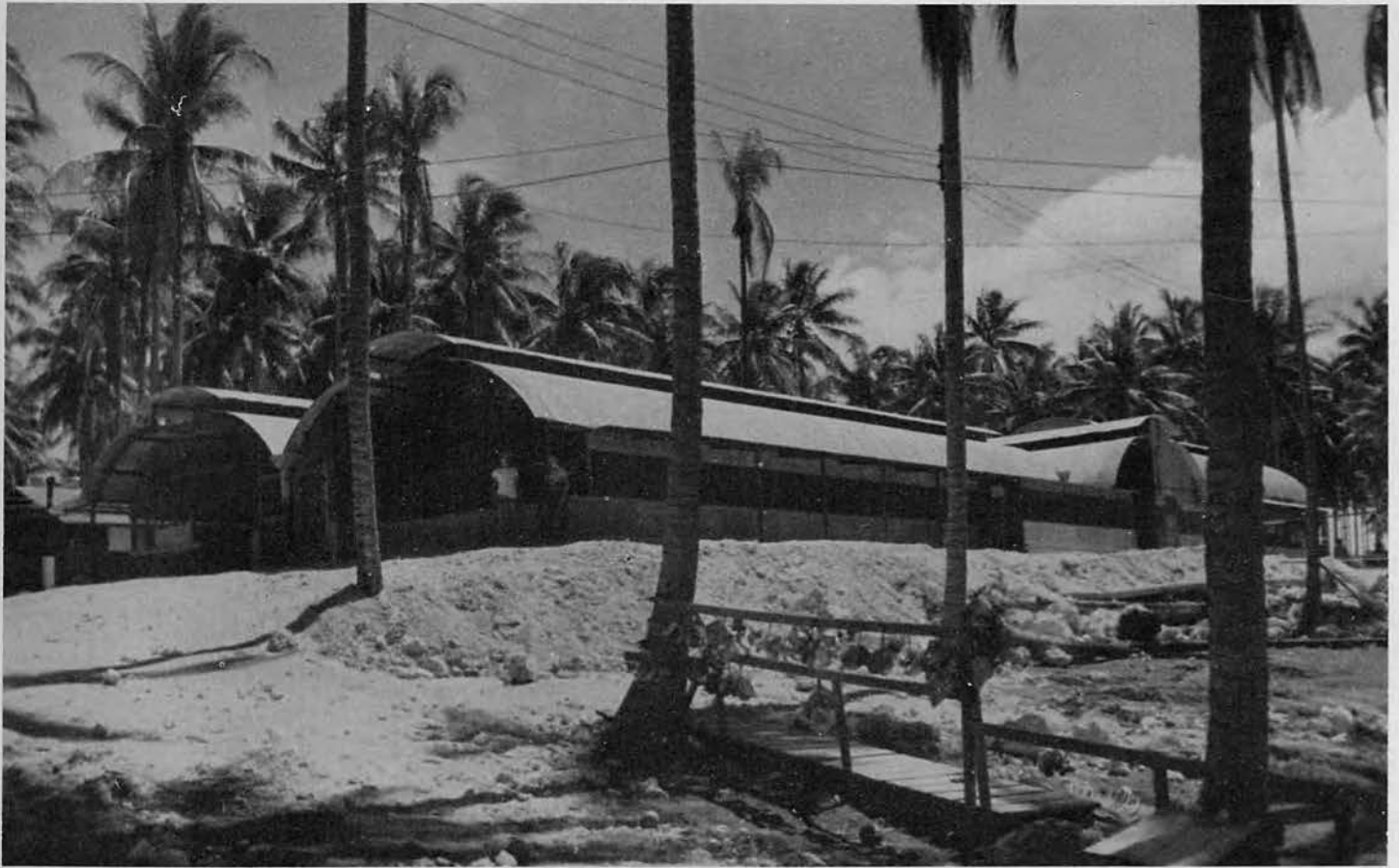
THE NEW MESS HALL AND GALLEY
