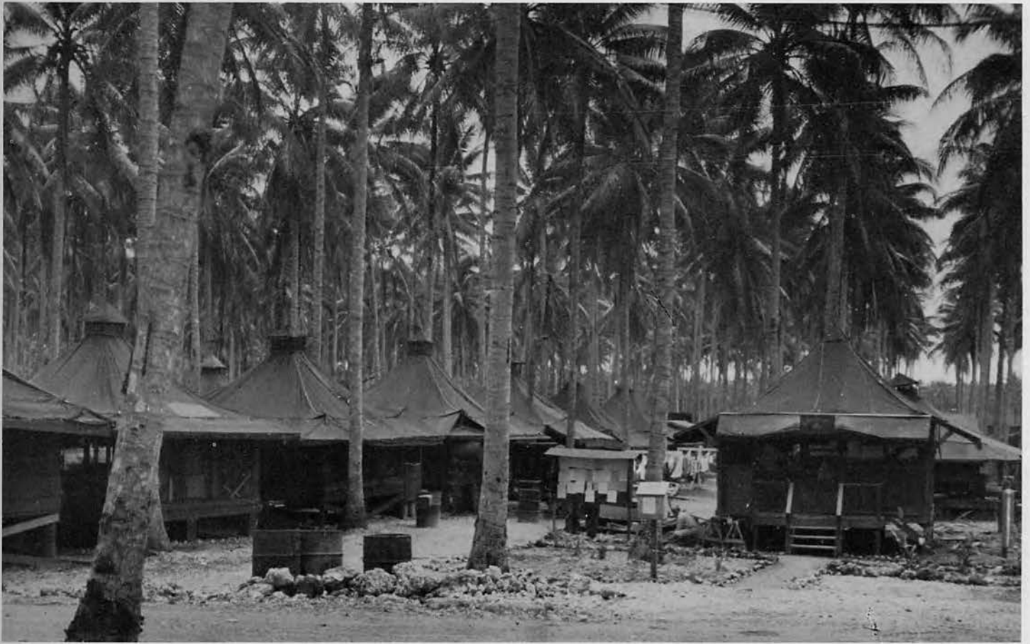
"A" COMPANY STREET
