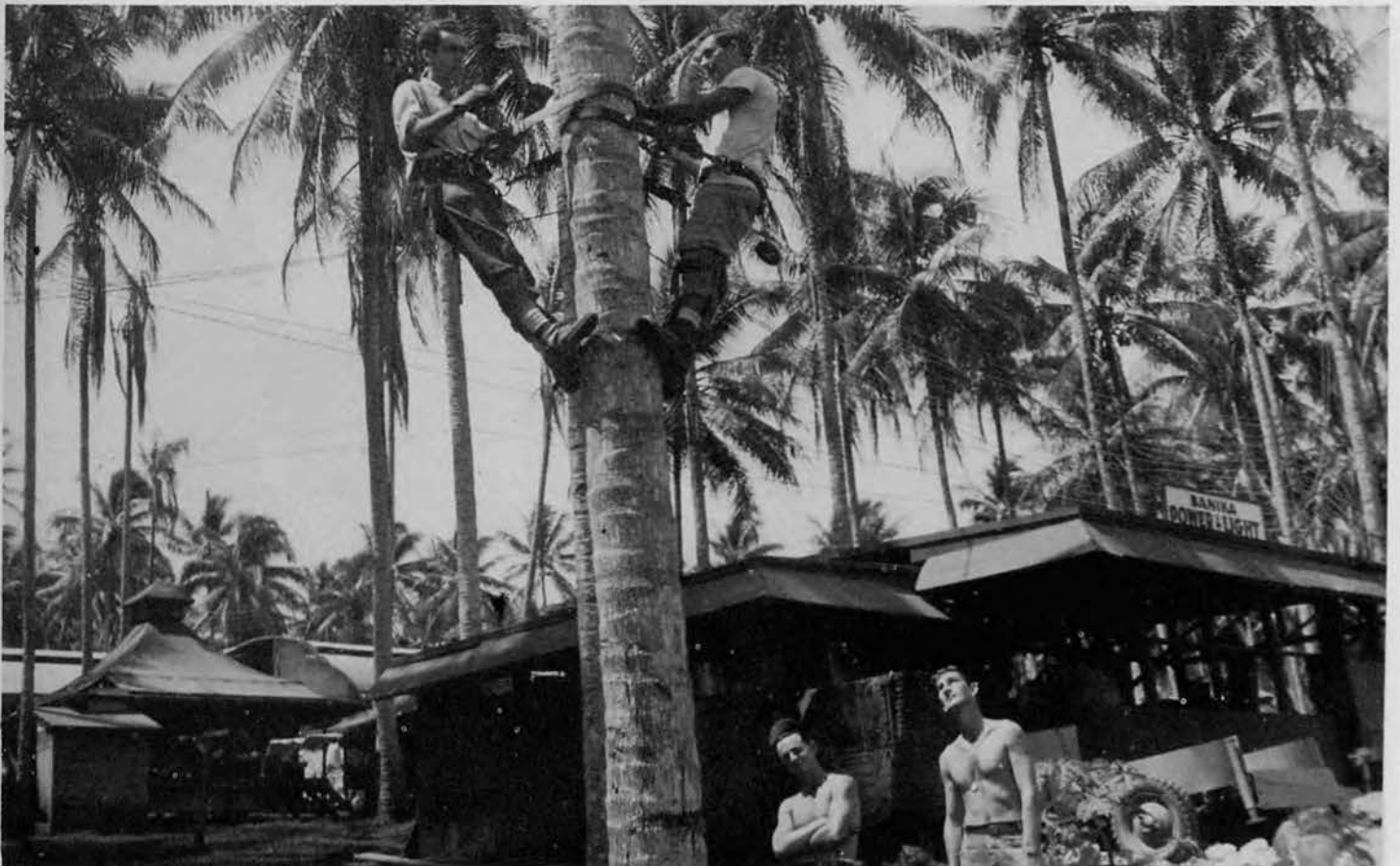
ELECTRICIANS AT WORK
