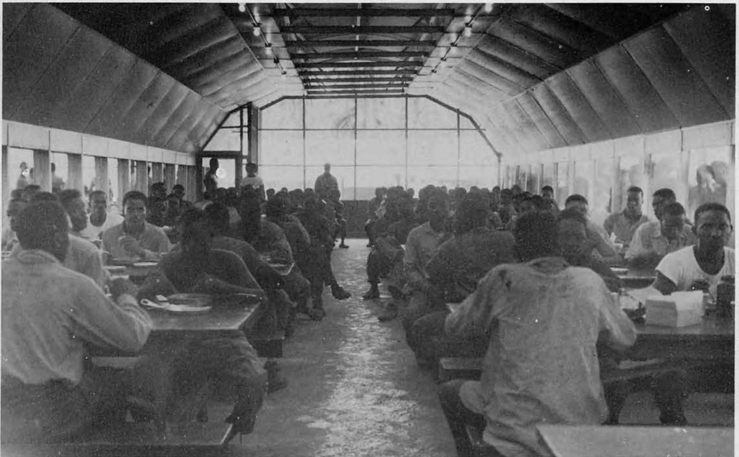
INSIDE MESS HALL
