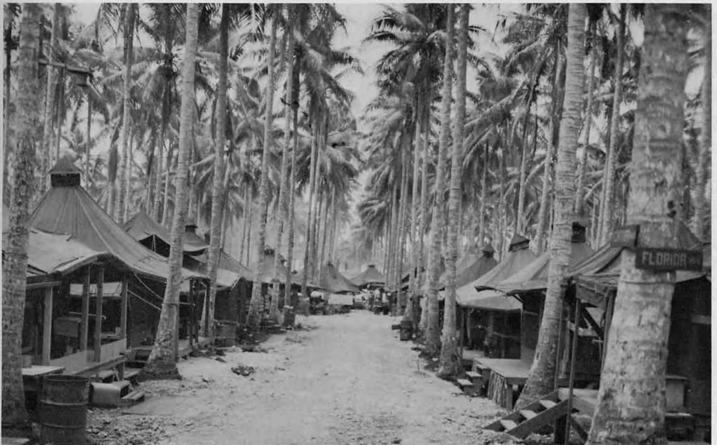
"B" COMPANY STREET
