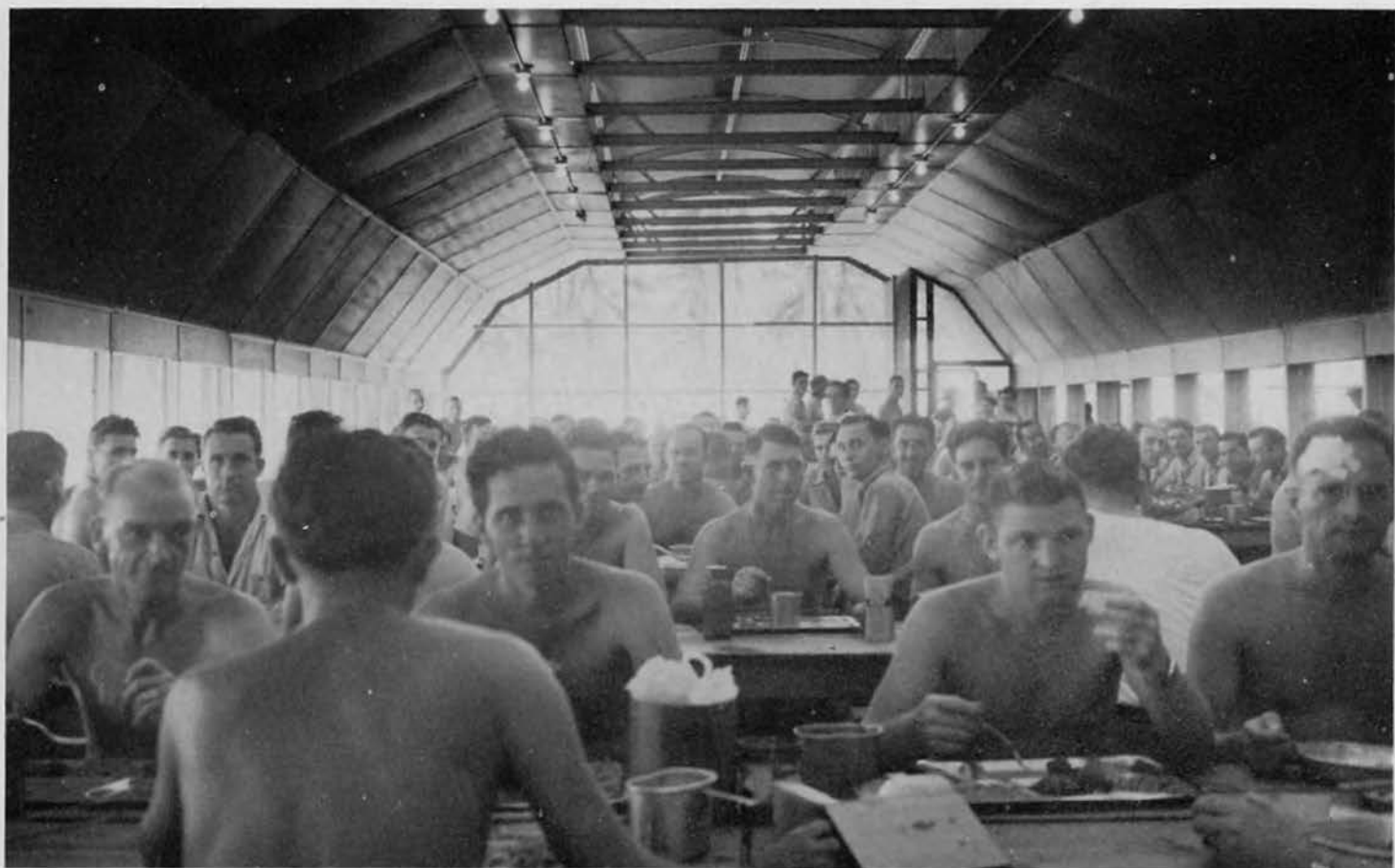
INSIDE MESS HALL
