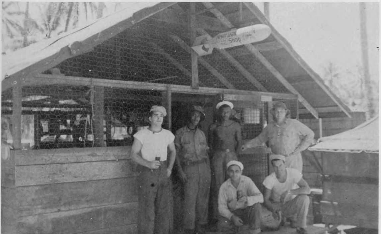
"NEVERLEAK" PLUMBING SHOP
