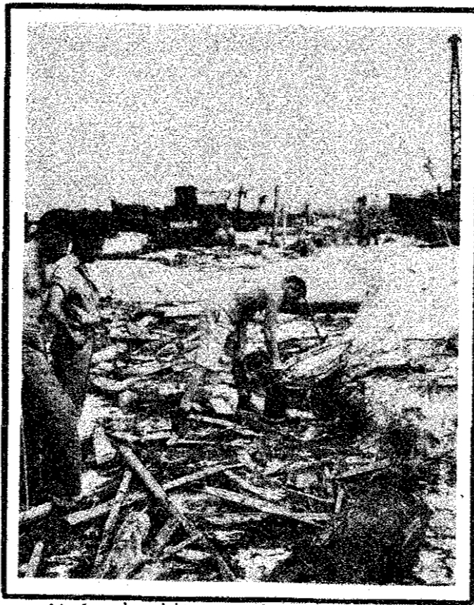
Marines demolition experts — Orange Beach
