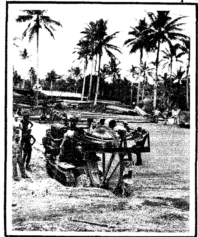
Ditch-digger prepares way for water-pipes
