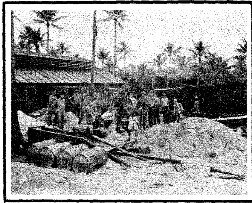
Cheekers as well as carpenters pour the footing - 20th May
