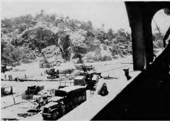
Company B's Dock Area
