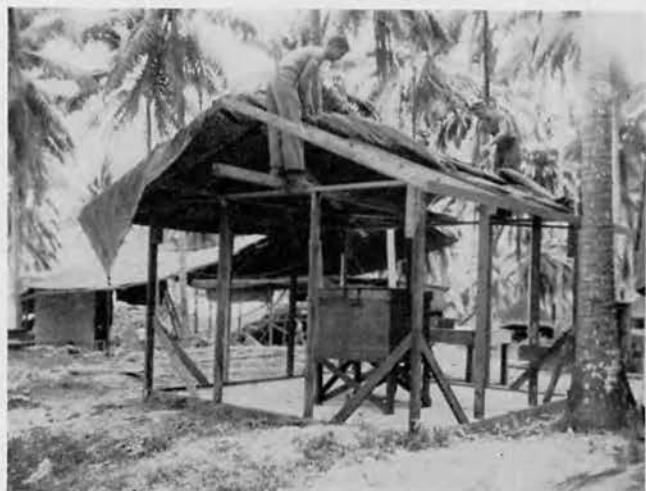
Erecting Public Drinking Fountain on Russells
