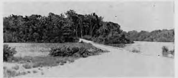
Bridge Connecting Sasavele and Roviana Islands
