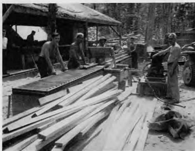
Jap Motor Powering a Home-made Saw
