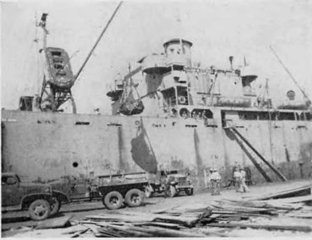
Stevedore Operations on Tulagi Dock
