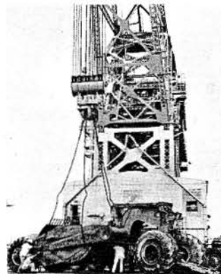
HEAVY EQUIPMENT IS HOISTED BY CRANE
