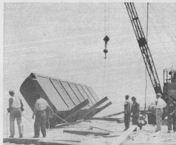
Fig. I-12 A barge assembly string is being launched from a wharf.
