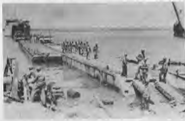
LST discharges vehicles and equipment onto pontoon causeway.
