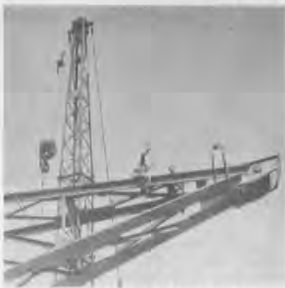
Ship repair requires heavy cranes.
