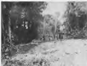
Roadwork must begin on D-day.
