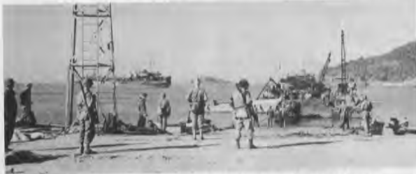
Pontoon pier being set up by Seabees to unload supplies at Korea.
