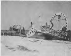
Seabees use a Gilhoist to lift a landing craft out of the water.
