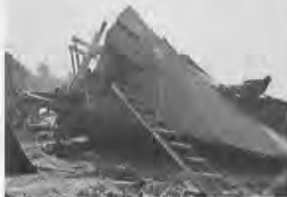
Cruiser bow section is a typical ship repair job.
