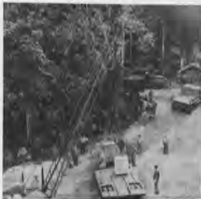
Cherry picker unloading cement clumps.
