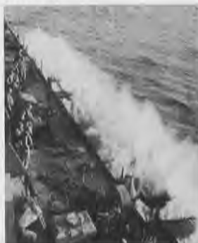
Seabees chop lashings and launch pontoon causeway.
