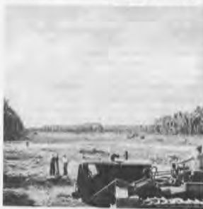
Seabees ready to begin final surfacing.
