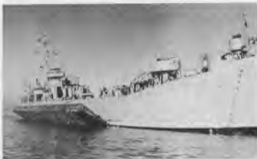
Pontoon causeway section just before launching.
