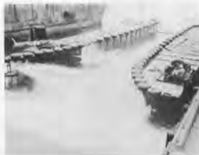
Pontoon seaplane berth tests water jets.
