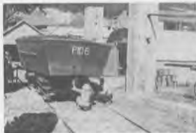
Marine railways are efficient for servicing small boats.
