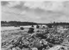
This rock will make good sub-grade.
