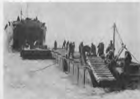
Putting the ramps into position.
