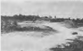
Putting finishing touches on a taxi-way.
