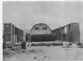
Gate vessel in pontoon drydock.
