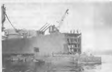
Cruiser with the damaged bow section removed.
