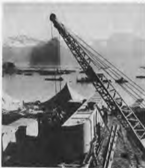
Seabees assemble pontoon string in the Arctic.
