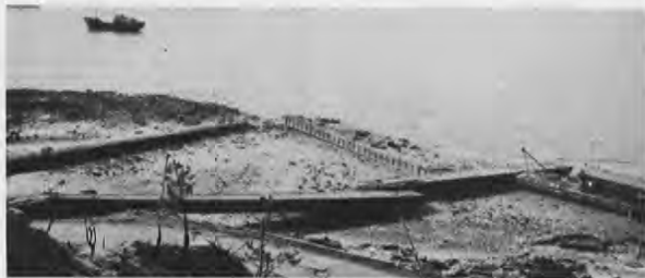
Pontoon barges and causeway set up by Seabees to evacuate troops from Inchon.
