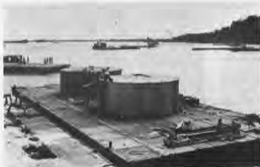
Seabees put finishing touches on fuel barge.
