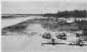
Operations are often underway before strip is finished.
