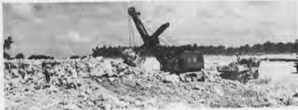
It takes a big shovel to handle rock like this.
