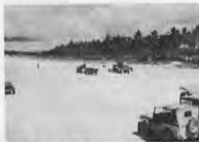
Surfacing shoulders along side runway.
