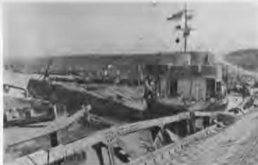
Storm damage at Normandy was a real disaster.
