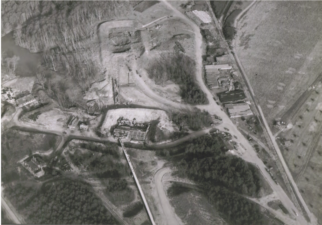
This aerial view shows the incident's relation to the rest of the Depot. The two craters at the top of the picture represent the remains of P-2. Despite the severity of the explosion, the sand and dirt barricades around each building limited the direct impact of the explosion to just to P-2. (HRNM photo)
