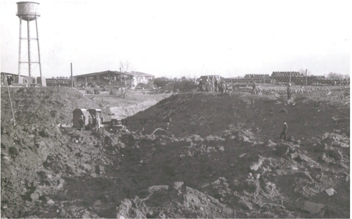
In the middle of the night on November 16, 1943, the equivalent of over 150,000 pounds of TNT exploded at the Yorktown Mine Depot (now known as Yorktown Naval Weapons Station) killing seven workers and causing a noise that could be heard in Richmond and Norfolk. The explosion caused two craters, each twenty-five feet deep and over 150 feet wide, and shattered glass for miles around. (HRNM photo)
