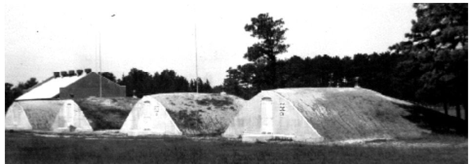
The Navy first opened St. Juliens as an alternative to Craney Island for ammunition storage. These concrete “igloo” type storage facilities are typical structures for storing ordnance. (U.S. Navy photo)
