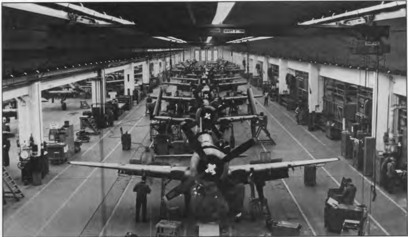
NADEP, Norfolk personnel (then known as the Overhaul and Repair Department) work on Navy Grumman F8F Bearcats on the assembly line in NADEP's Building V-88. The Hampton Roads Naval Museum has several photographs, maps and documents telling the story of one of the most important Navy institutions in Hampton Roads (March 1950 U.S. Navy Photo)
