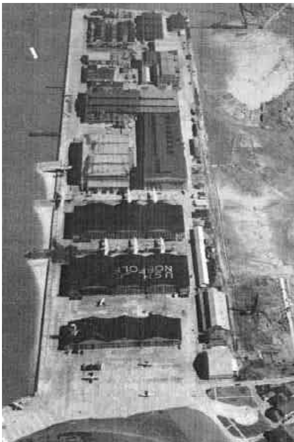
The "SP" or Sea Plane Hangars from the air. Many of the hangars, which were built in the 1940s, are slated to be replaced by newer hangars. (National Archives photo)
