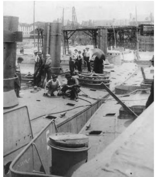
Trigg Company workers take a break while working on the torpedo boat Stockton (TB-31), 1900. (Naval History and Heritage Command photo)
