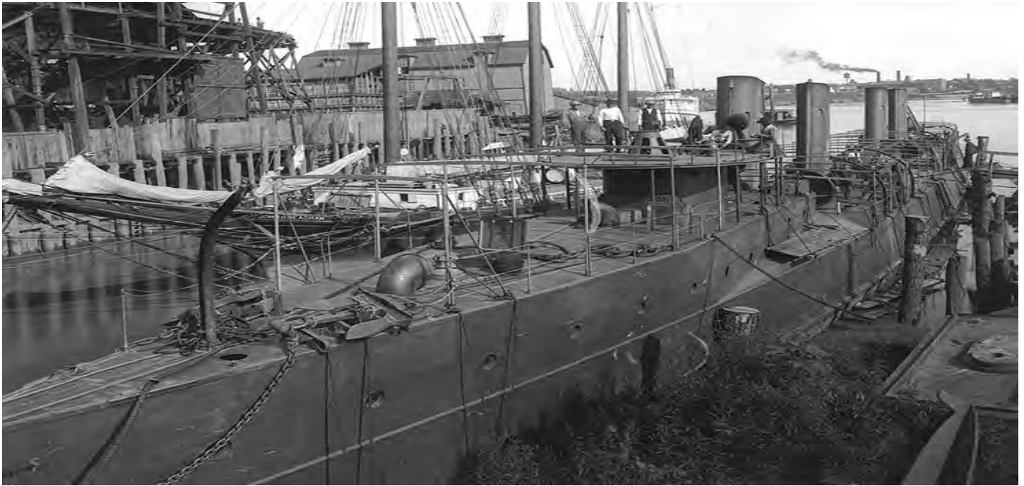
Proud Trigg Company employees pose with the nearly completed Dale. By this point in the construction, the only parts missing were the ship's torpedo tubes and guns. After her construction, Dale then went to the Navy's testing grounds in the Chesapeake Bay to undergo grueling builder's trials. Normally, it took six to seven months after launching for the Navy to accept a new warship. Dale and Decatur, however, were considered such well built ships, that the Navy accepted them in two months. (Naval History and Heritage Command photo)
