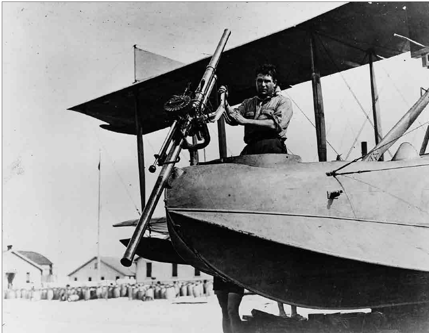
The Davis recoilless antisubmarine gun mounted on a flying boat.
