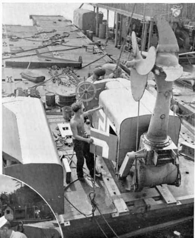
Setting a repaired unit in place aboard a barge.
