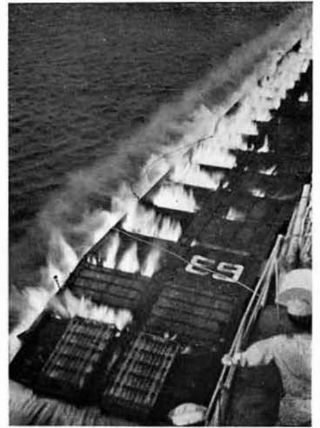
Causeway section hits the water with terrific force.
