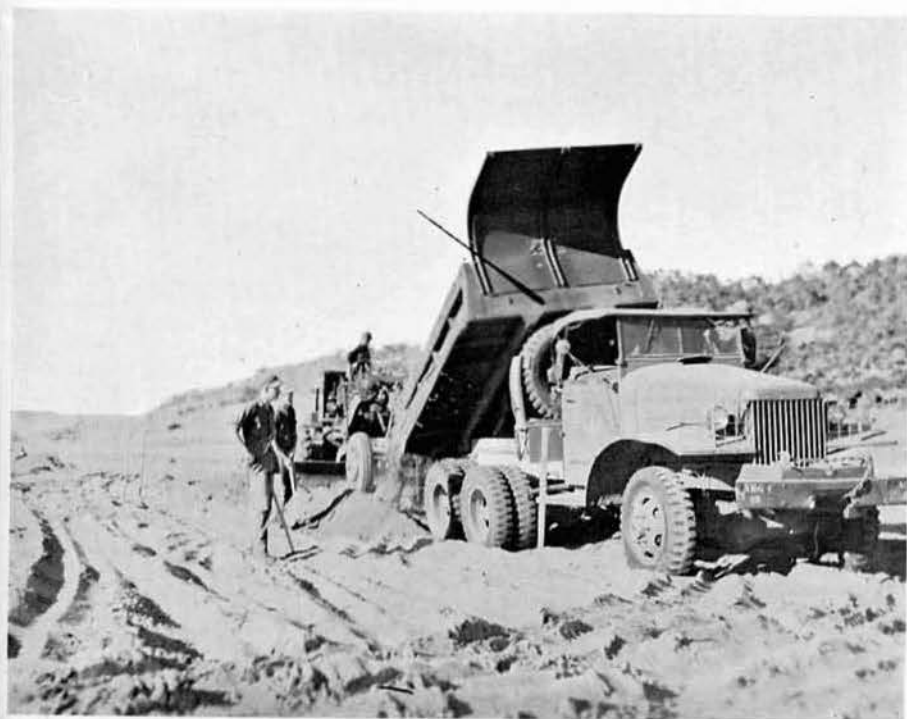
Fill is dumped and the grader does a finishing job.
