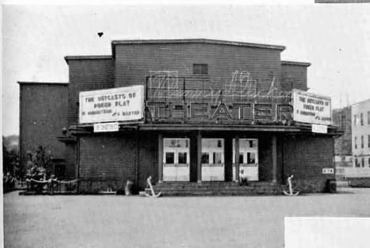
"Benny Decker" theatre at Fleet Activities.
