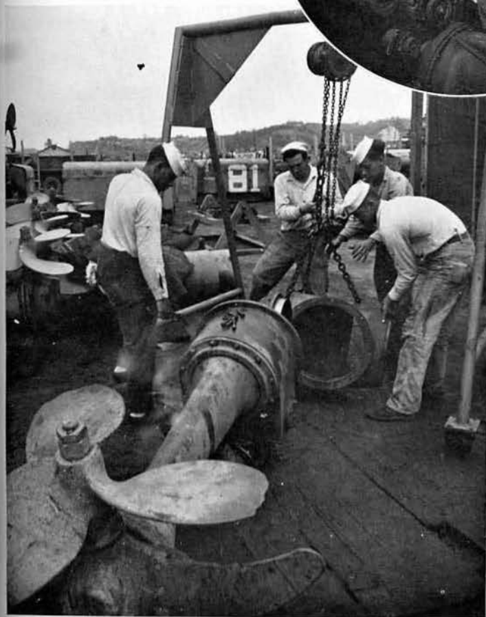
Crew repairing "tail section".
