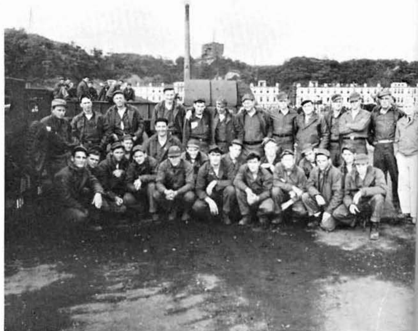
Right: LT RAHM and Pontoon Construction Crew in Yokosuka in the early days of the Korean conflict.
