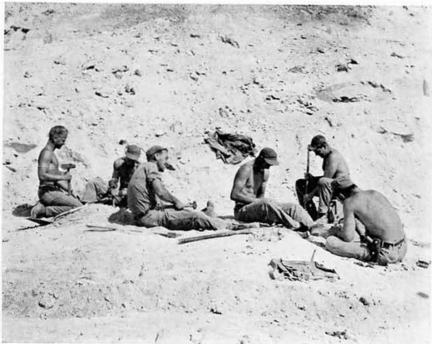
Drilled holes are loaded with TNT.
