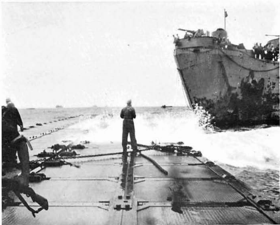
LST comes in as a breaker strikes the causeway.
