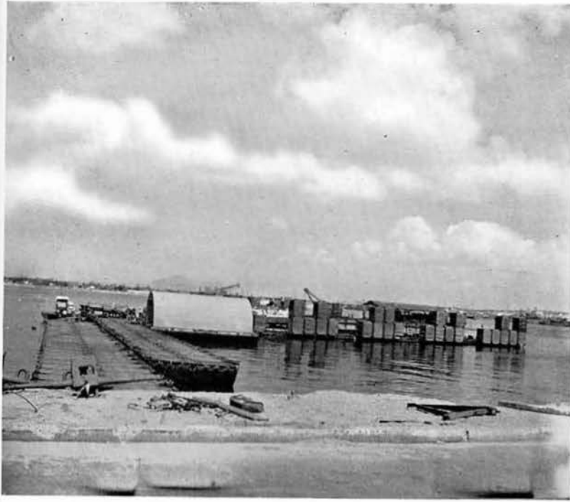
Pontoon Pier and Dock at Coronado.
