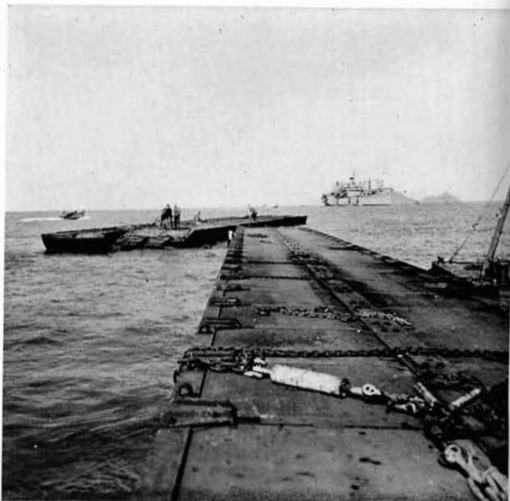
Joining causeway sections.
