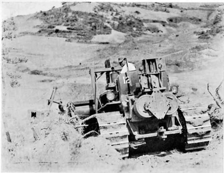
D-8 bulldozer working on a down-hill grade.
