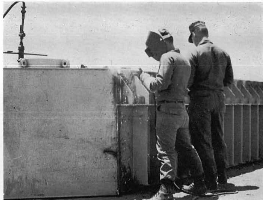
Steelworkers weld portions of a pontoon bridge.
