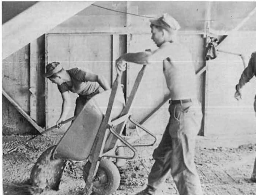
BUR2 THRONSON and BUR2 WHITTLE pour and level a concrete floor.
