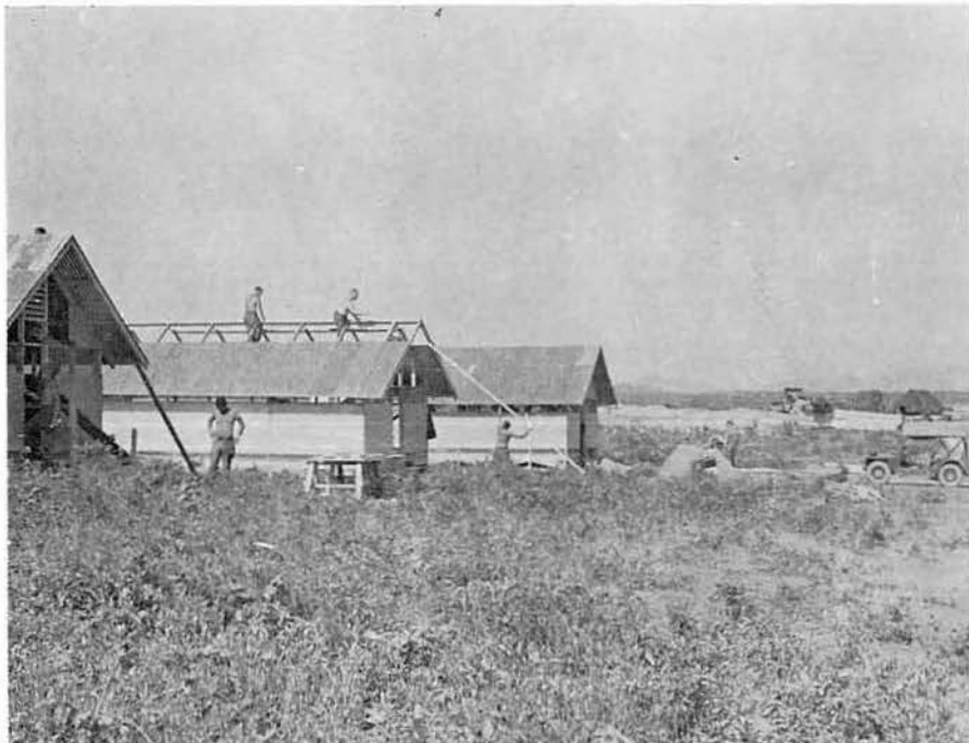
The first three huts near completion.
