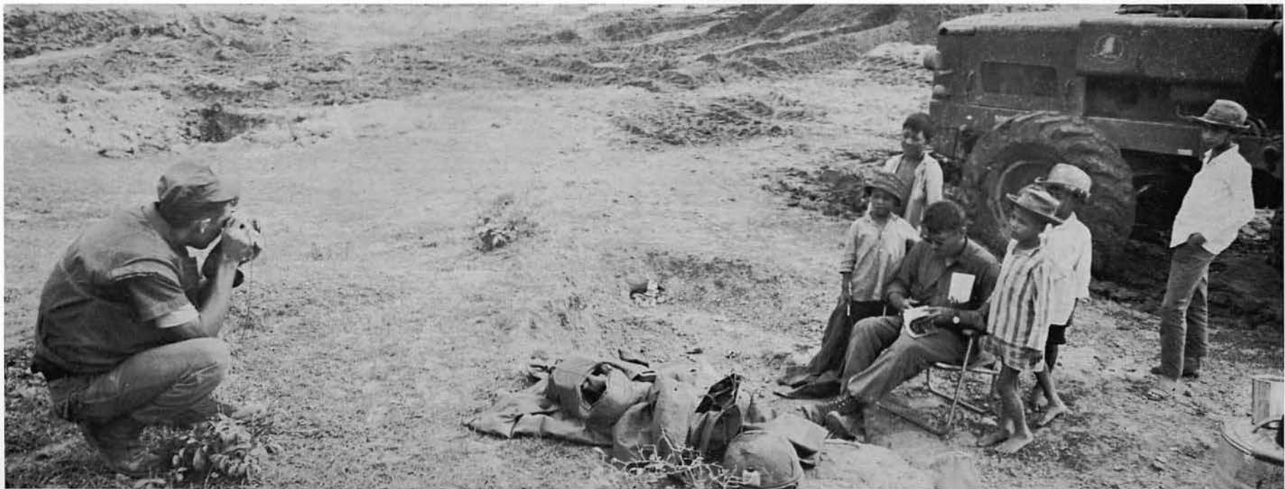
EAD2 MILLER , the Battalion photographer, is taking a photograph of EAD2 SHILLER and some of the local children who invariably gather around construction projects. The boys have brought a Vietnamese book for his inspection.
