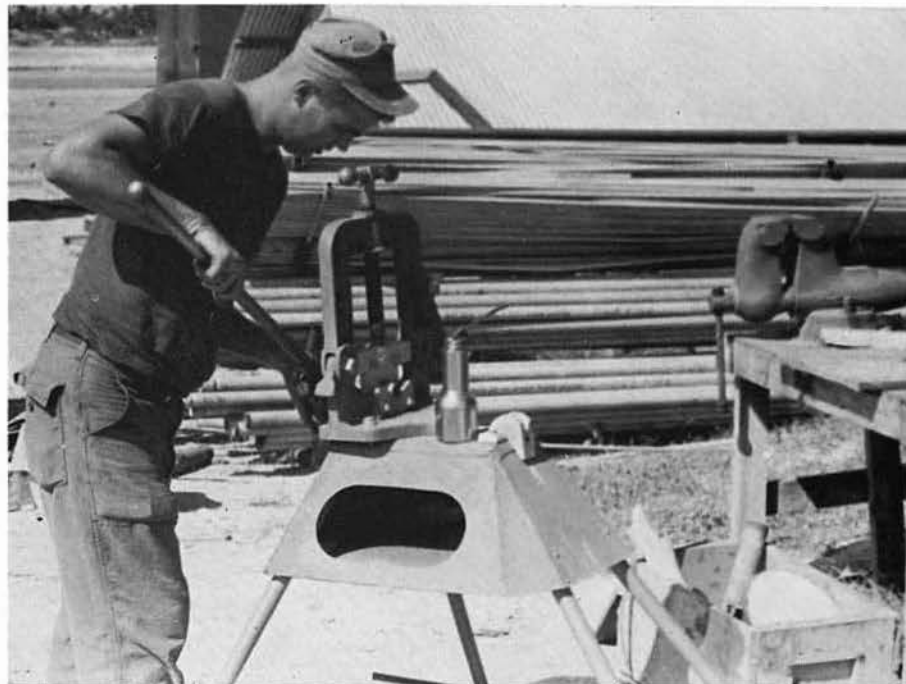
SWF2 OBACZKY cuts threads on a section of pipe.
