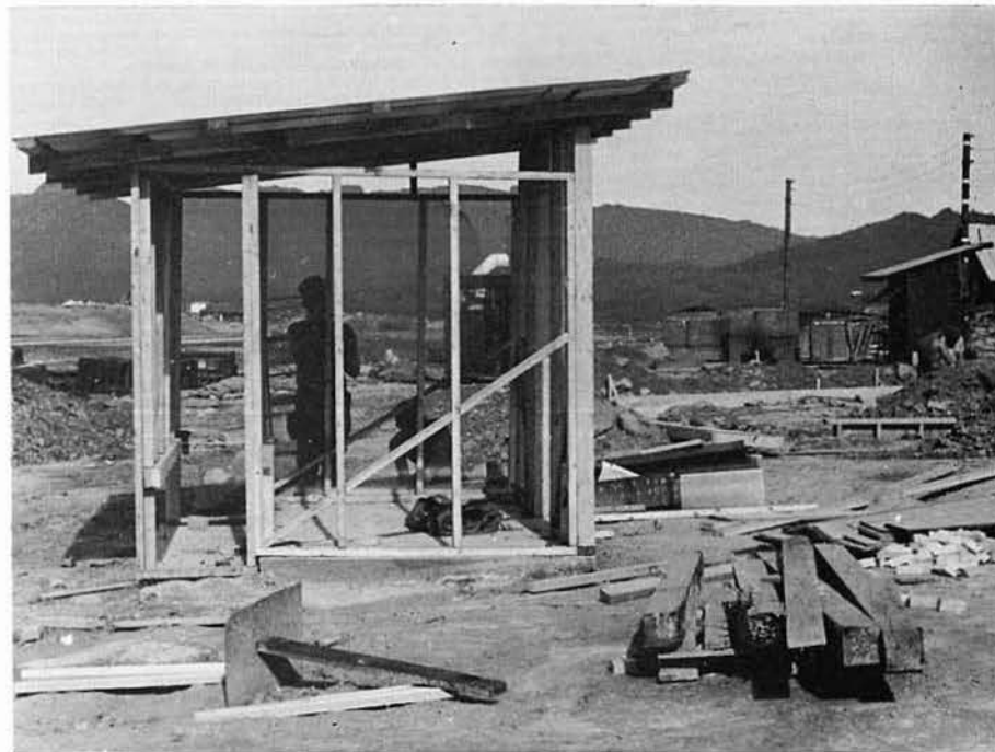
BUL2 GUESS and CN WALKER build a 4 hole burn out head.
