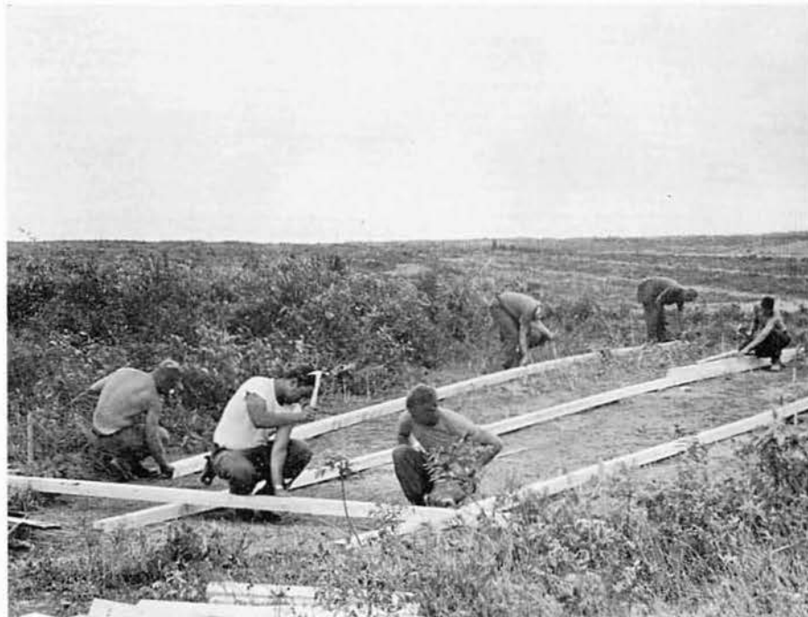
Builders assemble the girders and floor joists for a new hut.
