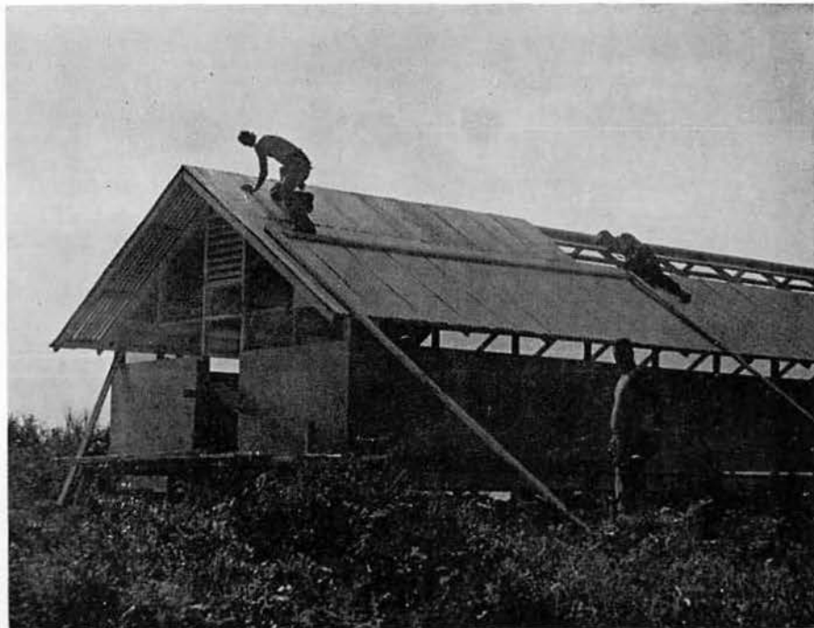
Steelworkers lay tin on a hut.
