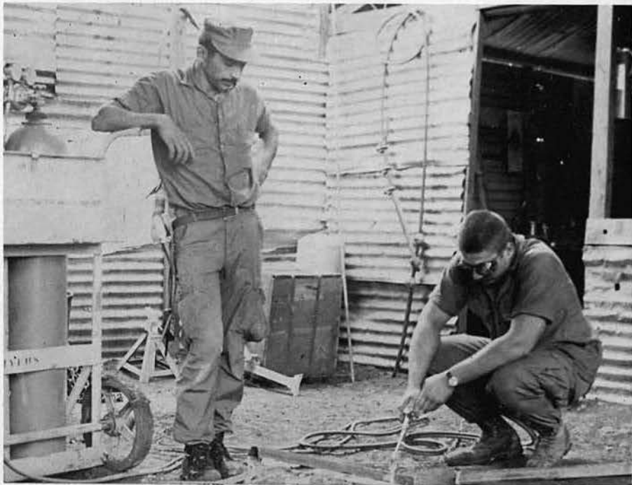
UTP2 RUIZ waits as CEWCN YOST cuts stakes with a torch.
