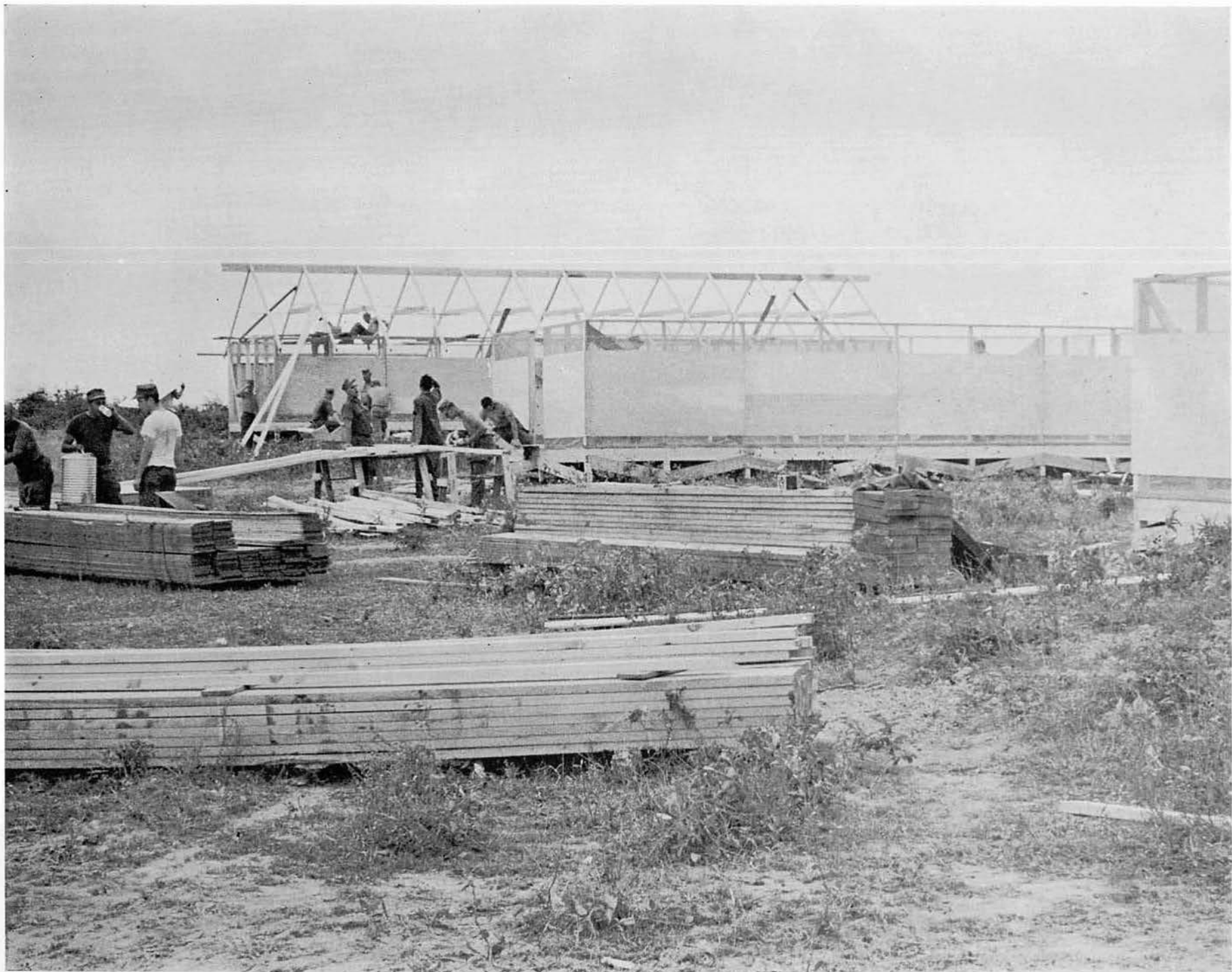
More and more huts going up.
