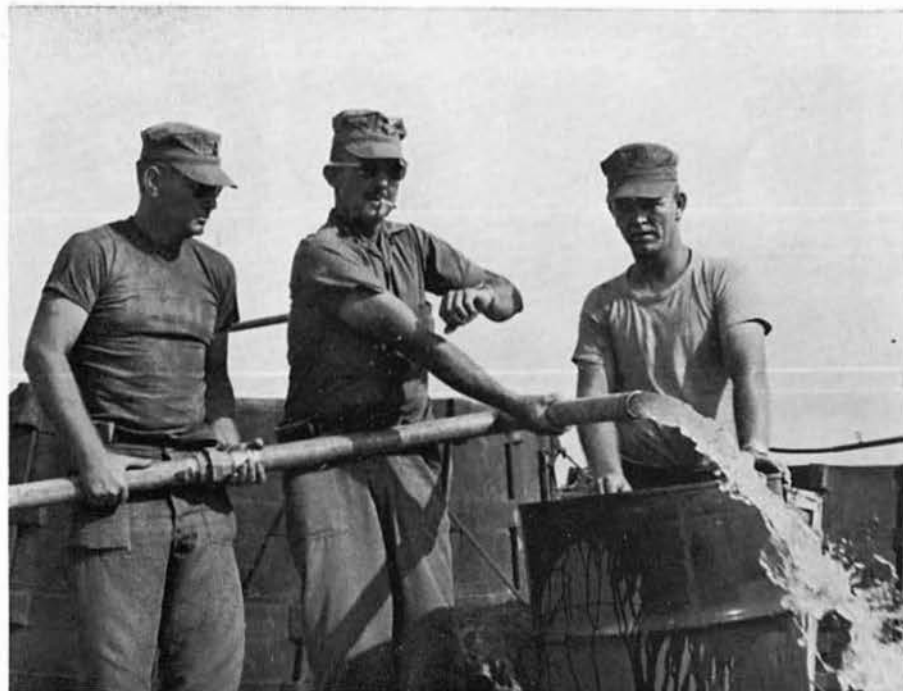
UTP2 WALTERS, UT1 ATTEBERRY and UT1 SMITH test the water flow from the new CBMU 301 well to determine gals/min.
