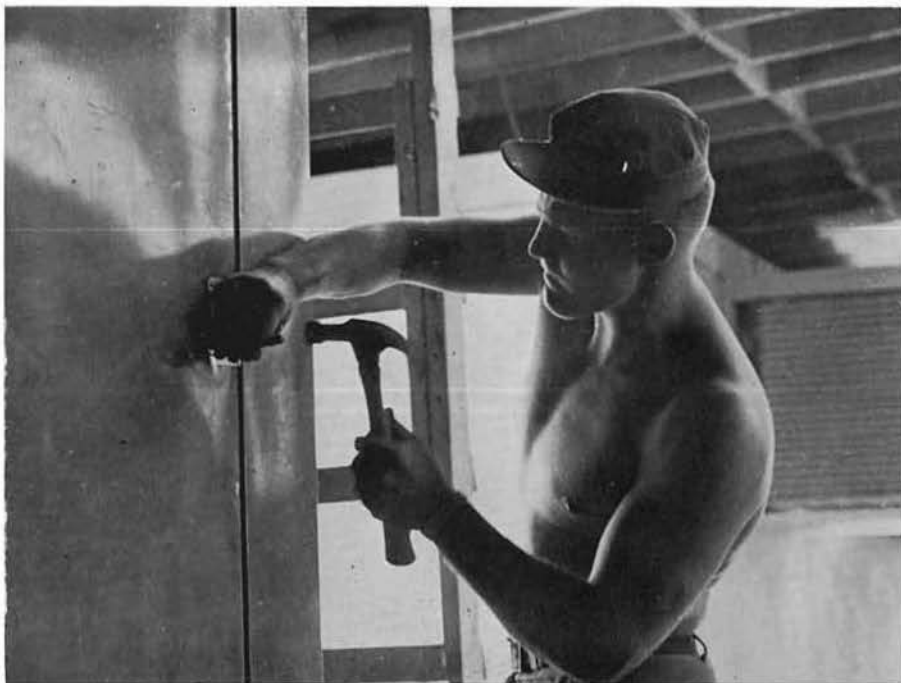
SWE2 ROBINS attaches a hinge to a metal door.
