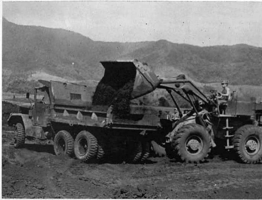
EON3 BROKAW loads dirt during the runway renovation project.
