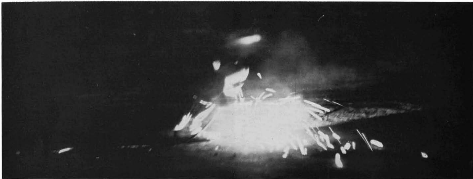
SWEEN REINIG, working on the night shift, cuts anchor bolts holding the matting down.
