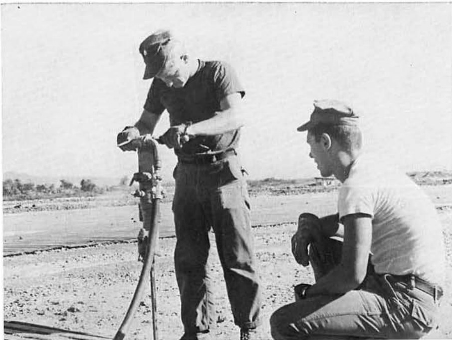
SWE2 JONAS drills a hole in the matting to set runway anchors as SWE2 PRATT observes.
