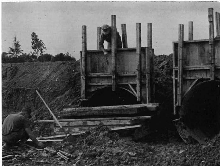
Culvert construction near the 9th Marines camp by 301 Seabees.
