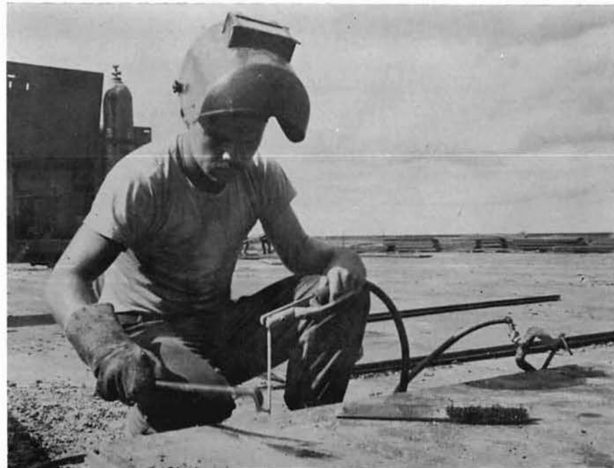
SWF2 REEK patches matting that has been damaged by enemy rockets.
