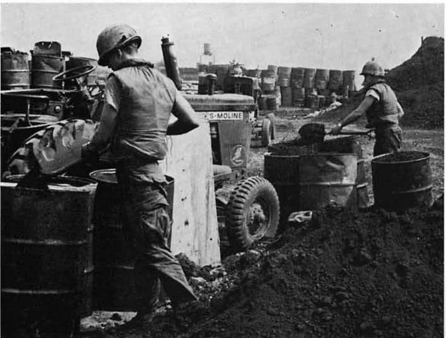
Two Seabees from Det. Bravo (Khe Sanh) fill 55 gallon barrels with dirt to be used as revetments.
