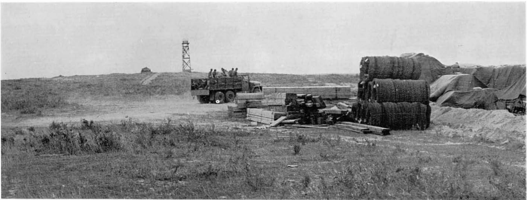
The Main Body campsite prior to beginning of construction.
