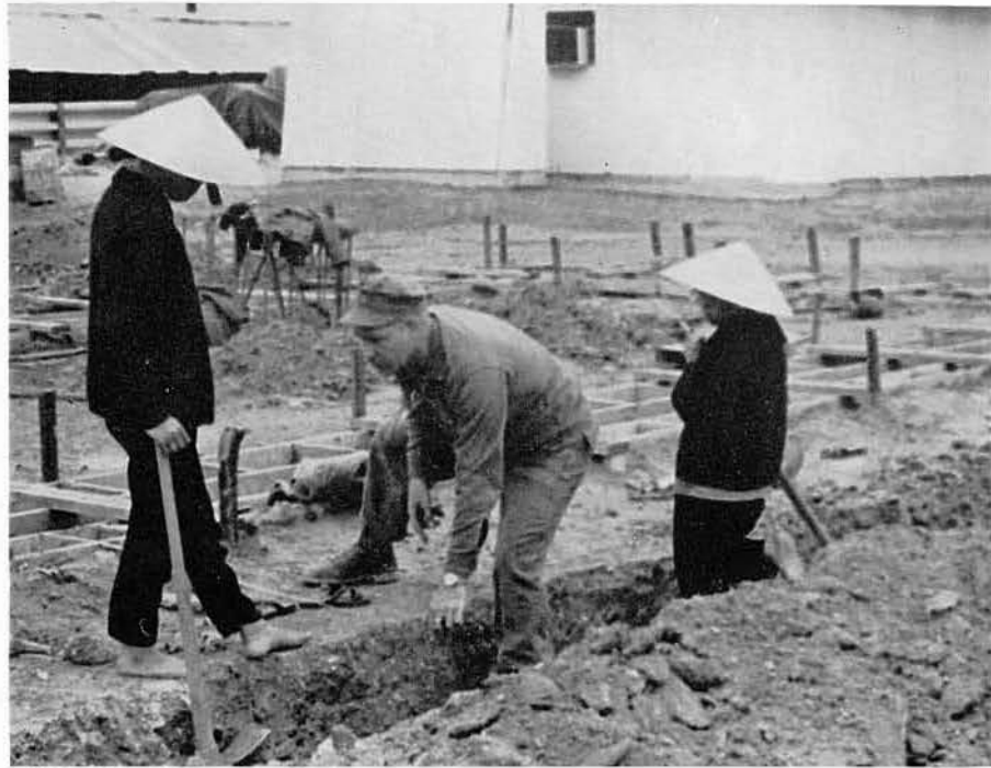
BUL2 WEBBER assists in laying the foundation with native workers.
