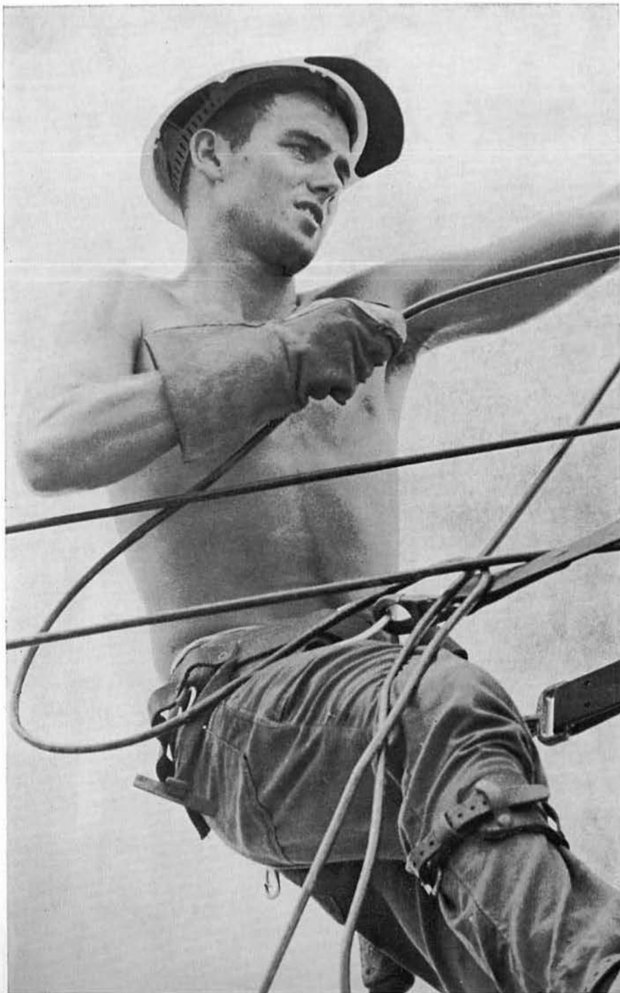
CEW3 MURRAY strings power lines to the camp 'hooches'.
