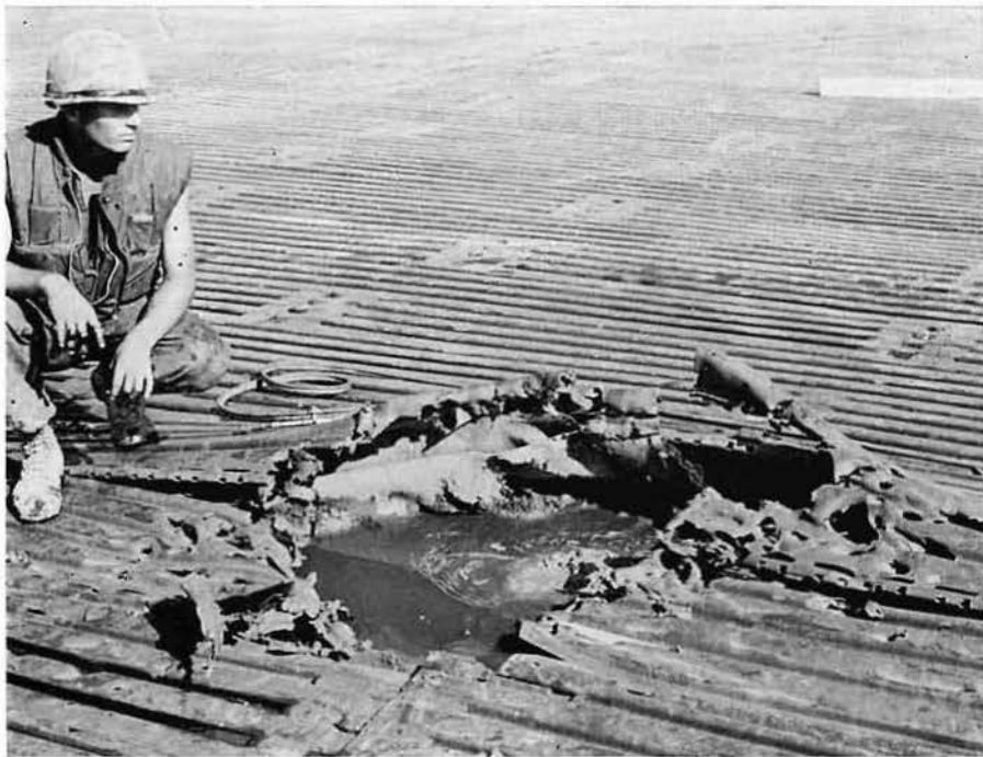
BUR2 CAPP5 surveys damage on the airstrip runway apron caused by a rocket.
