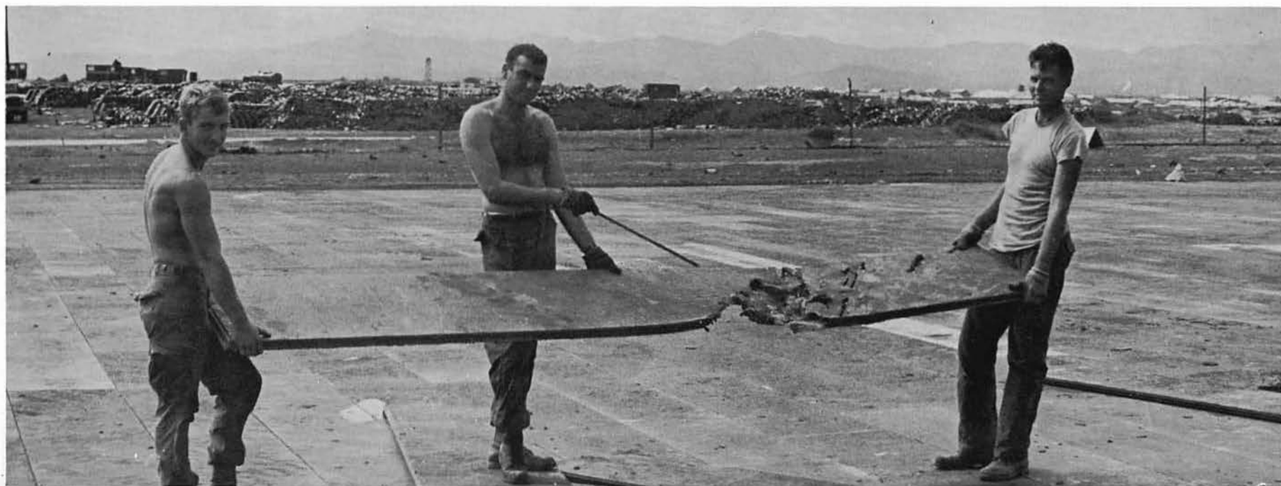
CN WILSON, SWE3 BLUME and SWF3 CROW display a damaged section of runway matting after an attack in September, 1967.
