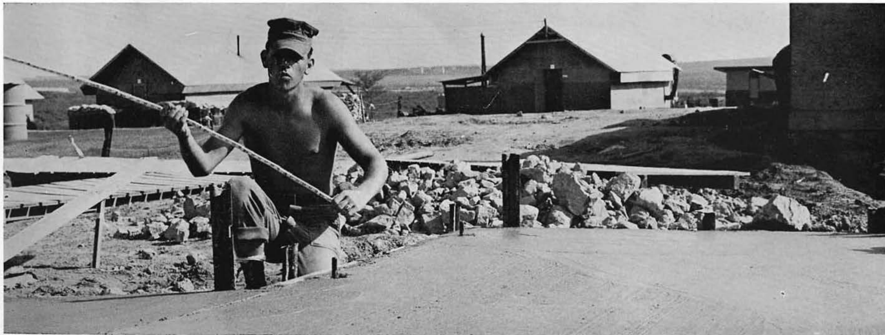
BUL3 WARD checks out the CBMU 301 sick bay floor slab.
