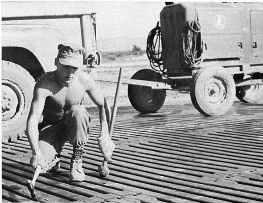
SWE2 ECCLESTON repairs a section of the runway.
