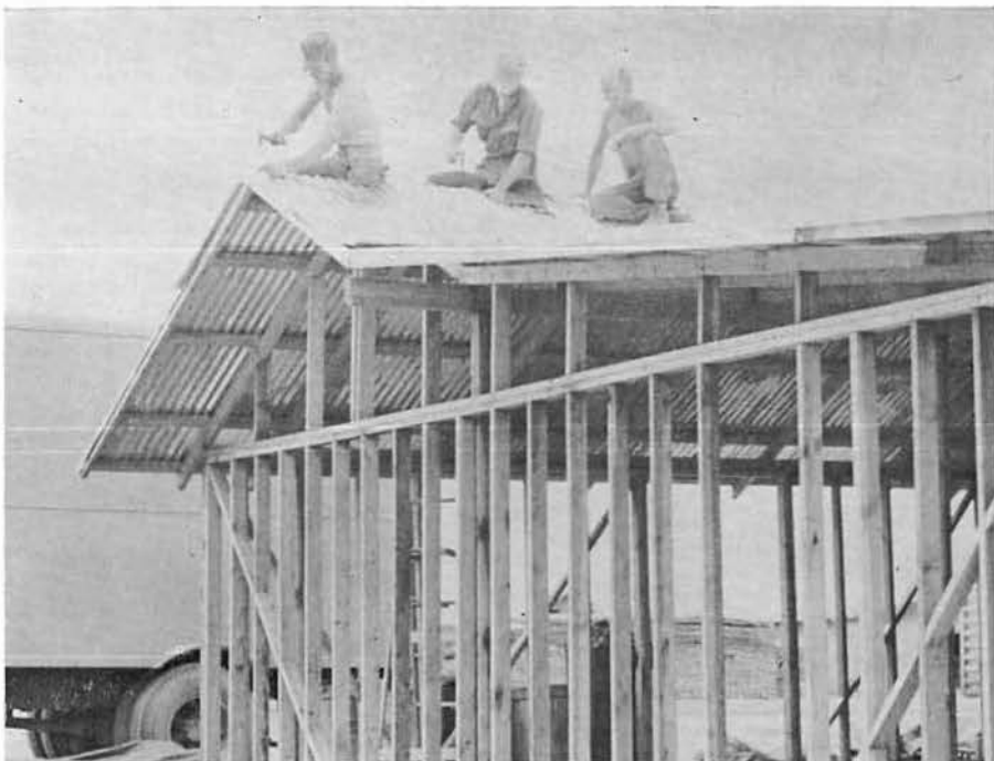
A new building for graves registration built by Charlie Company.
