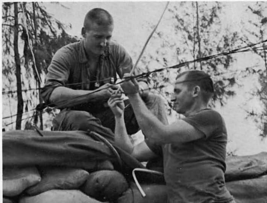
CEP2 FOGLE and CEW3 RICHMOND splice wire from a hut.
