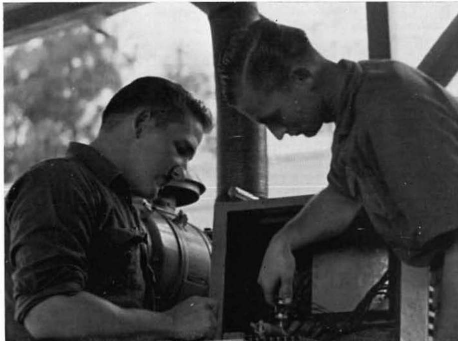
CEP2 FOGLE and CEW3 RICHMOND perform preventive maintenance on the electrical system of a generator.
