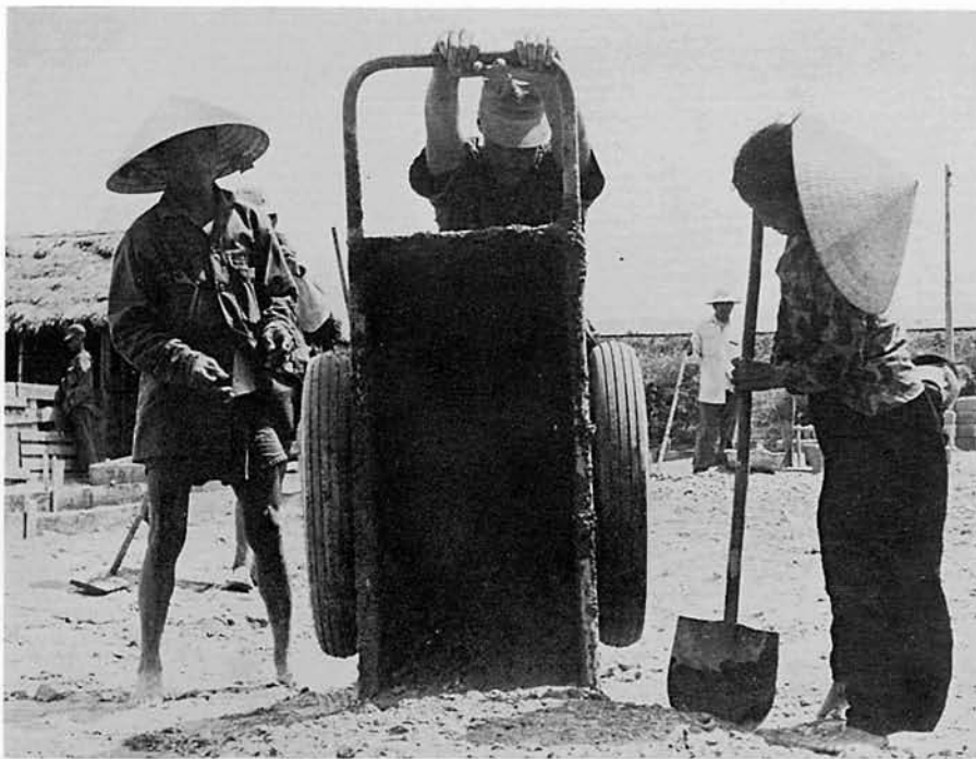
BUR2 CAPPs shows the natives how to use the "Georgia Buggy" in a civic action project at the village of Dai An.
