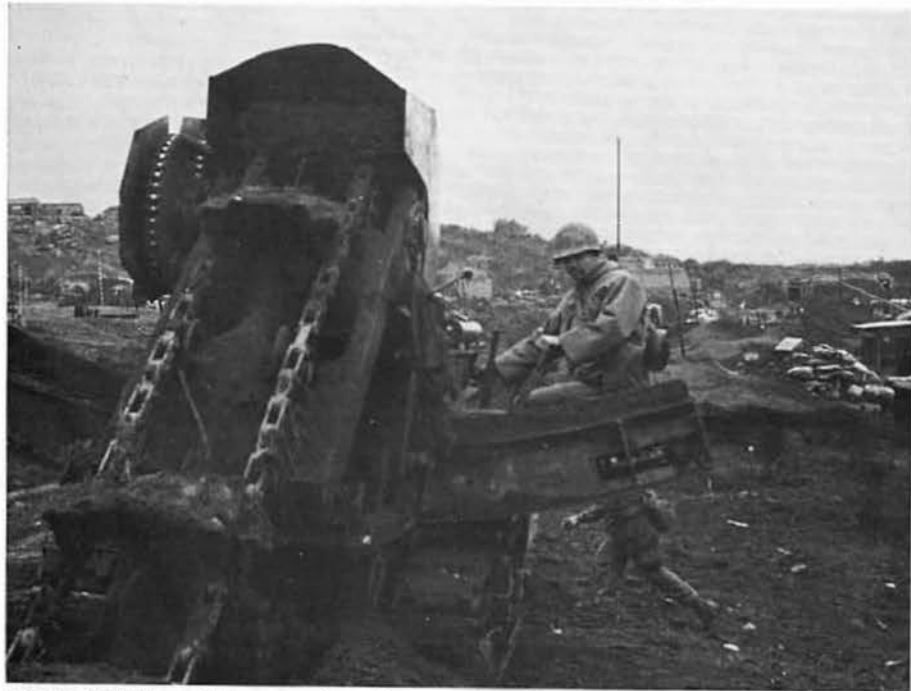
EON2 BONE and his trencher dig trenches for the Marines at Con Thien.
