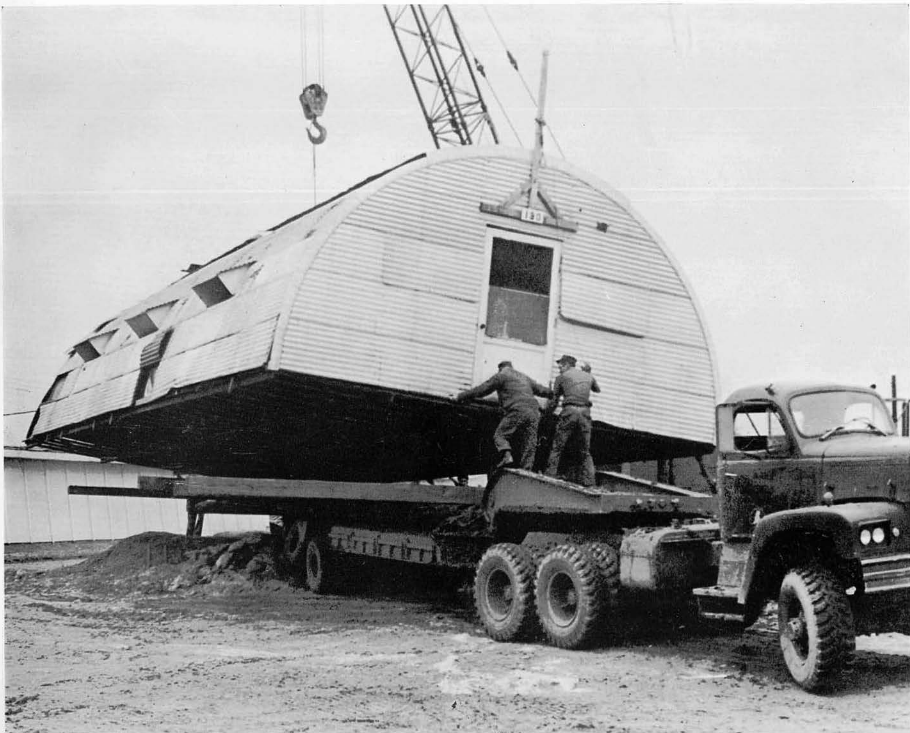
The lowboy trailer goes into the house moving business. This Quonset hut from the Air Force is proposed for the Officer's and Chief's club.
