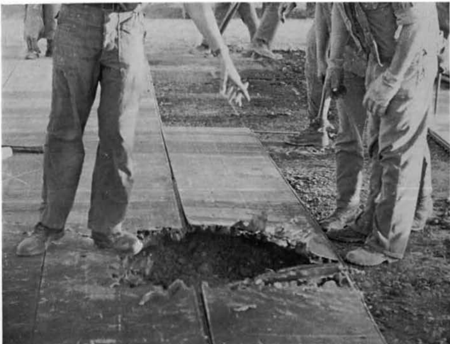
A 122 mm rocket scores a direct hit on Dong-Ha runway. Repairs are usually completed within a few hours.
