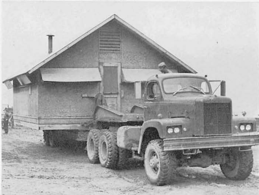
After a short tenure at the new location it was converted to the Chiefs living quarters.
