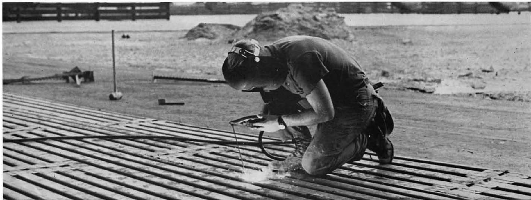
CN WILSON uses a cutting torch to repair the runway.
