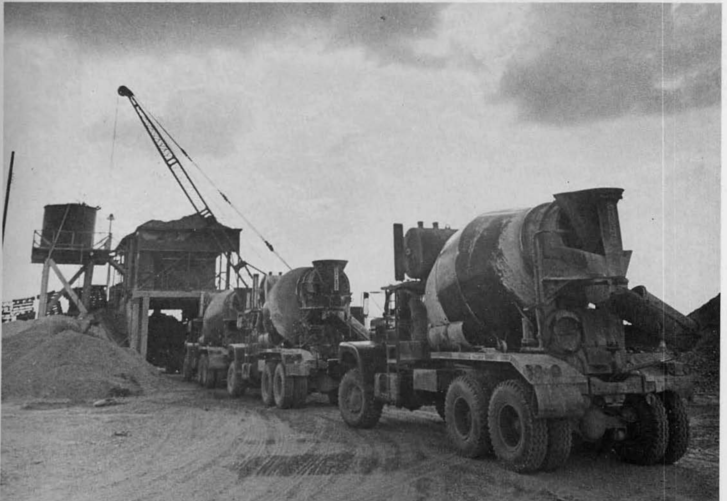
Below: Transportation's transitmixers line up for a load of concrete.
