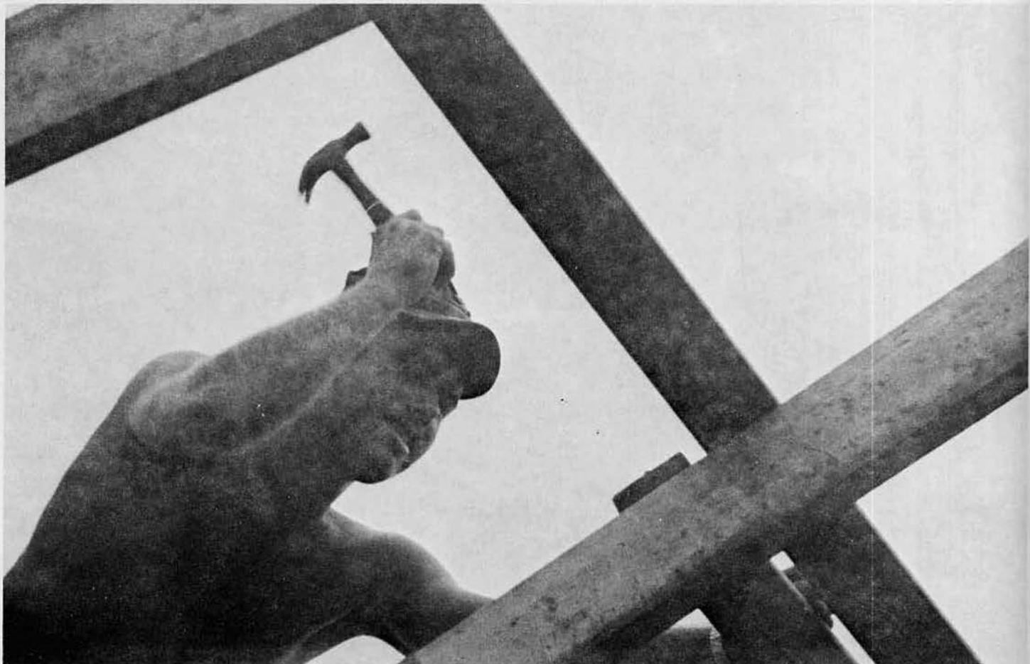
Below: BU3 C.L. Coudran works on the new firehouse.
