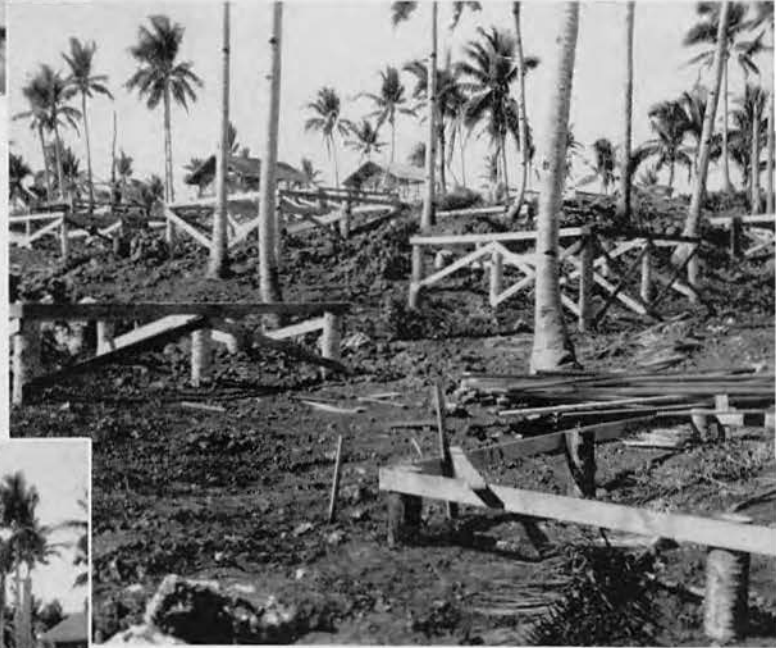
FOUNDATIONS ARE MADE PRIOR TO MOVING
