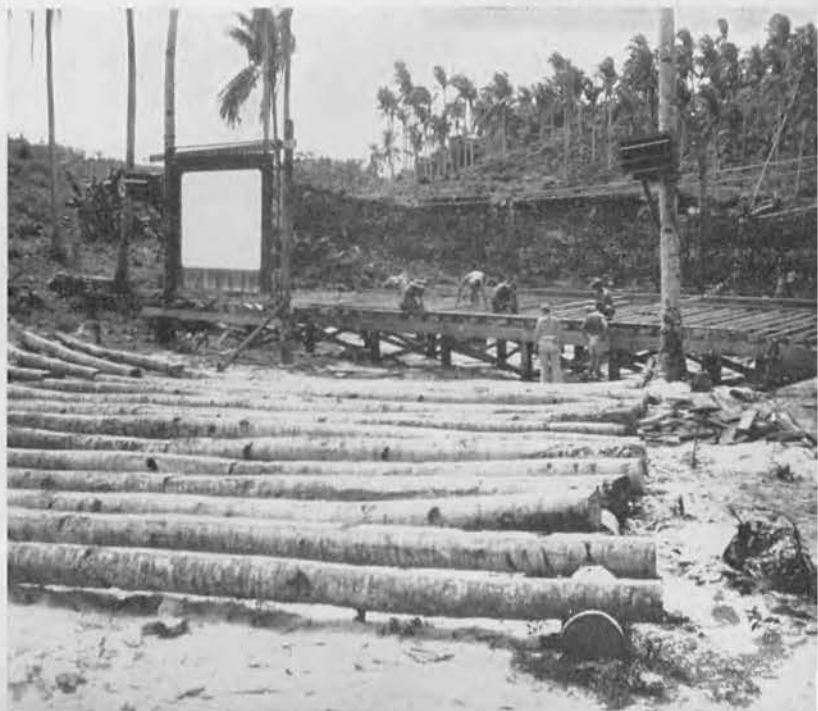
BUILDING THE STAGE
