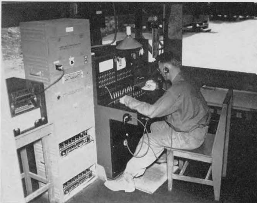
ORIAN AT THE SWITCHBOARD
