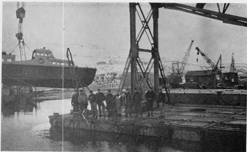
Heavy lift crane on pontoon barge picking up a "cinch" load.
