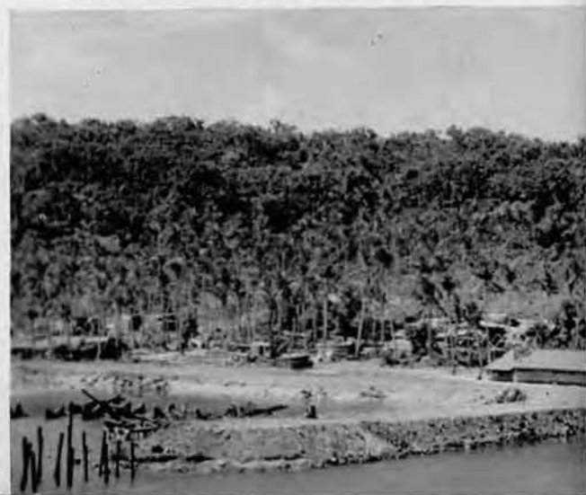
General view, from docks, of our cargo office and rigging lofts before improvements.
