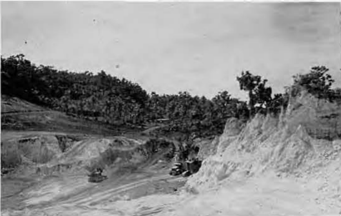
Digging in coral pits for fill and road surfacing.
