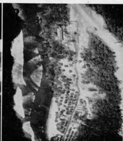
Left: 1. Hacked out of dense jungle growth and surfaced with sand from the beach our men made a civilized camp out of this savage country. 2. Due to the extremely porous nature of this coral island well drilling was out of the question. Brackish lake at top of picture furnished water for our condensers which turned out pure water for drinking, cooking and washing.
