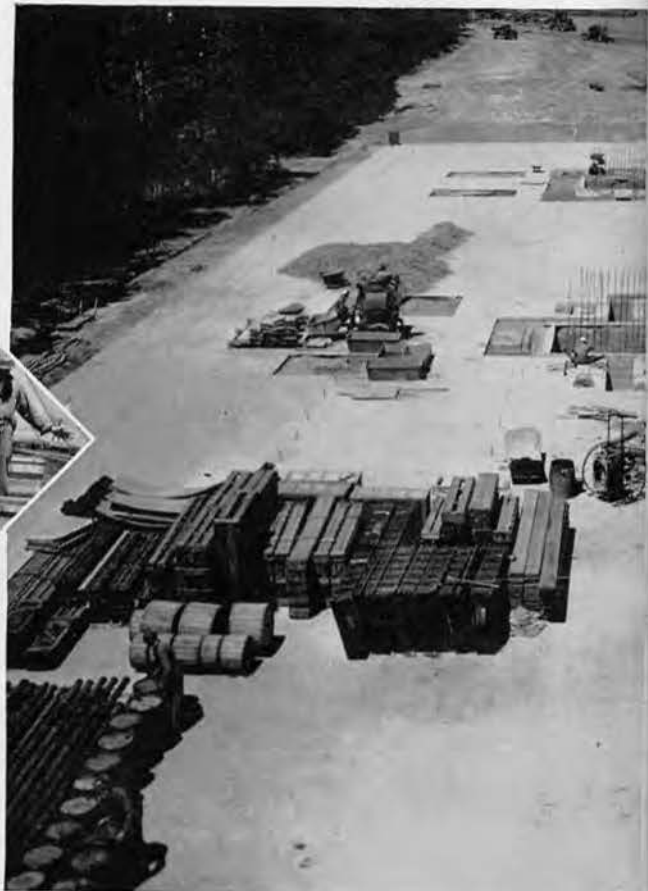
Looking aft along newly laid keel of U.S.S. "Seabee." Foreground shows piles of training cargo which was loaded and unloaded thousands of times yet never left port.
