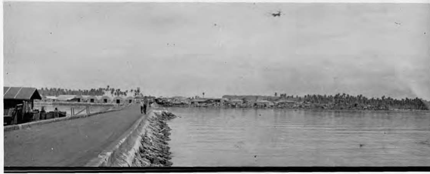
Jetty at Guiuan, Samar.
