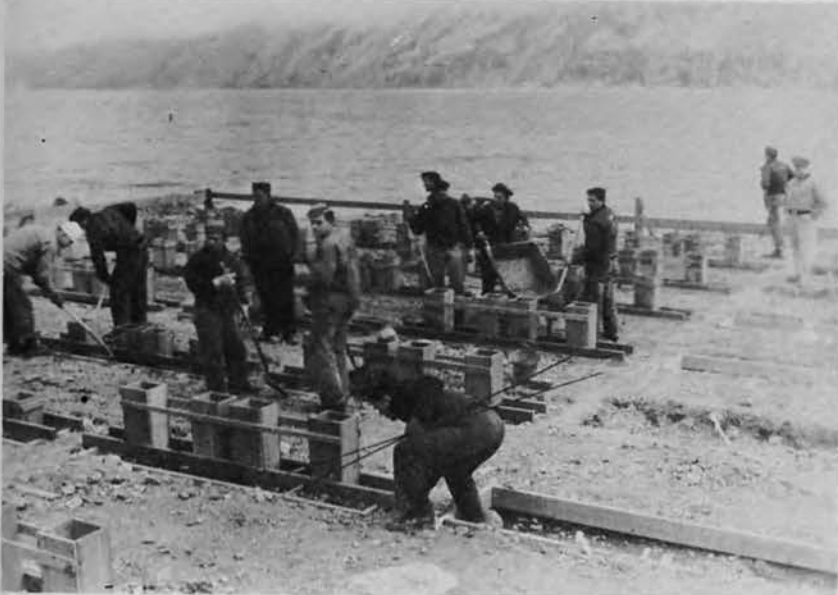
Drum Storage—Preparing Forms for Concrete
