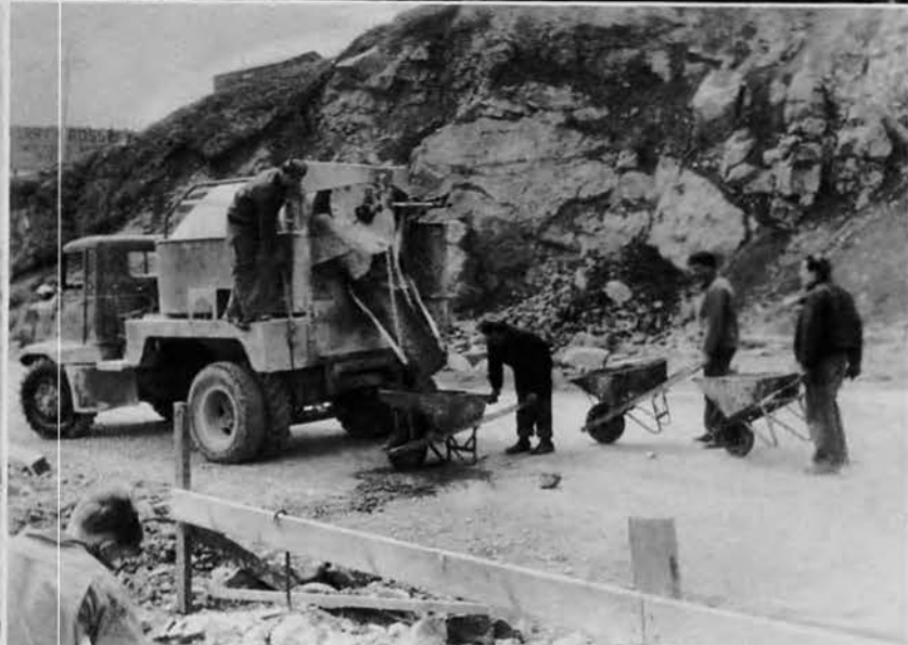
Concrete Mixer Truck discharging
