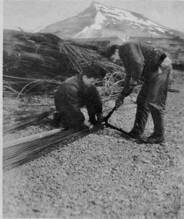
Cutting re- inforcing Steel
