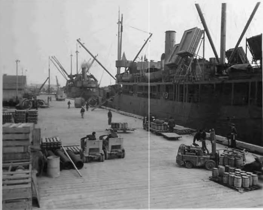
Temporary Pier Dock #1
