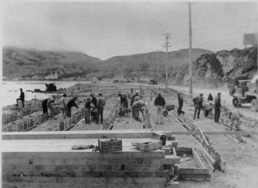
Pouring Concrete at the Drum Storage
