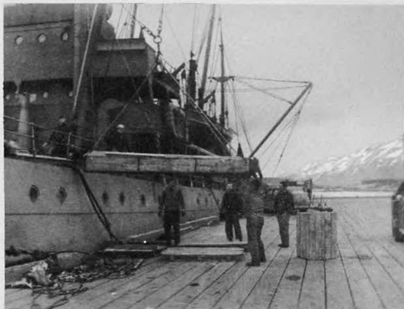
Discharging Cargo from Ship
