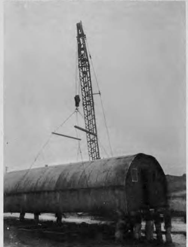
Dropping a Quonset Hut in place
