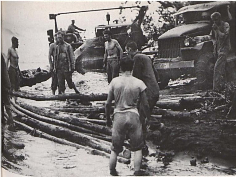
Trees and logs are put in place by Marines and SeaBees for a bridge across a jungle stream on the road to the Cape Gloucester airfield, New Britain Island.
