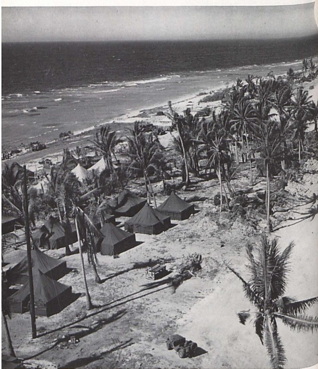
One of the major tasks of the Navy's SeaBees in the Pacific was improving captured Japanese airfields. Following the fall of Eniwetok in February 1944, they promptly began enlarging and improving the airstrip on the atoll. Tents in the palm grove house the aircrewmembers.
