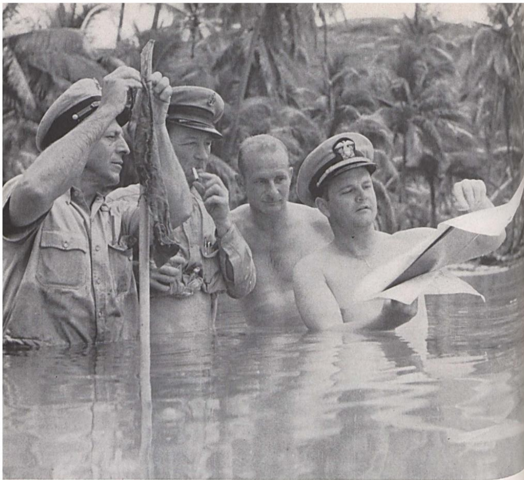
In spite of all the good-natured chaffing they received from the Navy and the Marine Corps, the SeaBees had what it took. Unperturbed by minor distractions, these men are well on the way to being up to their necks in work as they discuss plans and details for seaplane runway ramps.
