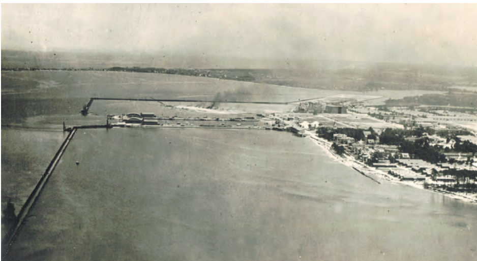
N.A.S. Norfolk in 1918 was a small, but growing operation. In the upper right hand corner can be seen the large hanger meant for dirigibles and in the center are the Government Piers left over from the 1907 Jamestown Exposition. The walls out in the water are the beginnings of the reclaiming operation. Eventually, the entire area inside the walls would be filled in and used to expand the air station and the Operating Base. (HRNM photo)
