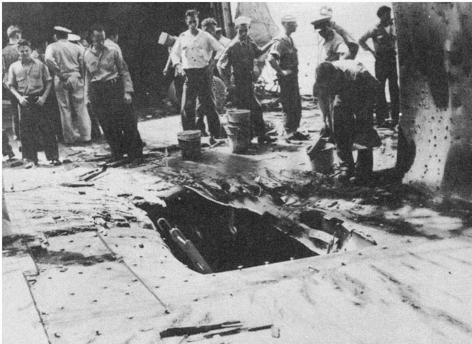
Hole in deck of Chester caused by bomb hit on February 1, 1943
