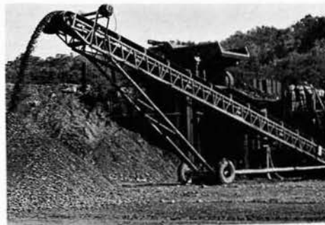
"Rock Crusher" in operation at quarry. From boulders to pebbles in minutes
