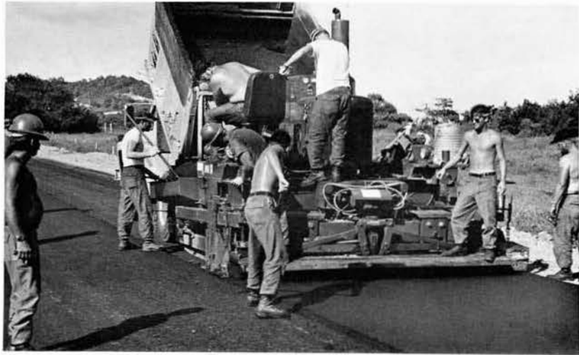
Alfa Company road building crew laying asphalt on Leyte-Boxer Dr.
