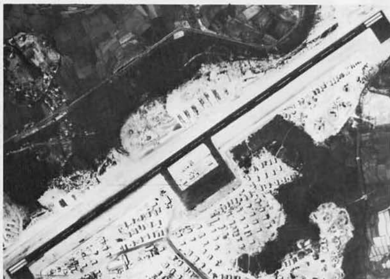
A cloud's view of the job site
