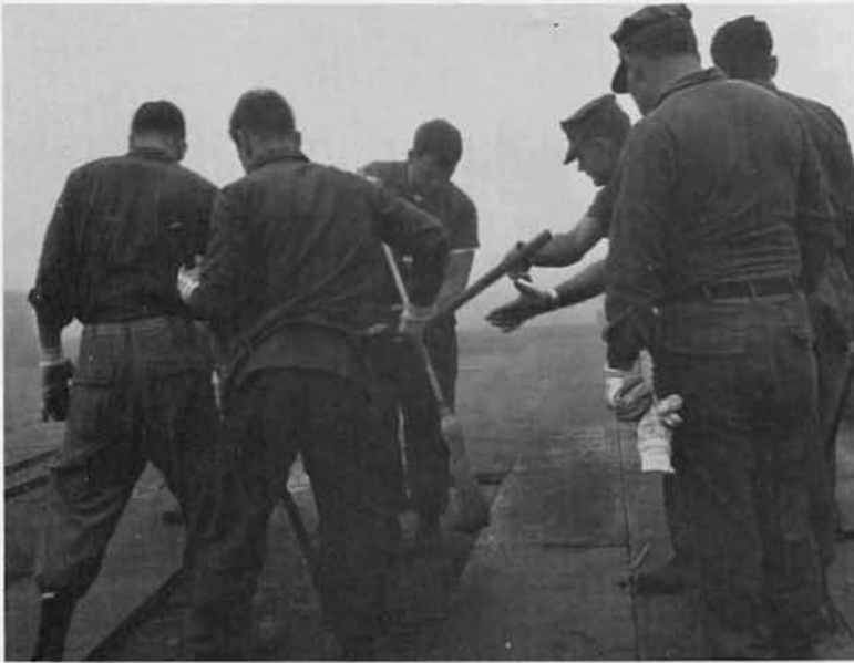
Laying of runway matting
