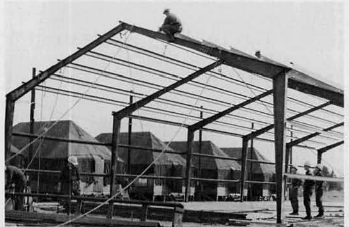
Butler construction training
