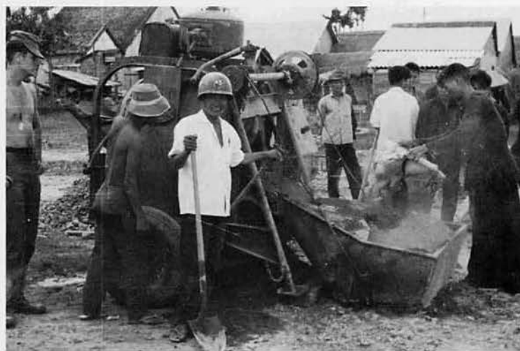
CMA2 James supervises cement mixing
