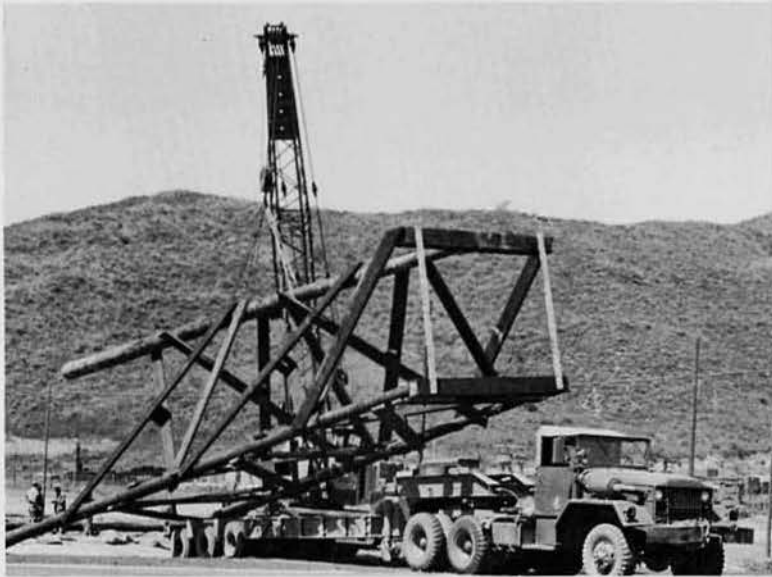
Completed towers were hauled by truck. . .
