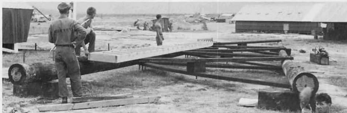
Tower construction at An Hoa
