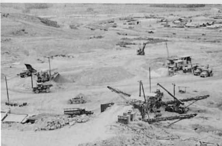
Crusher and batch plant.
