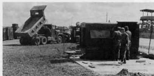
Generator prepared for use.
