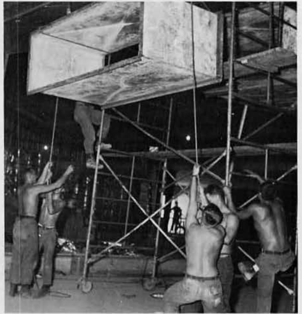
Ductwork goes in!
