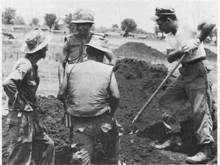
Men filling sandbags?
