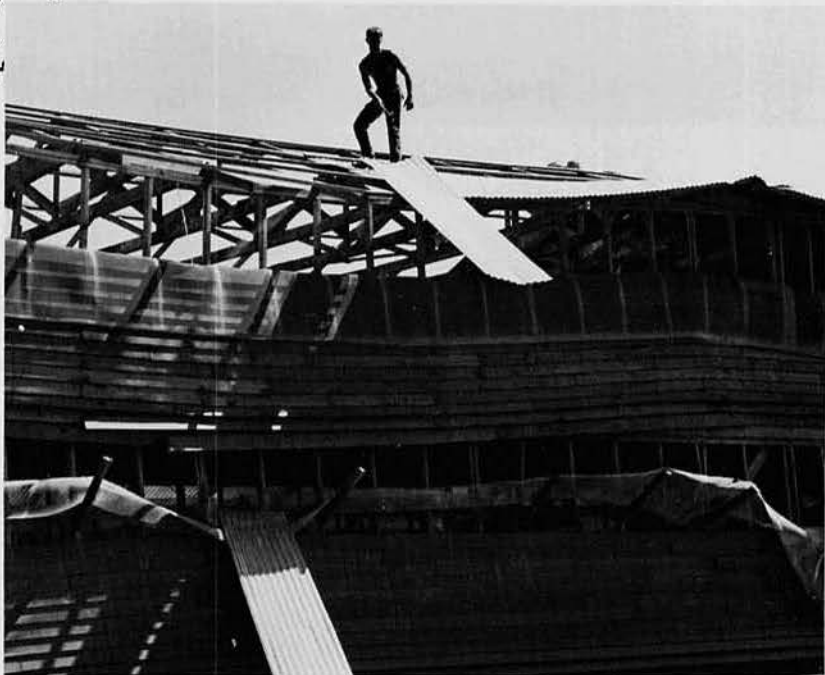
Rocket damage repair work
