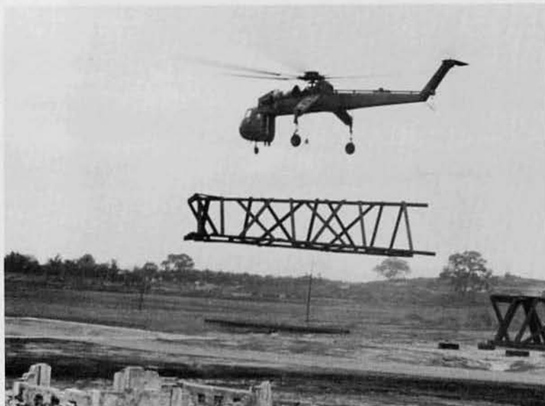
. . . and by aerial crane
