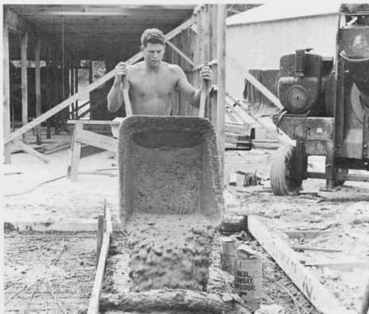
Pouring the concrete deck
