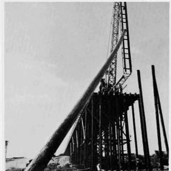
Piling goes in place
