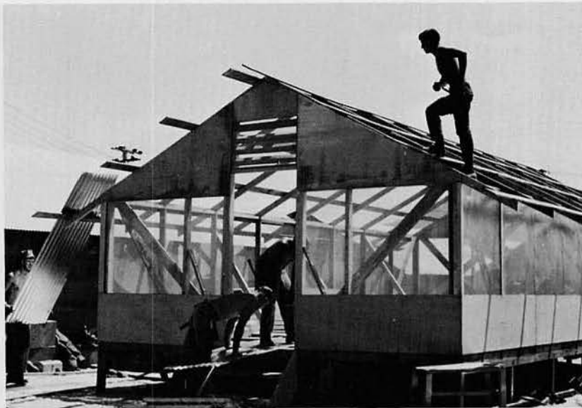
Another strongback going up!
