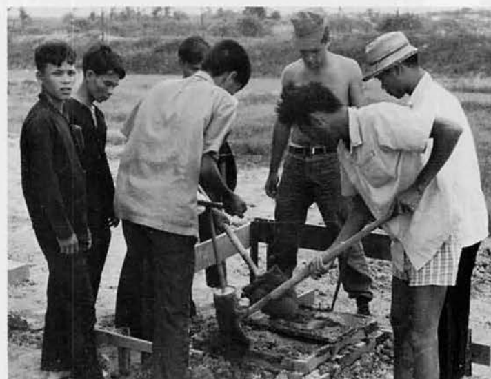
Pouring footer at Chieu Hoi Center
