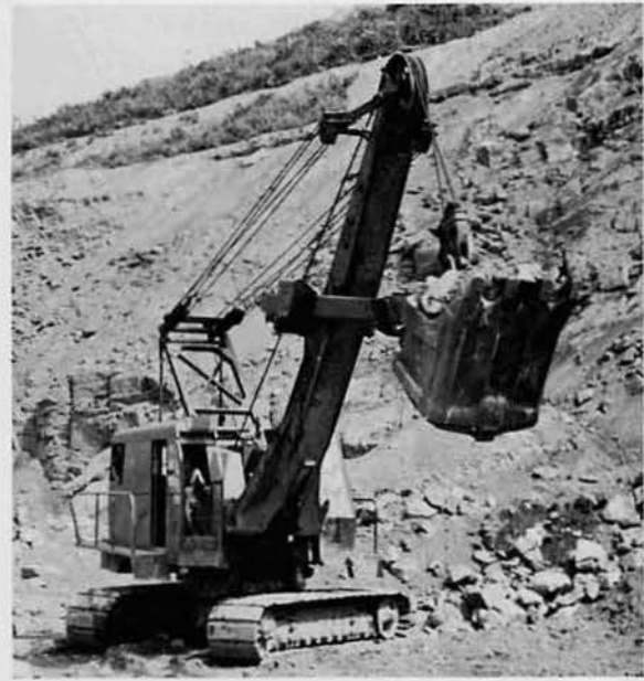
Picking up blasted rock.
