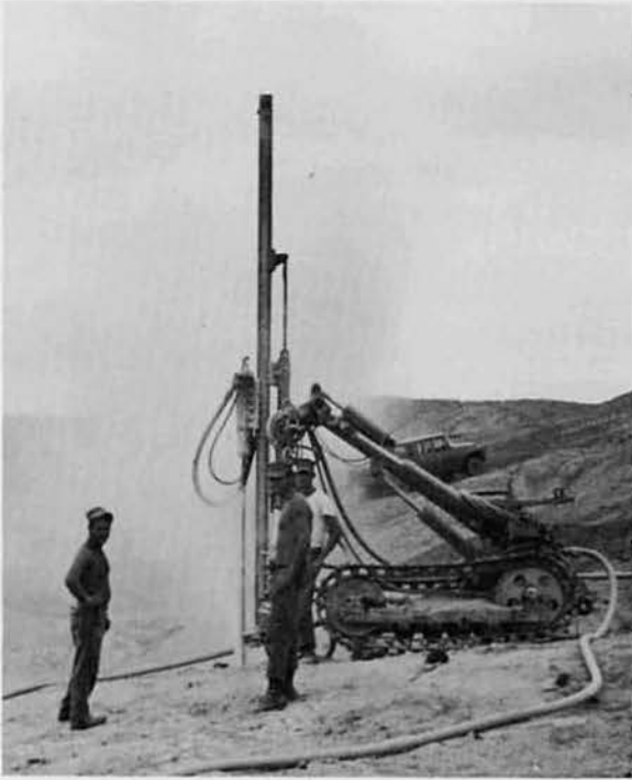
Preparing the blast.
