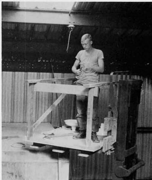
CEW2 Fox installs lighting
