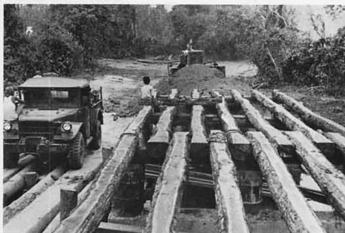
62' timber bridge over Lam Plai Mat
