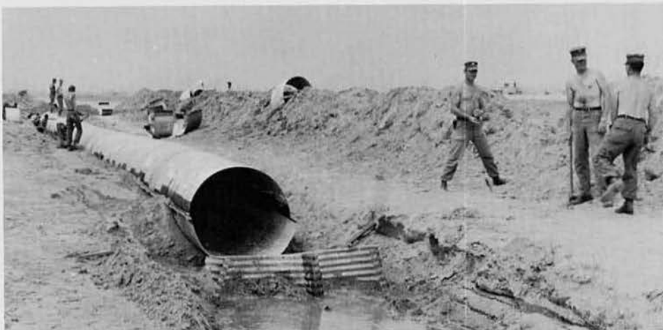
Drainage ditch at Danang Airbase
