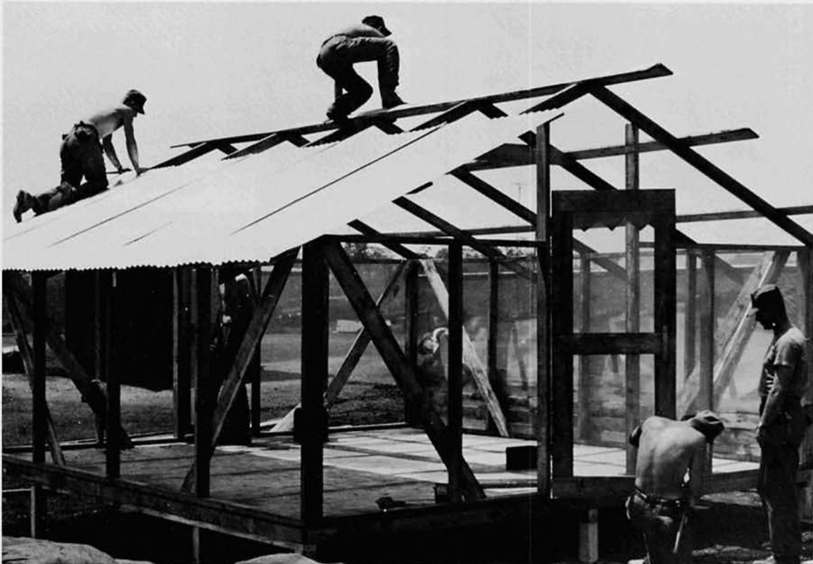
One of the many strongbacks that were built.
