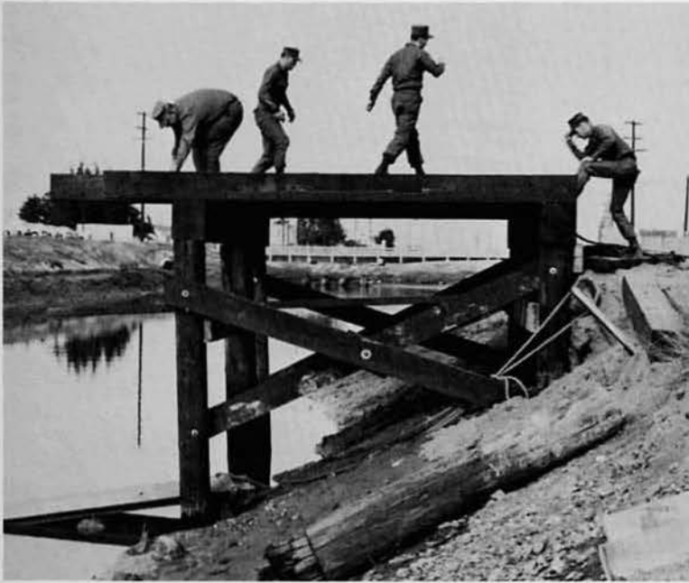
On the job training at Port Hueneme
