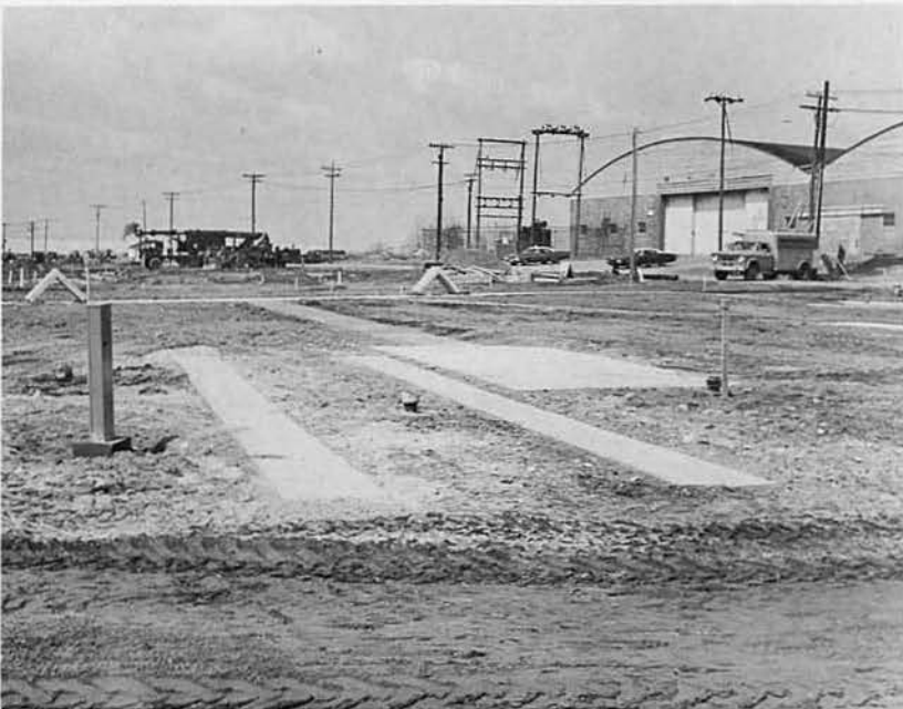
Finally another pad was completed.
