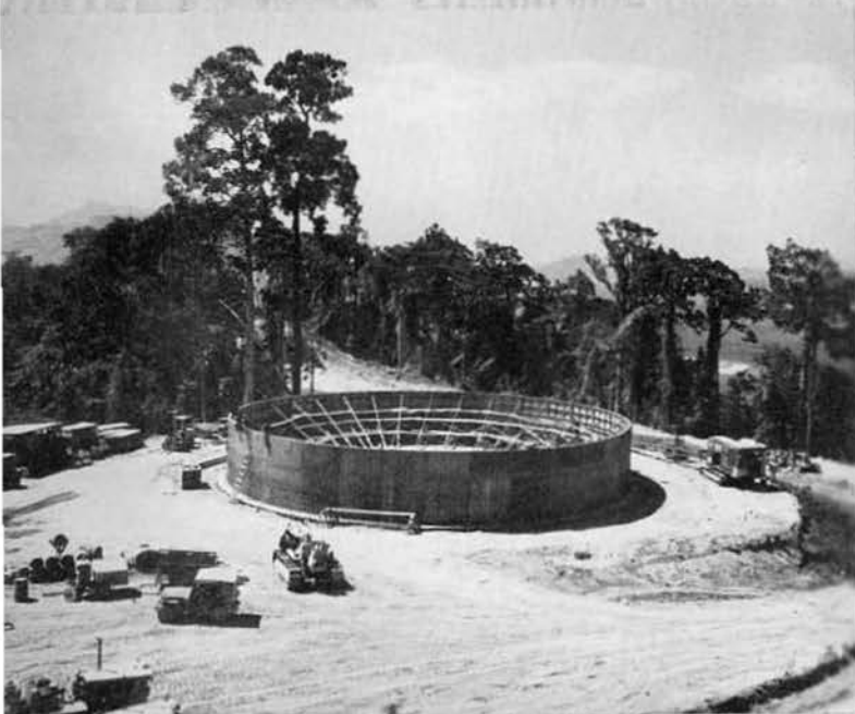
● HIGH LEVEL RESERVOIR GRAVEL-SAND HOPPER ●
