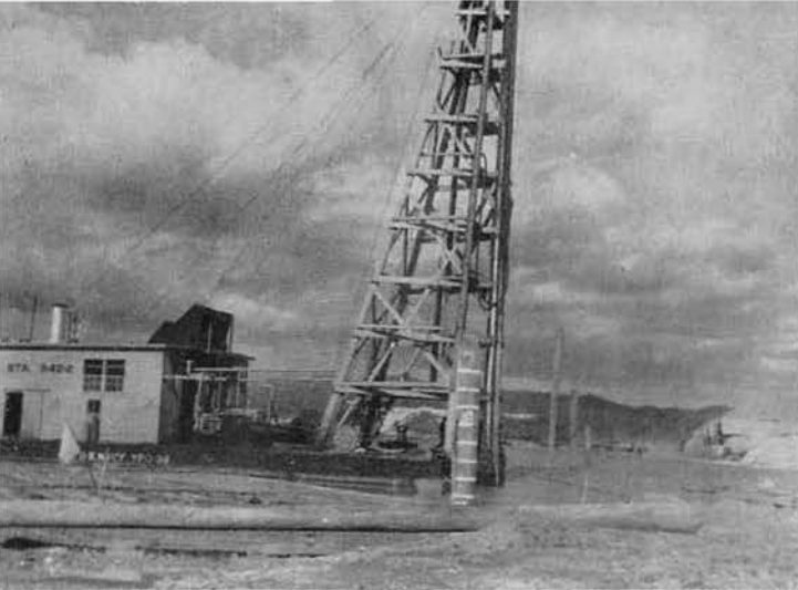
● YARD PILE DRIVER (YPD-38)
