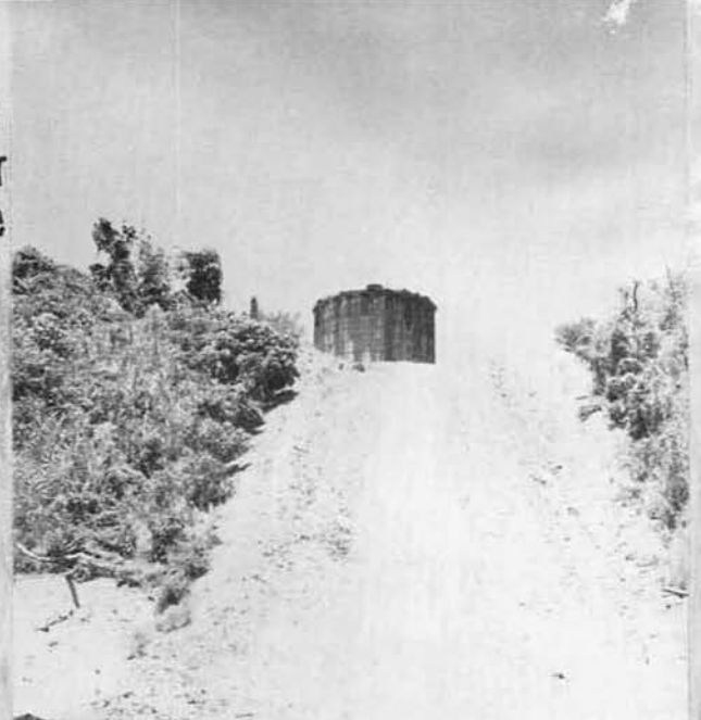
MOUNT MARITAN STORAGE TANK ●
