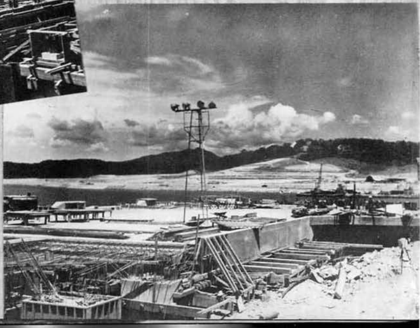
CARRIER WHARF CONSTRUCTION
