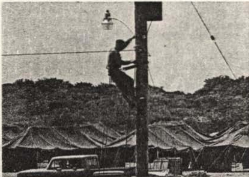
FOUR rigging street lights at Orote Point.
