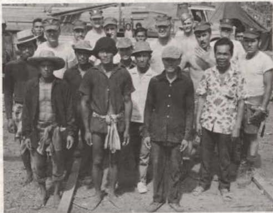
Builders from Delta Company and some of the Thai carpenters.
