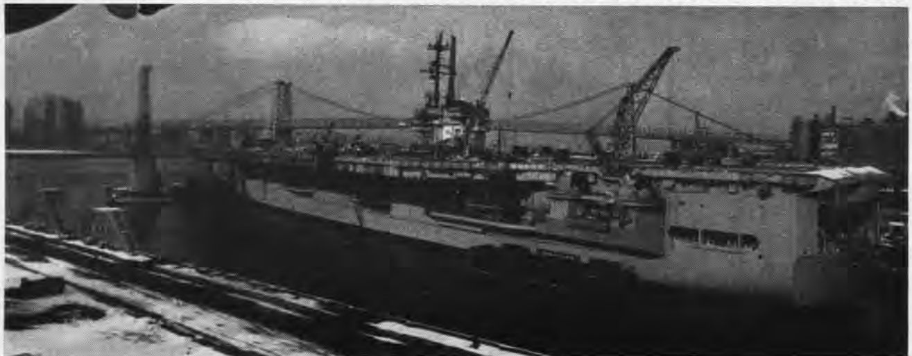
WORKMEN READY THE USS INDEPENDENCE FOR HER COMMISSIONING AND EARLY OPERATIONAL DEPLOYMENT WITH THE ACTIVE FLEET
