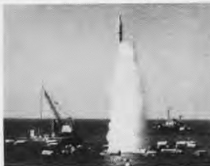
TEST POLARIS UNDERWATER LAUNCH GEAR
