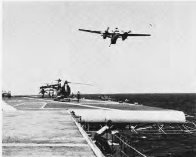
VS-34 52F, MAD BOOM AND RADOME EXTENDED, MAKES FLY-BY
