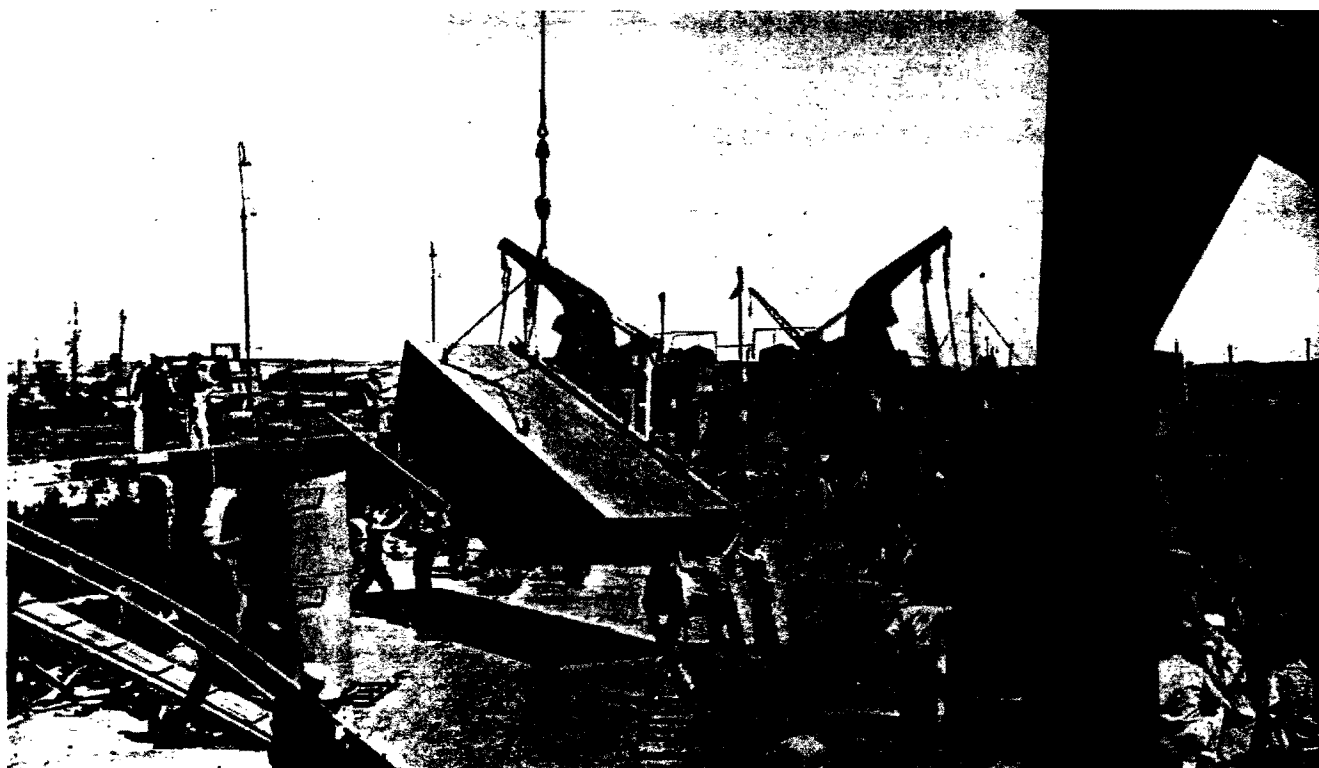
Unloading and Salvage Operations after Dropping Anchor at Advance Base
