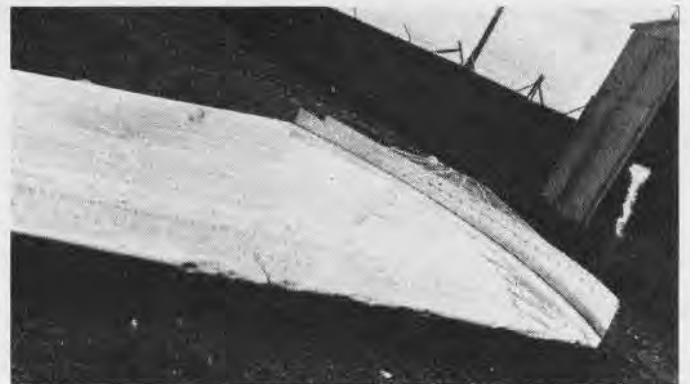
HAIL CAUSED THIS DAMAGE TO DC-2 WING IN LESS THAN THREE MINUTES
