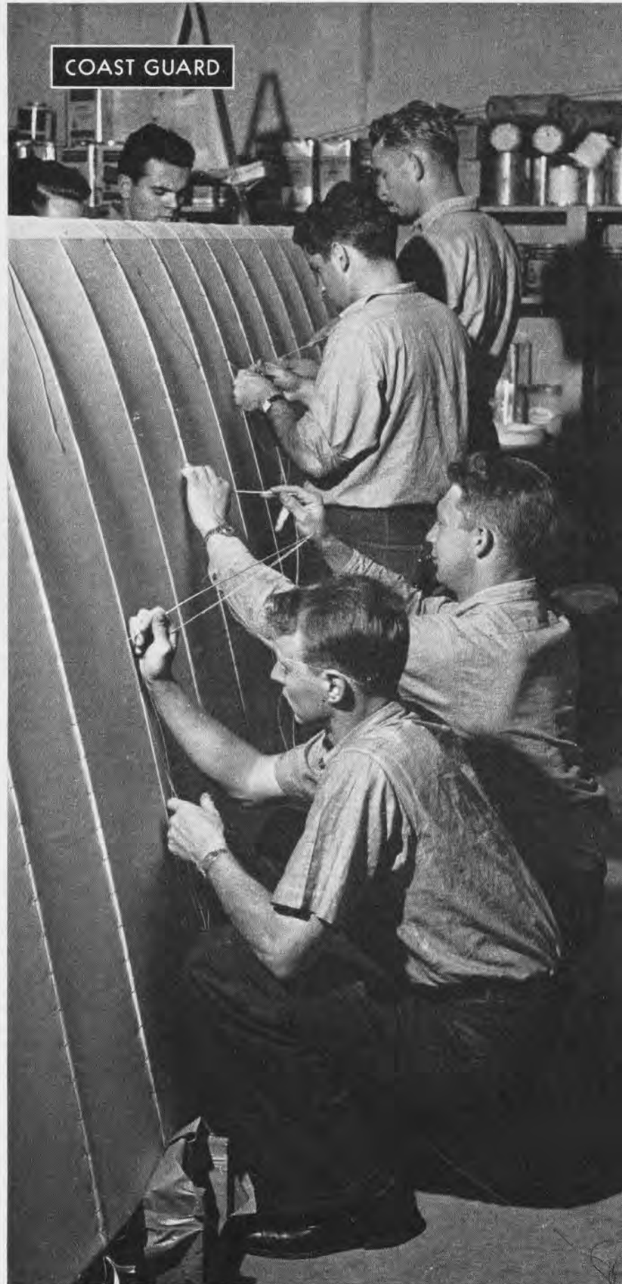
RIBSTITCHING MERCERIZED COTTON COVER TO STABILIZER FRAME DEMANDS PROFESSIONAL KNACK
