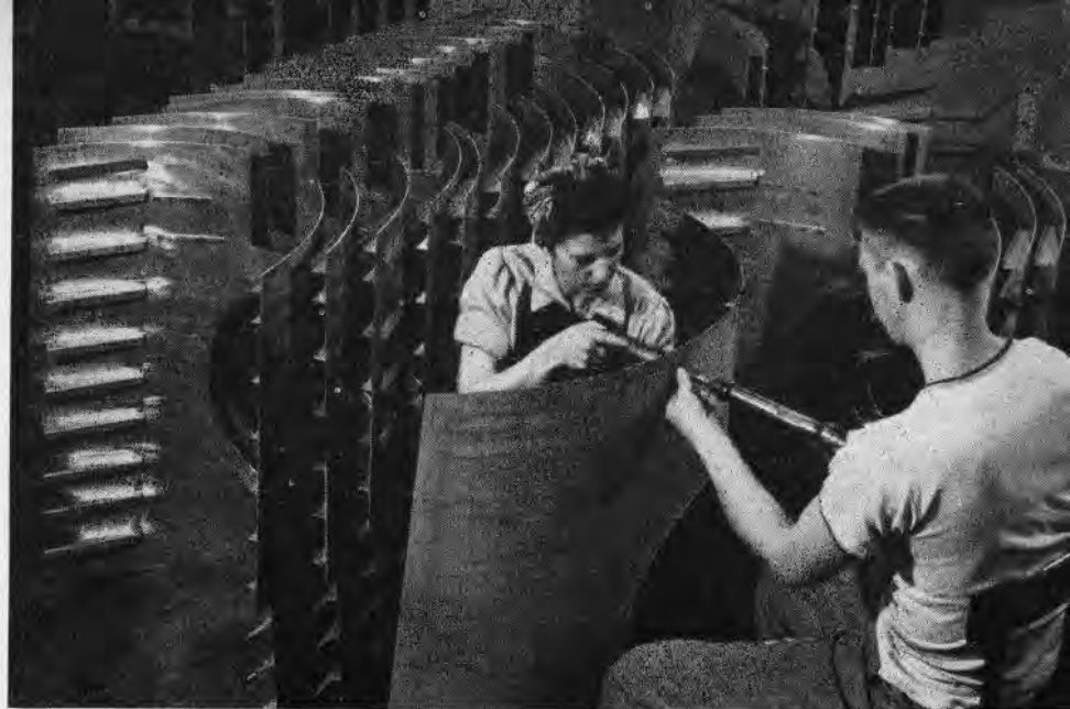
CLIQUE FASTENERS THAT TEMPORARILY HOLD RIB STIFFENERS ARE BEING REPLACED BY RIVETS
