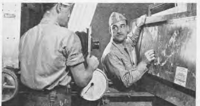
Quonset hut is erected to house precision copying cameras which are used to make aerial mosaic maps of Jap islands; Army, Navy and Marine units all use maps to lay out attacks
