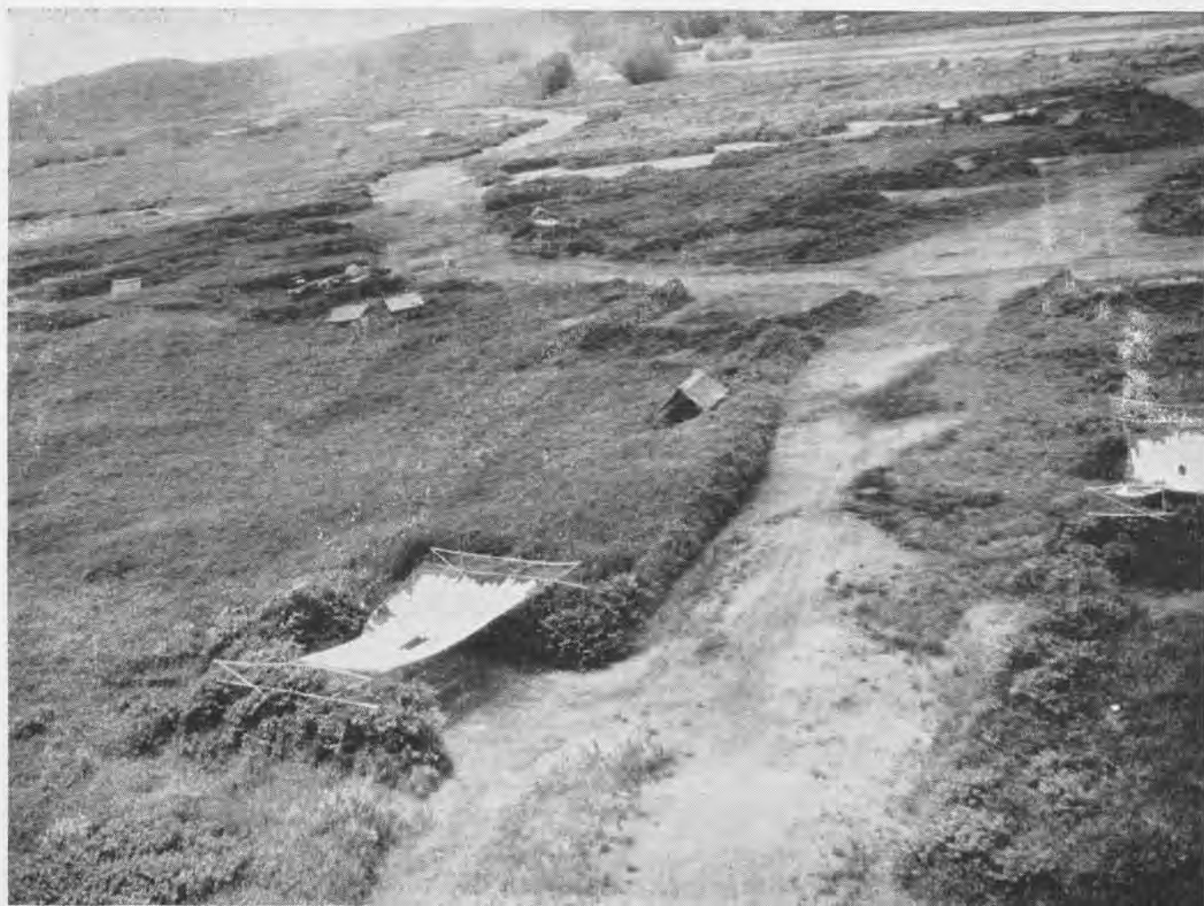
EFFECT OF NETTING INTERWOVEN WITH STRIPS OF CLOTH IS TO BREAK UP GEOMETRICAL OUTLINE, MAKING OBJECT LESS CONSPICUOUS FROM AIR
