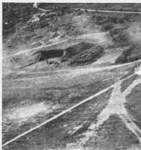
Grass sod covering plane revetment helps to blend it with immediate surroundings
